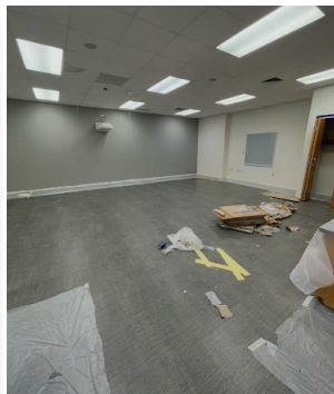
Rowe Lane Elementary Classroom Progress
