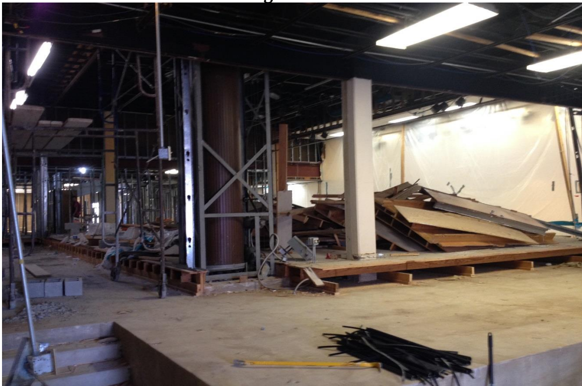
M.S. Stage/Cafeteria Remodel
