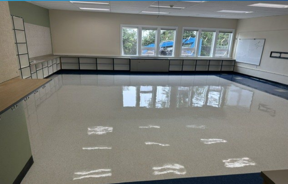
Yaquina View Elementary new tile floors
