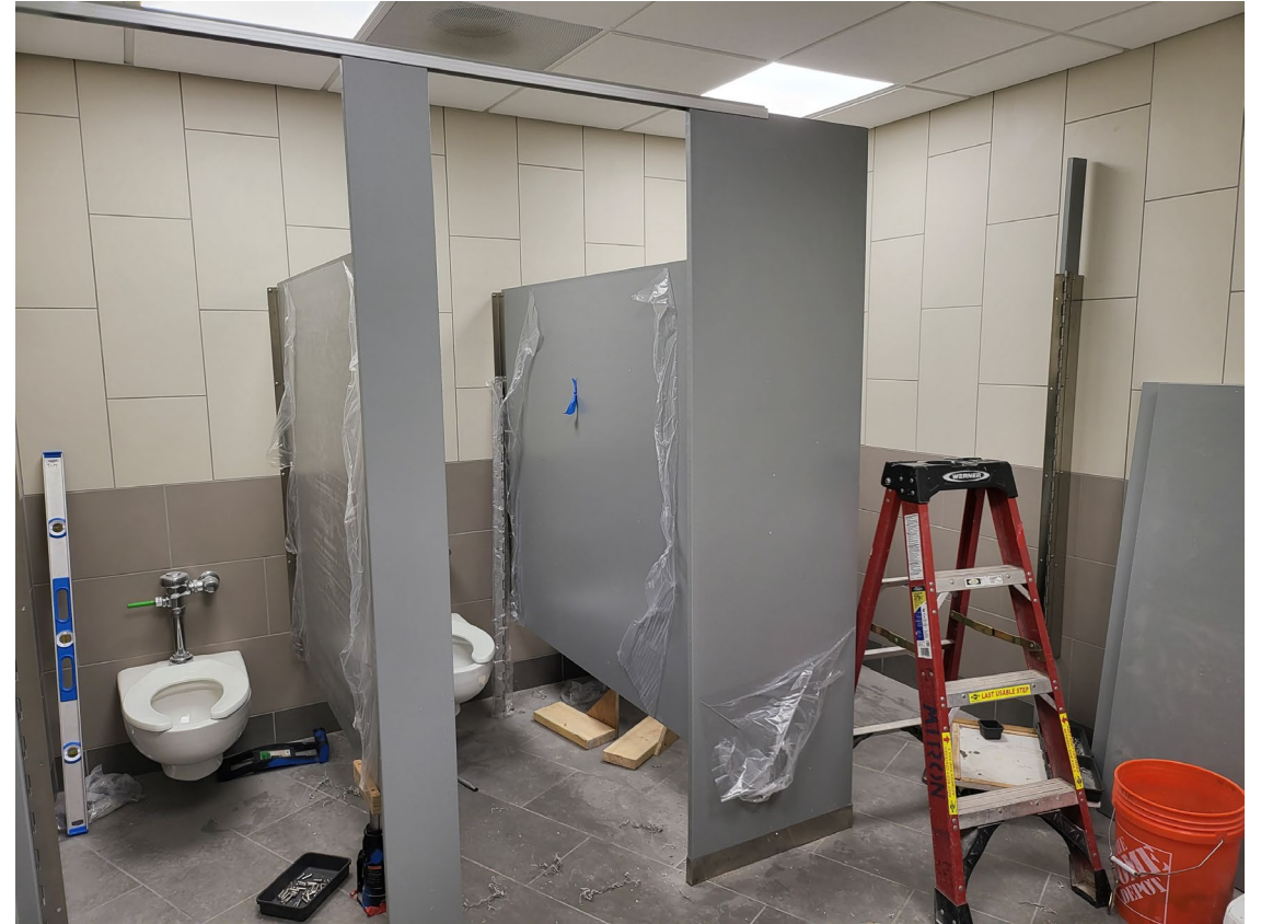
Renovated restrooms nearing completion
