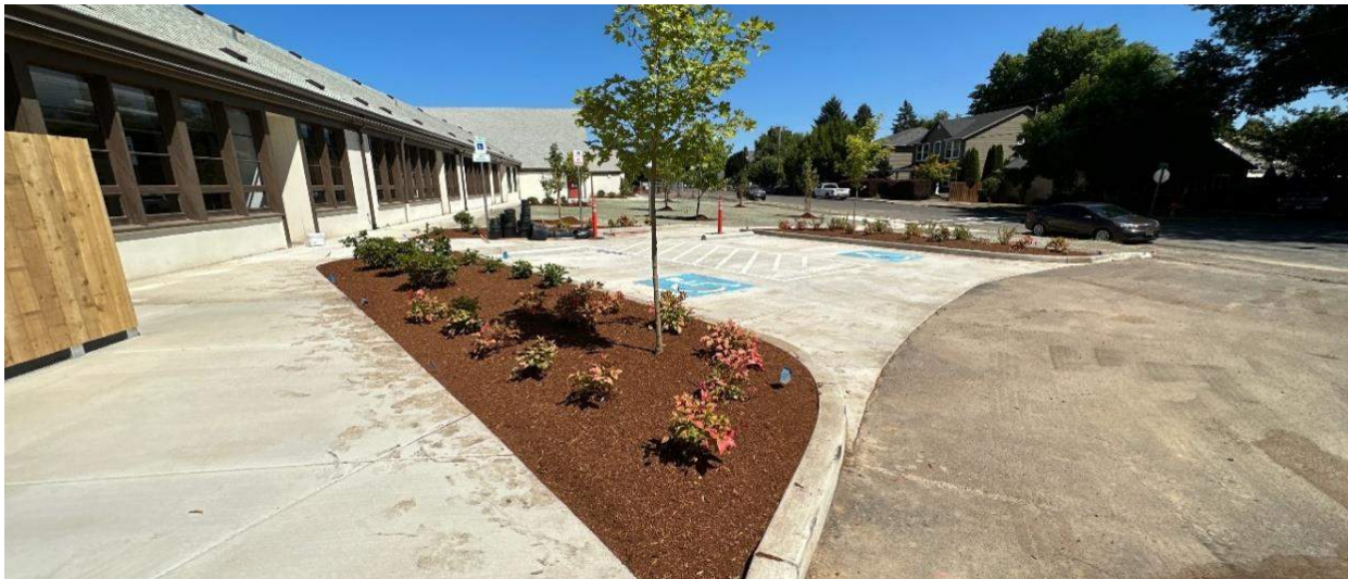
CHHS –New ADA parking at old entrance loop
