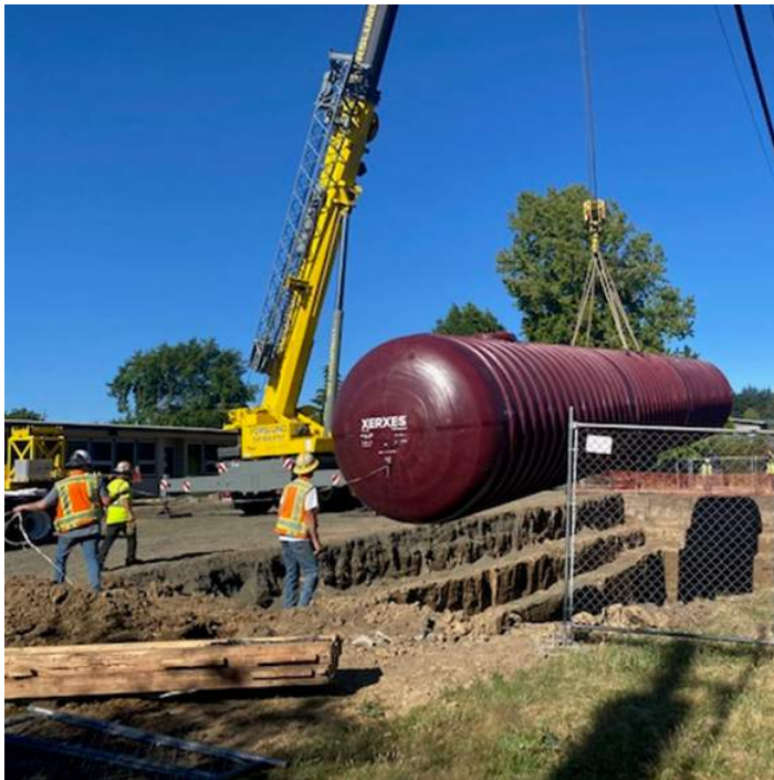
Fire Detention tank installed
