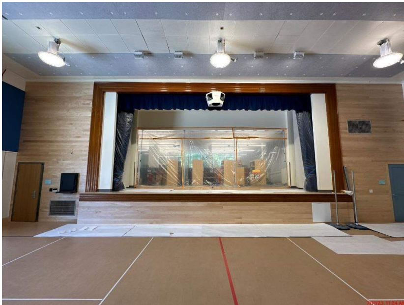
Franklin - New curtain and operable wall installed
