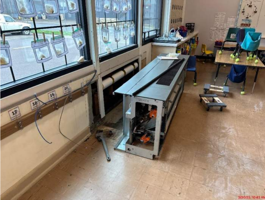
Franklin – Unit ventilator swap out
