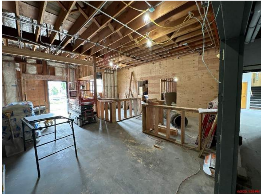
CHHS – Front office walls taking shape
