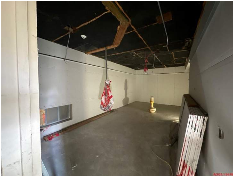
CHHS – New weight room area taking shape (old girls locker/shower room)
