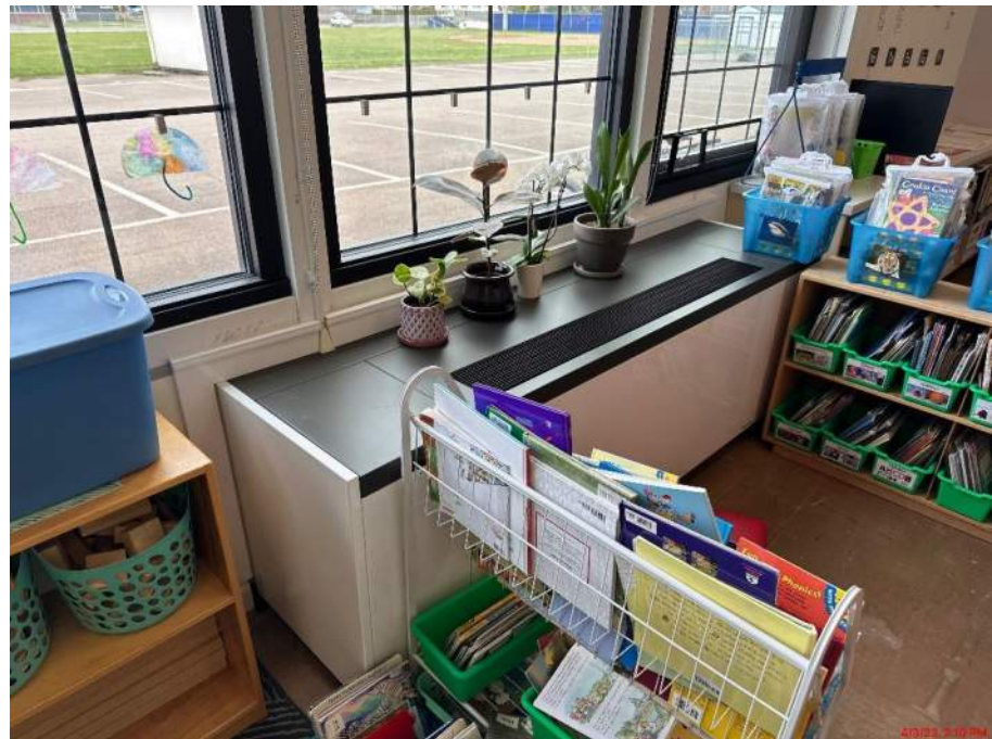
Franklin – New unit ventilator in place
