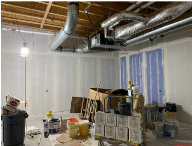
Staff Work Room
