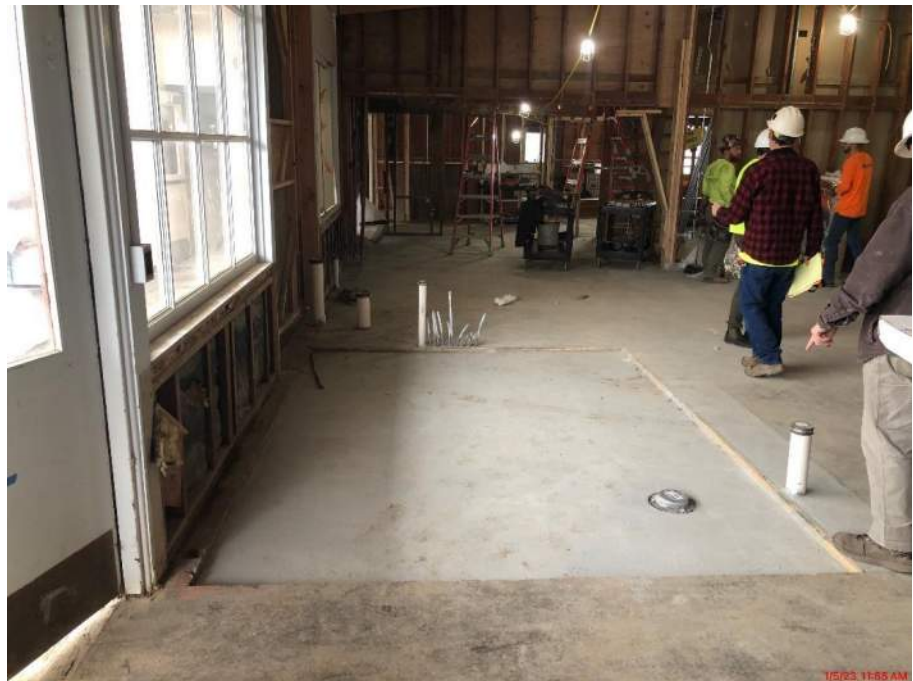
CHHS - New bathroom slab in place
