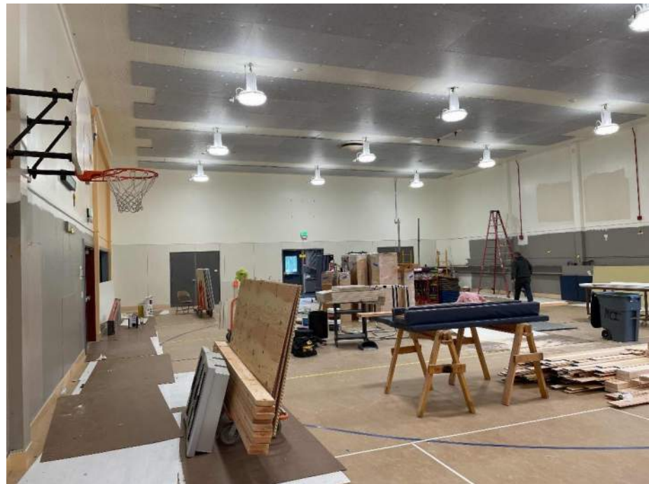
Franklin Gym – Wall paint, FRL wainscot, wood base install
