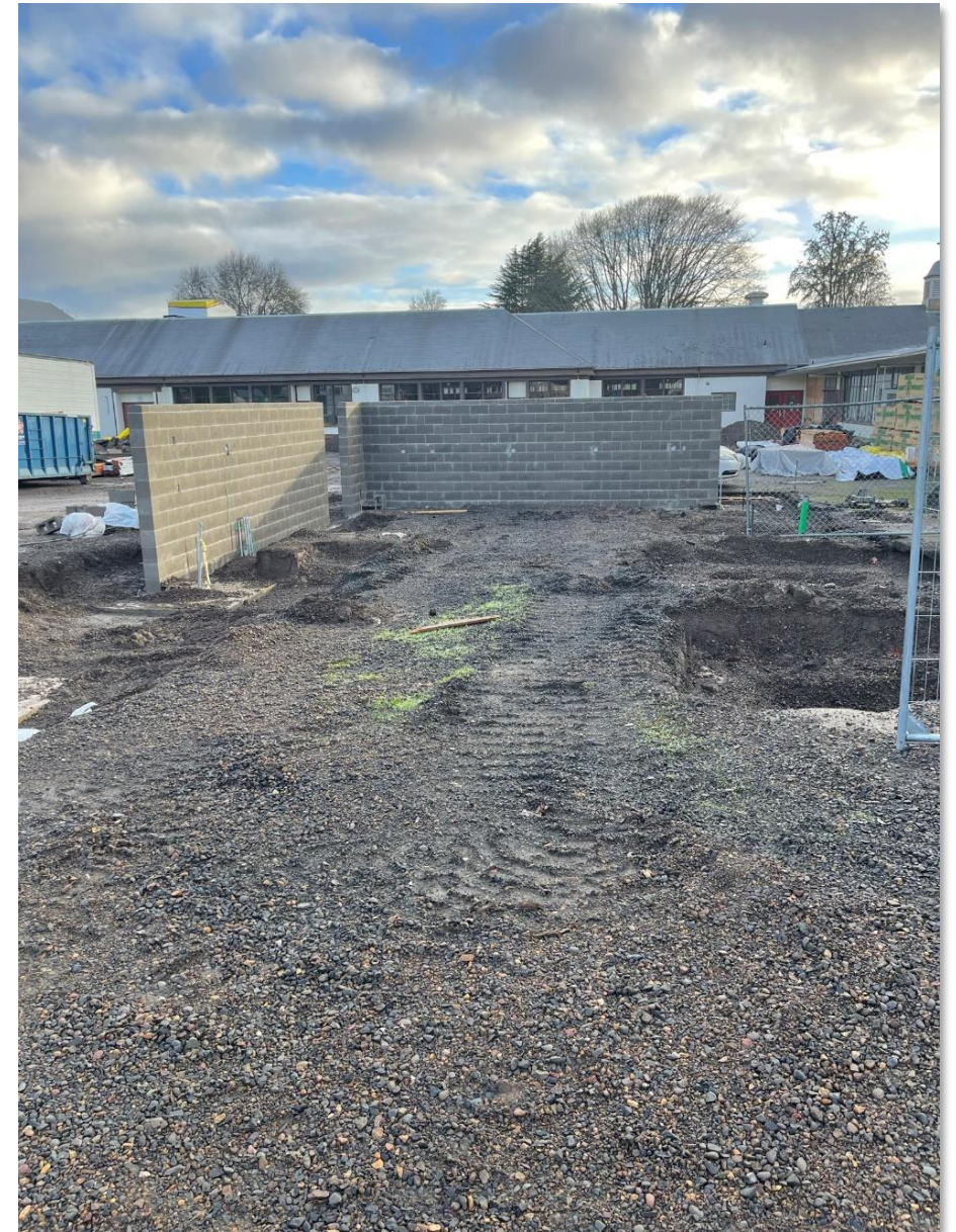
Covered Outdoor Learning progress
