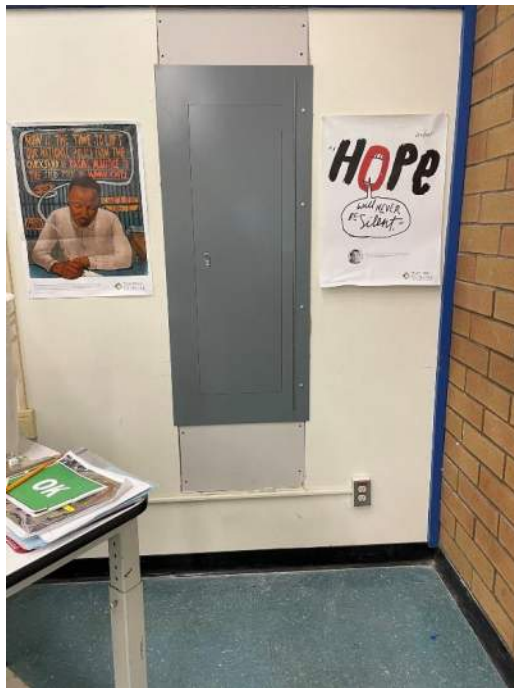
CMS – Elec panel after new panel is installed
