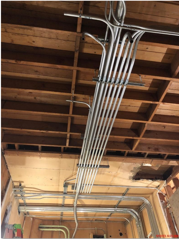
New electrical conduit - bringing the building up to code
