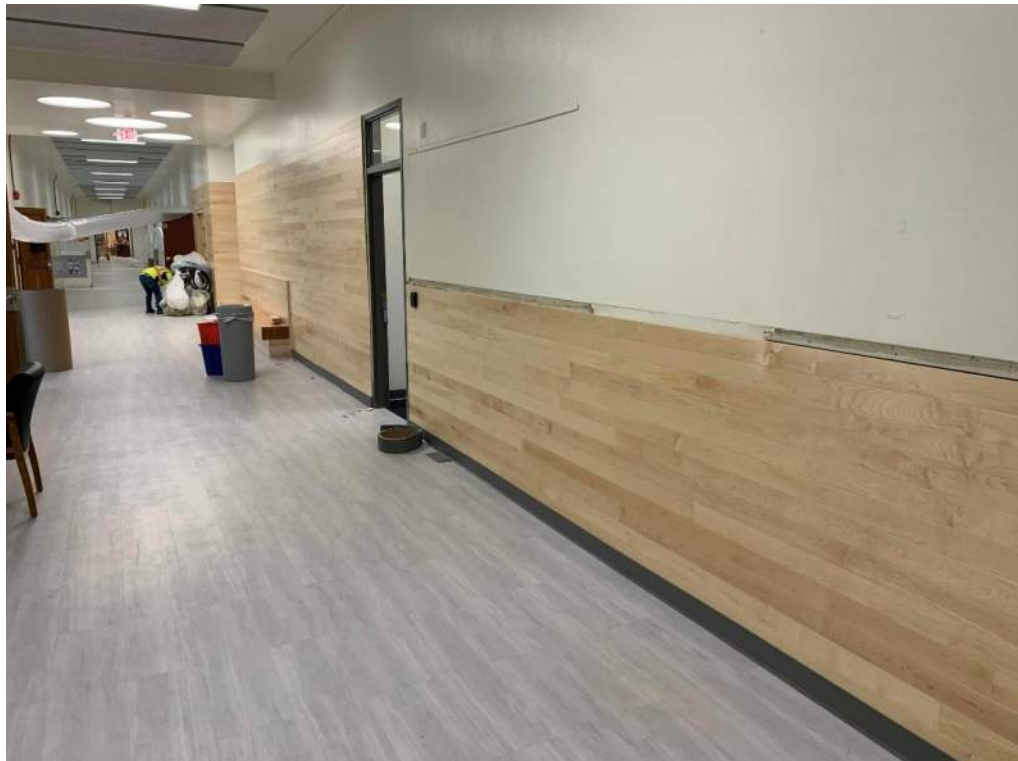
Franklin – new wood-1 wainscot in main hallway.
