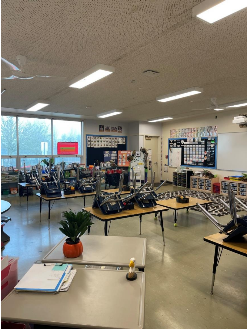
Classrooms now have new LED lights and ceiling fans
