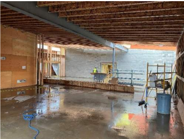
New Addition – Cafeteria
