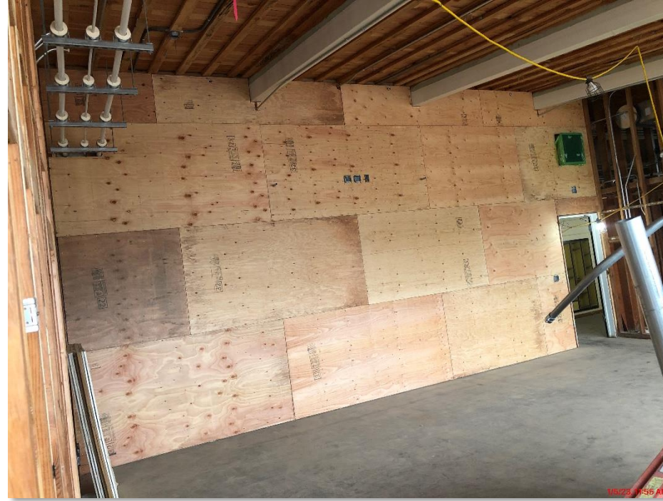
Shear Wall and other framing going up!
