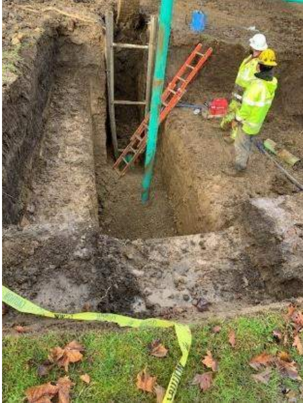
CHHS -New sewer connection to City services stub
