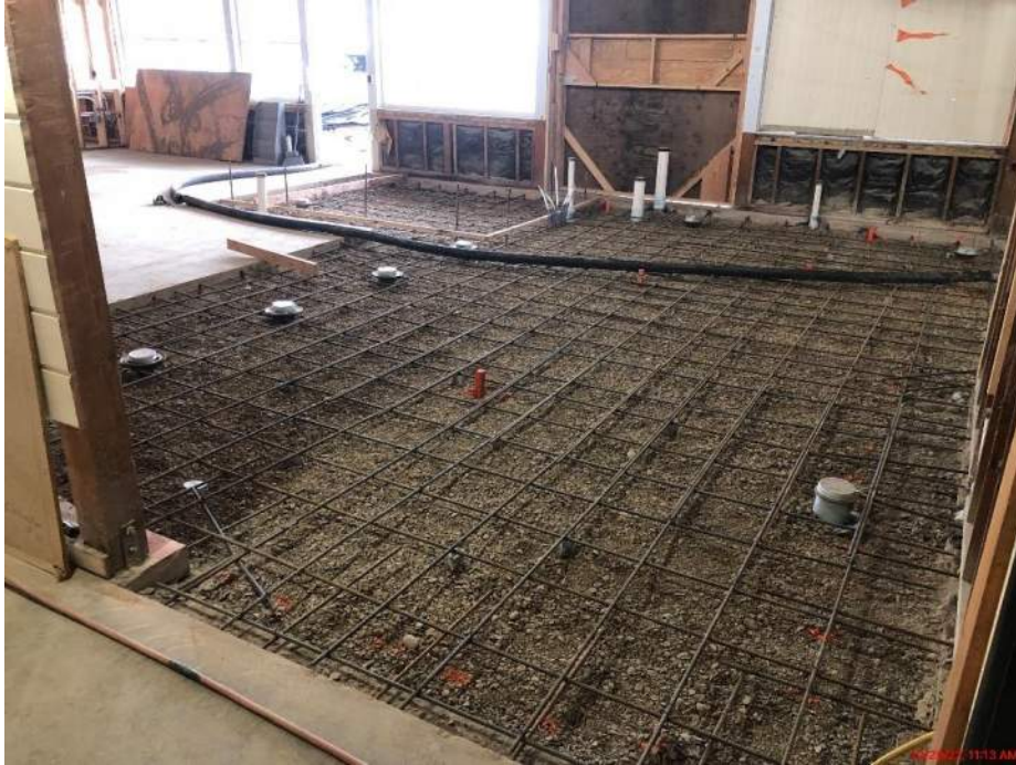
CHHS -New bathroom area slab prepped
