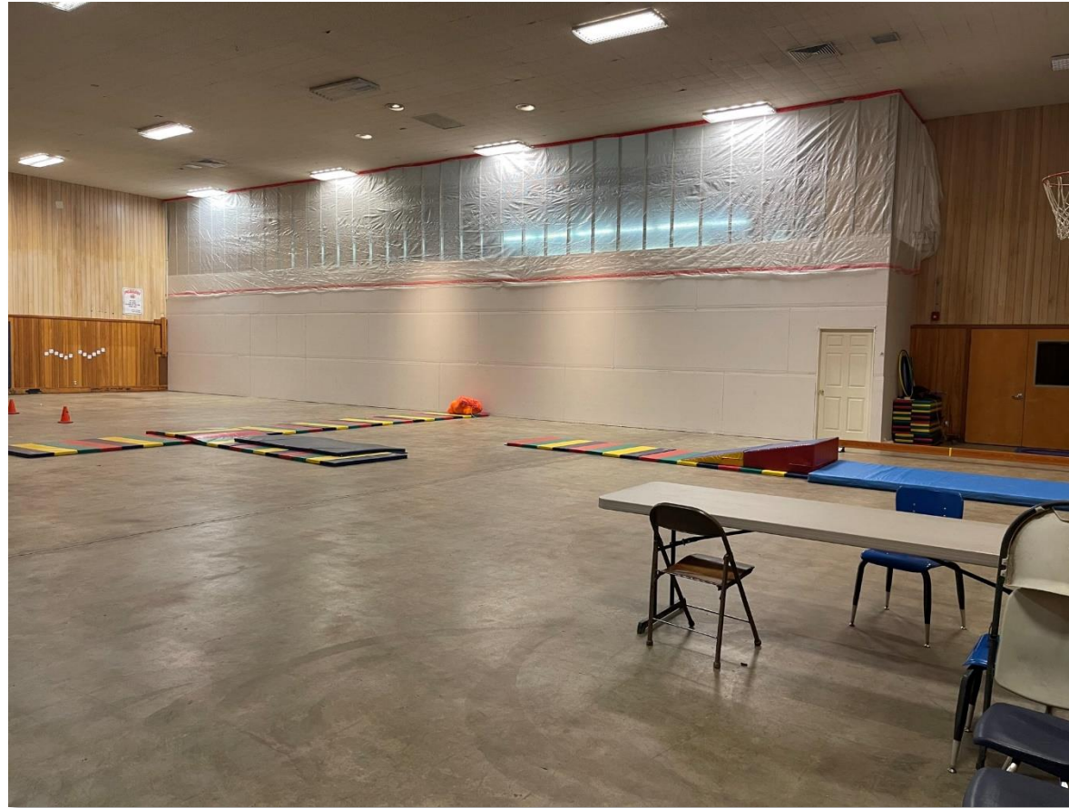
New Music Room framing (left) as seen from Gym (above)
