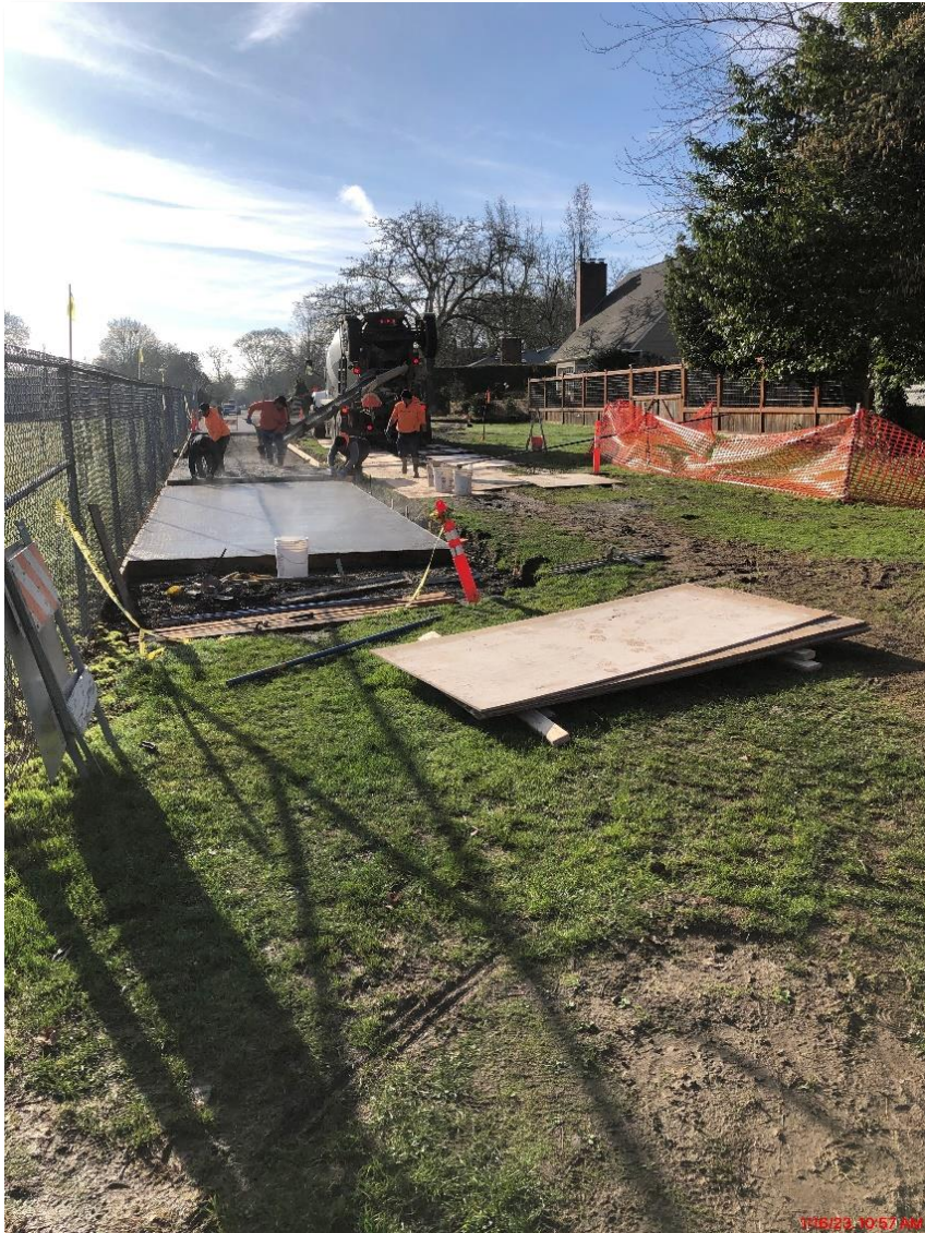
Work on the sidewalk along 33 rd St. continues
