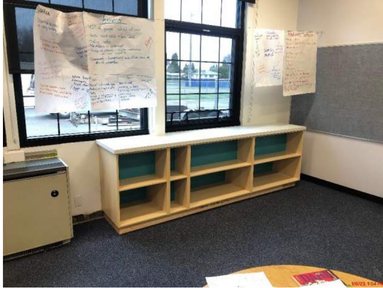
Elementary wing – new operable windows & new casework at unit ventilators
