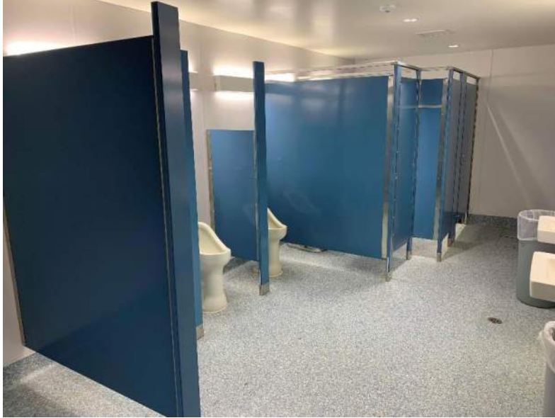
New toilet partitions in remodeled restroom areas
