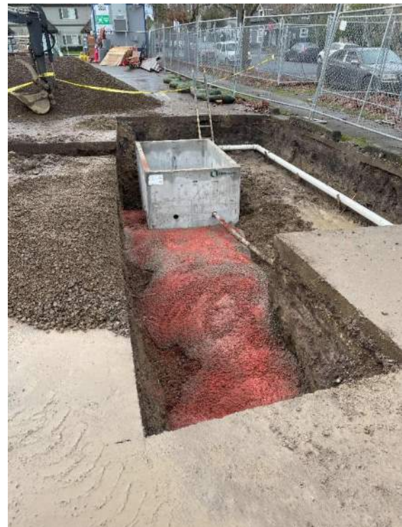
Franklin – New transformer underground and vault set
