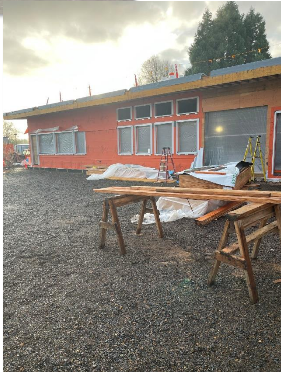
New Addition framing continues
