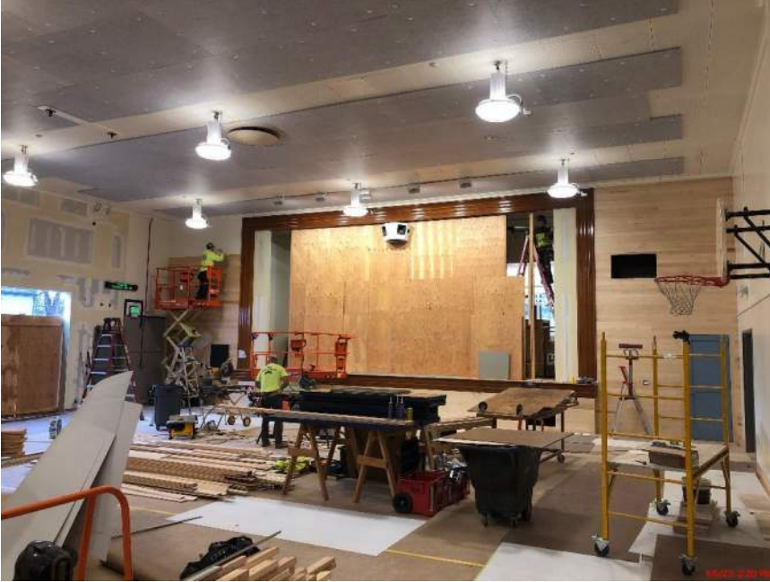
Franklin Gym – OH Door opening & Wood-1 wainscot over winter break
