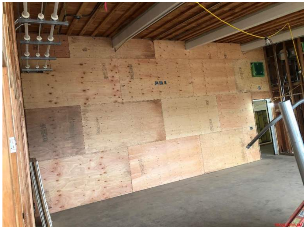
CHHS- mock up wall now a shear wall
