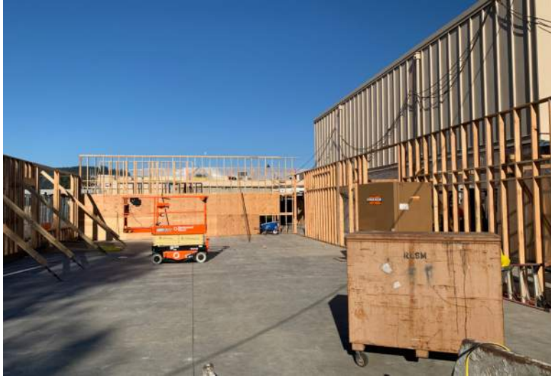
Art / Science Wing wall framing
