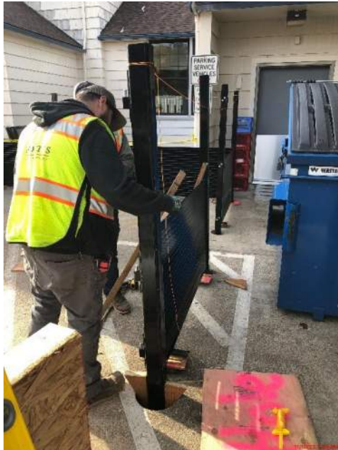
Trash enclosure in progress
