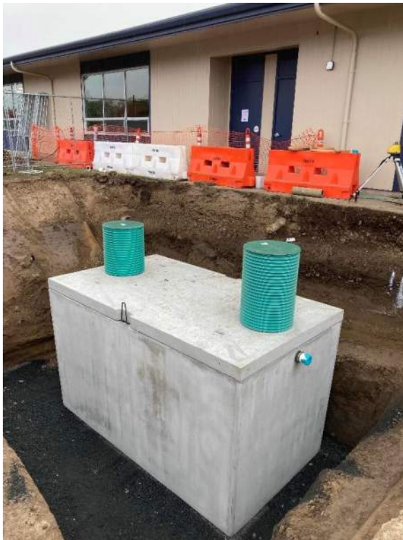
Installation of new septic tank
