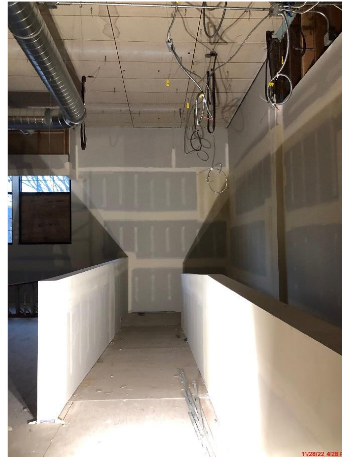
Library Ramp Wall Progress
