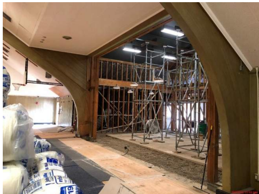
CHHS- Gym-Reception wall opened up for reframing & storefront
