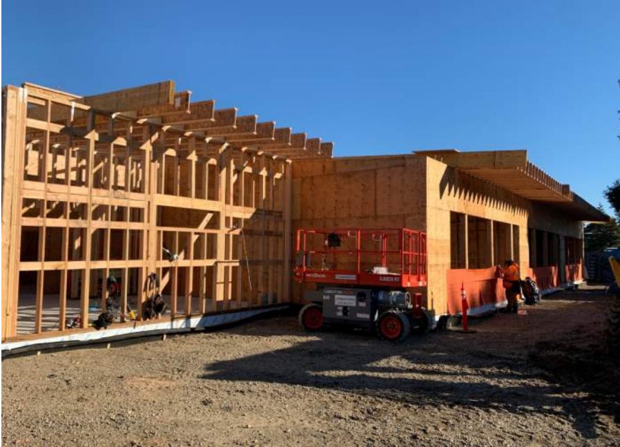
New Classroom Wing Framing
