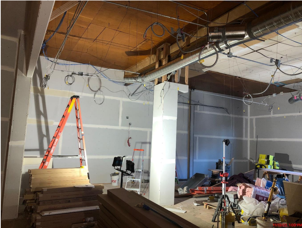
Library Finishes are Underway
