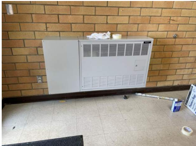
CMS – Cabinet Unit Heater Installation
