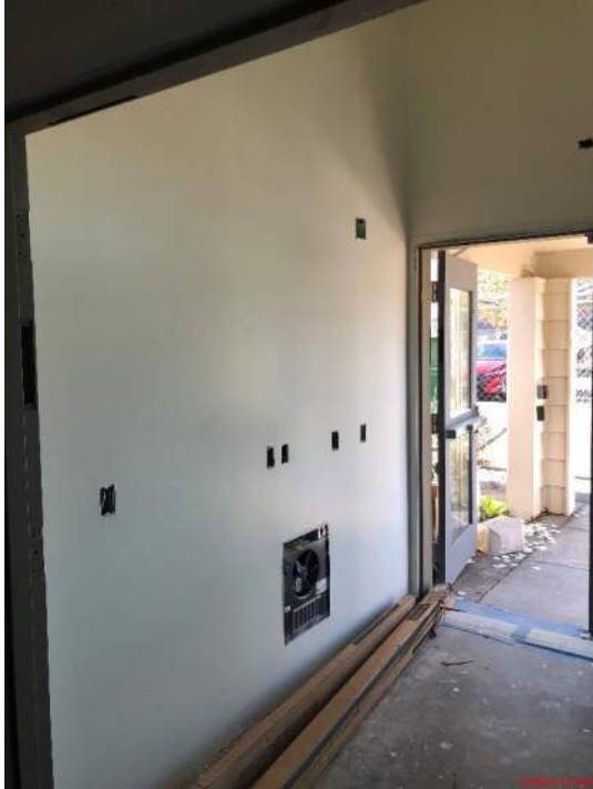
New Admin – finishes progress at entry
