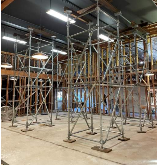
CHHS – temp shoring for reframing efforts
