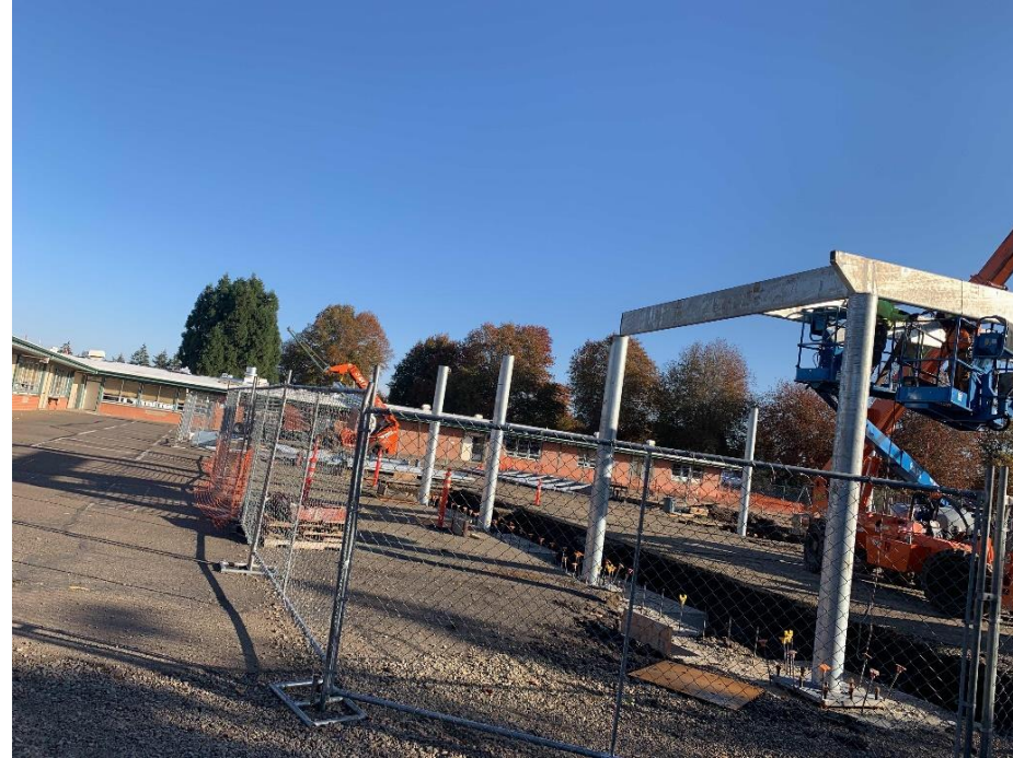
Covered Play Under Construction
