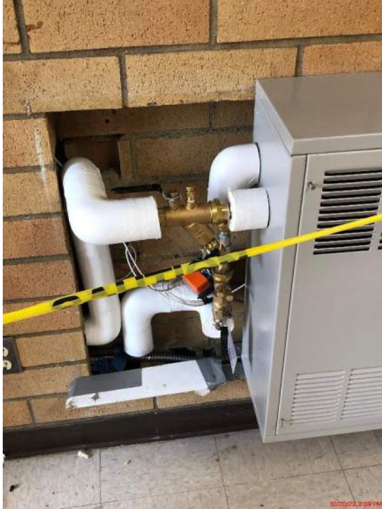
CMS – Cabinet Unit Heater Installation
