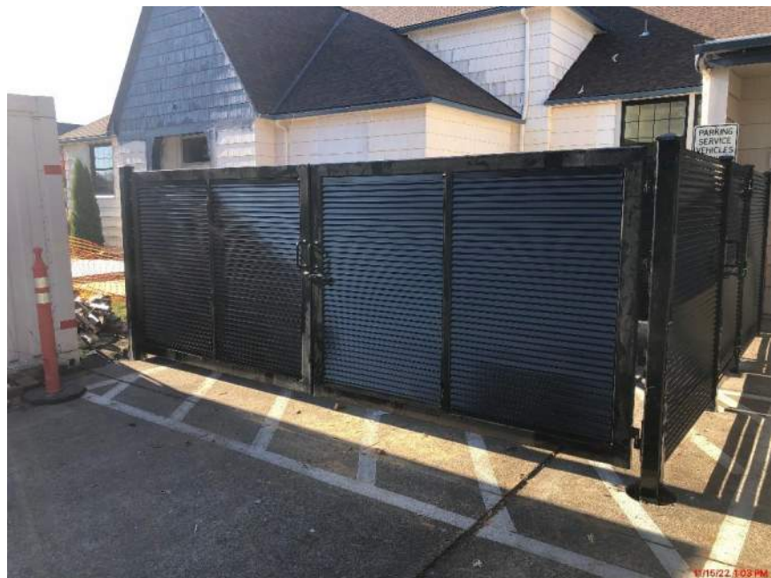
Trash enclosure finished
