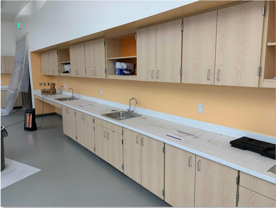
Science Classroom Progress
