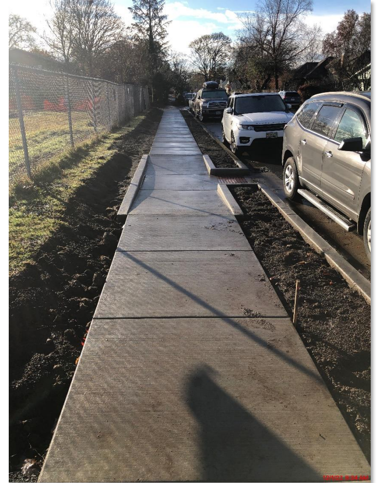
Site improvements along 33 rd Street
