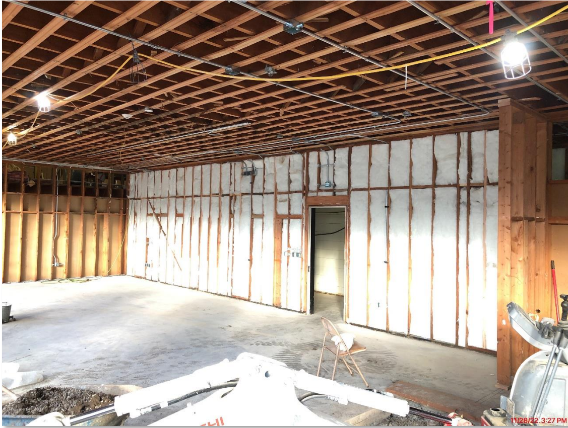
Sound Insulation Installed on Classroom Corridor Wall
