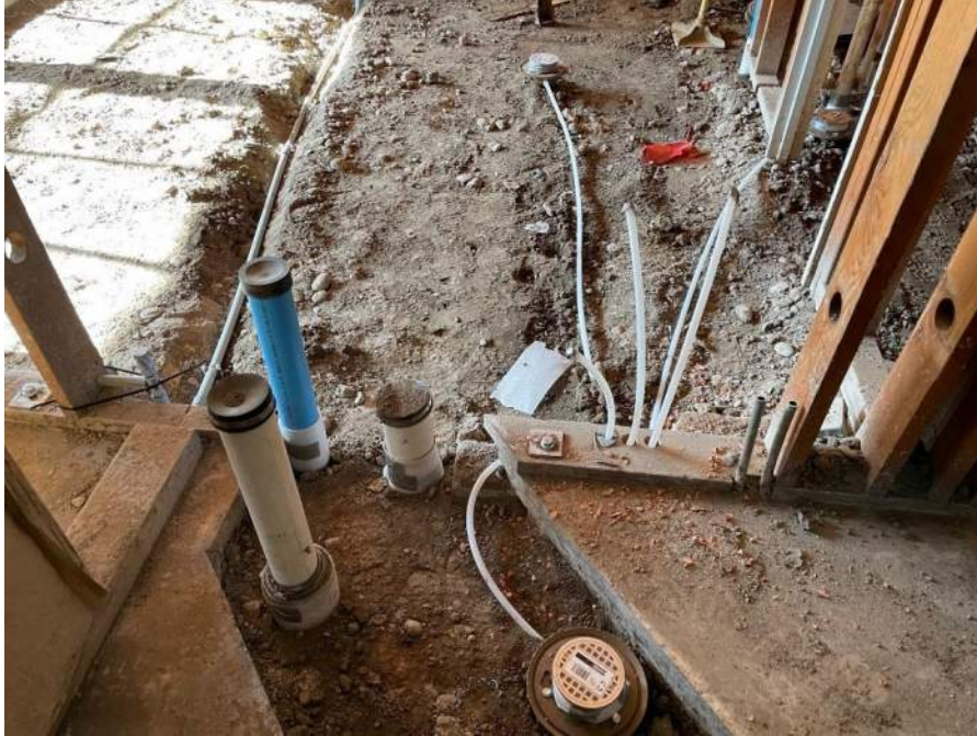
CHHS – Science plumbing underground progress
