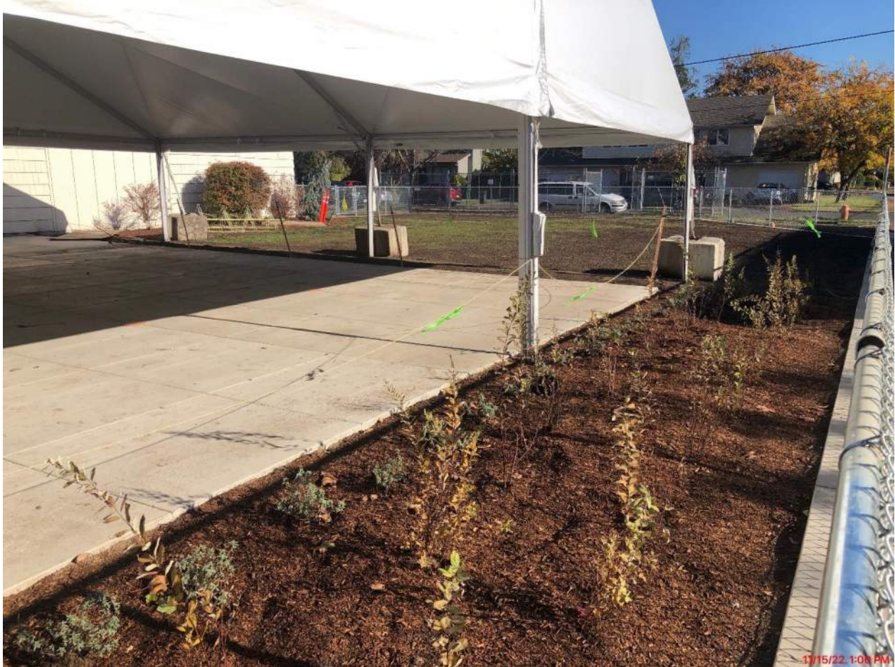
New Outdoor Patio landscaping & fencing
