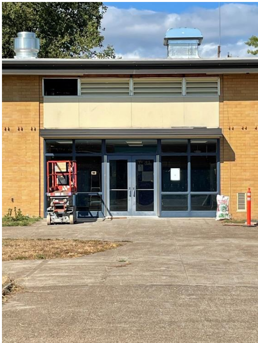
CMS – Louver Installation
