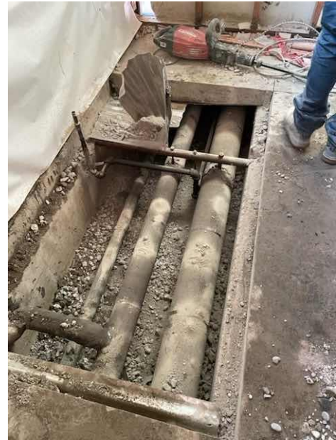
New Admin - Steam Tunnels Exposed for Piping Work
