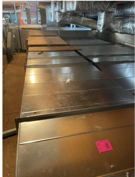
CMS – New Larger Ductwork Sections
