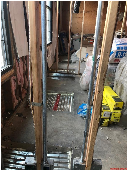
New Admin Tunnels Prepped for Slab Pourback
