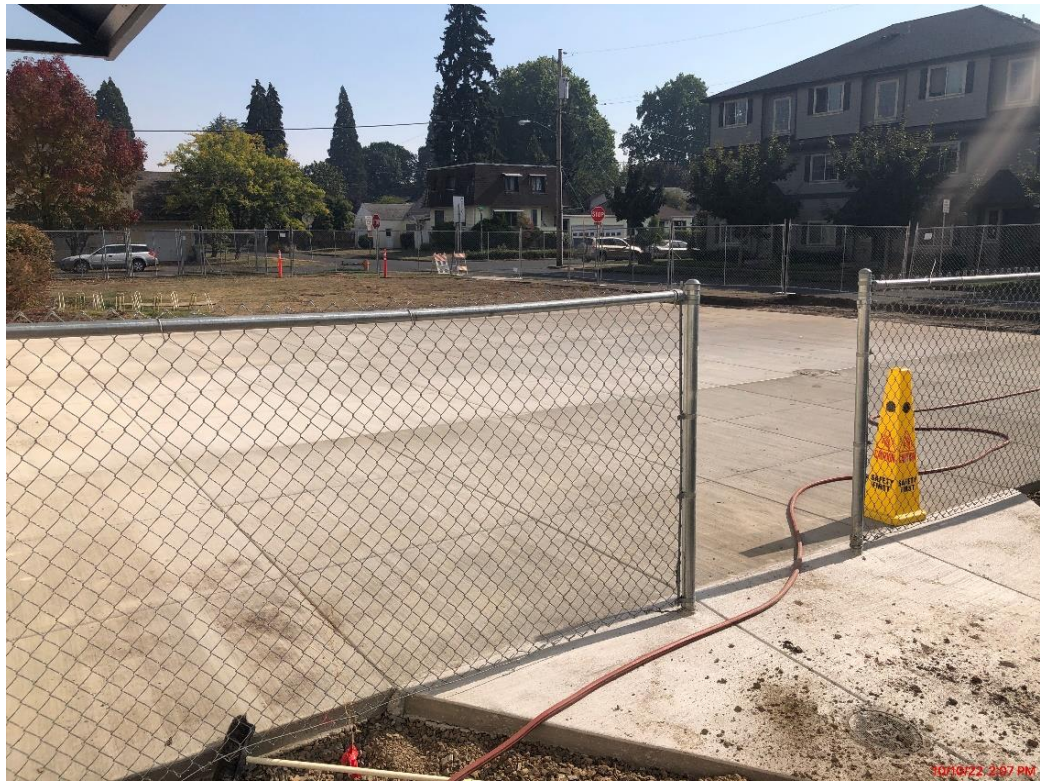
New Outdoor Patio Placed and Ready for Tent & Fencing
