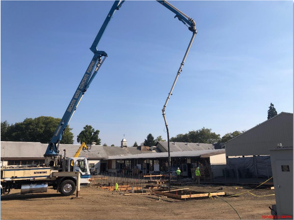
Pouring Footings for New Outdoor Classroom
