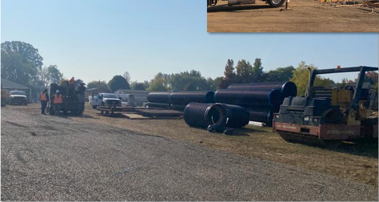
Storm Piping Staged
