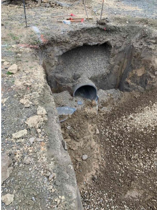
Abandoned 20" Waterline – Cut & Capped
