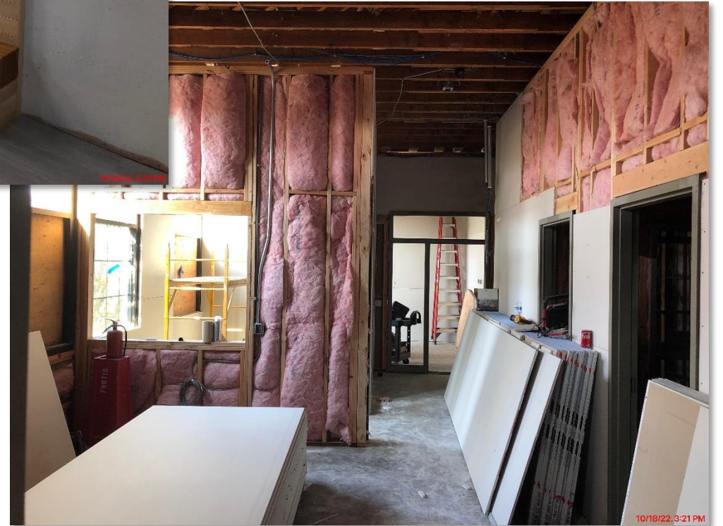
New Admin Space Progress
