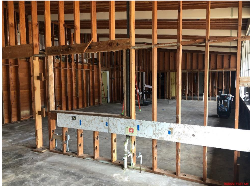
Area B Classroom Wall Demo
