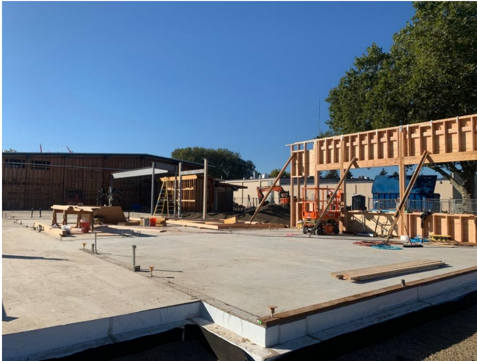
First Wall of the New Addition is in Place
