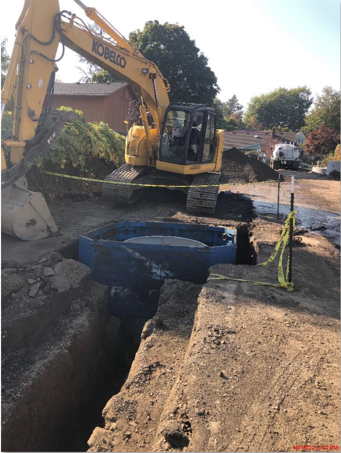
New On-Site Storm Manhole
