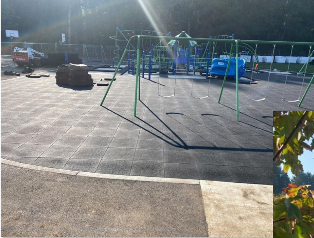
Playground Tile Installation Almost Done
