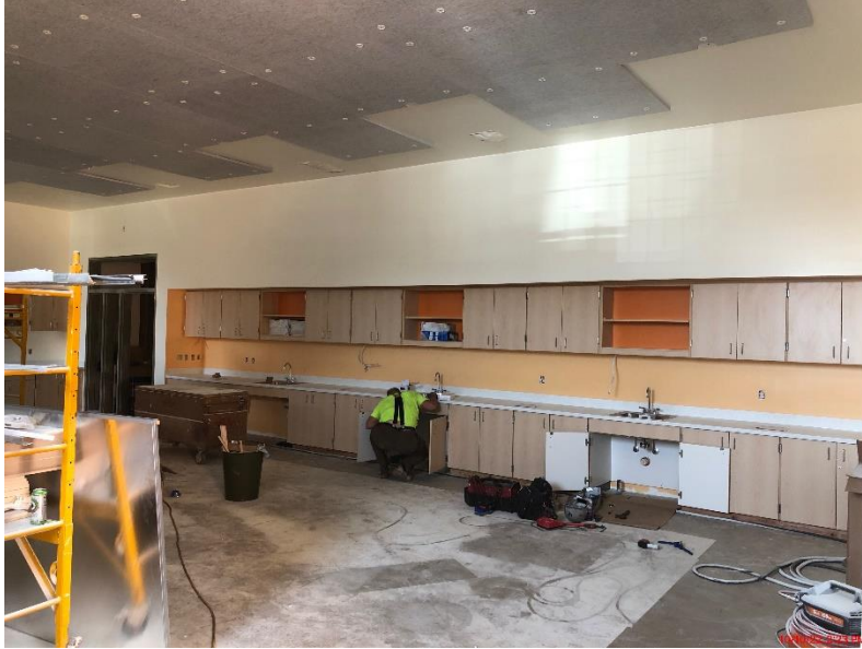
Science Casework, Acoustical Ceiling Panels and Finish Painting Almost Done
