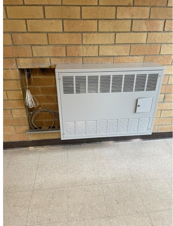
CMS – Cabinet Unit Heater Installation
