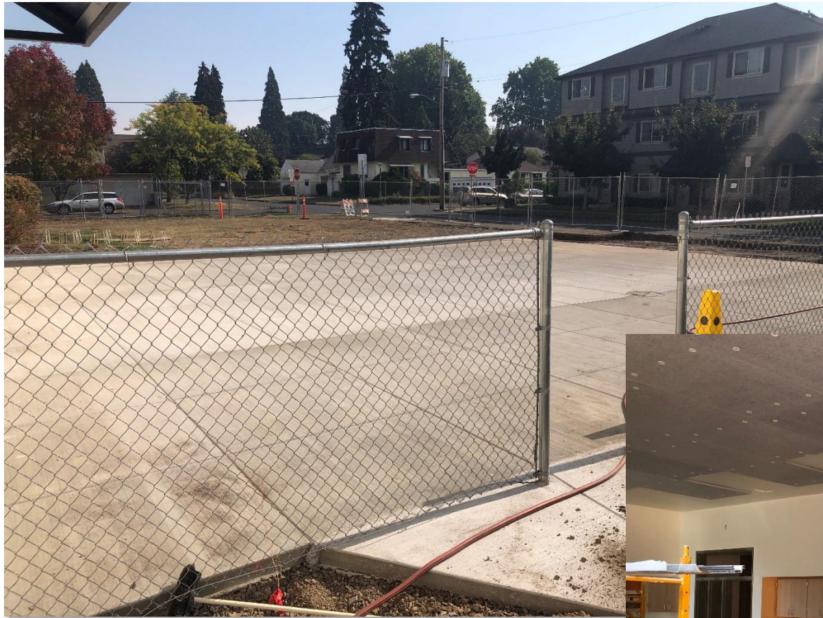
New Patio Has Been Placed
