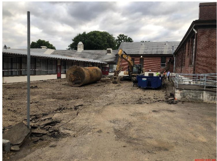
Fuel Tank Removed
