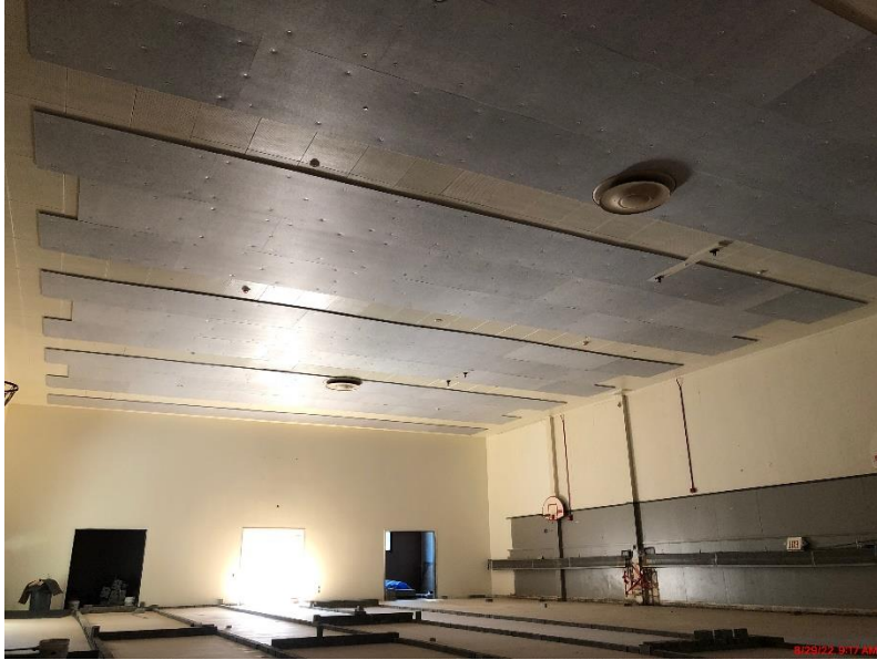
New Gym ceiling acoustical panels
