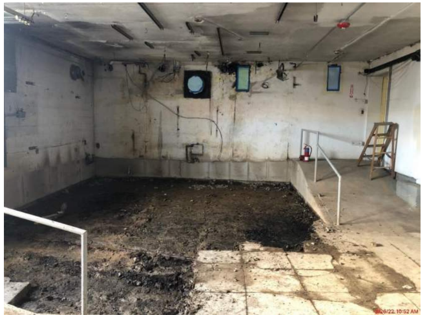
College Hill – Boiler Room Demo
