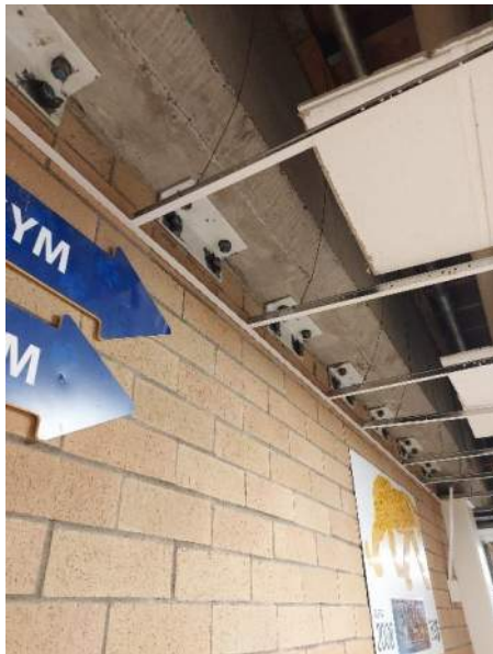
CMS – New seismic angles in gym corridor
