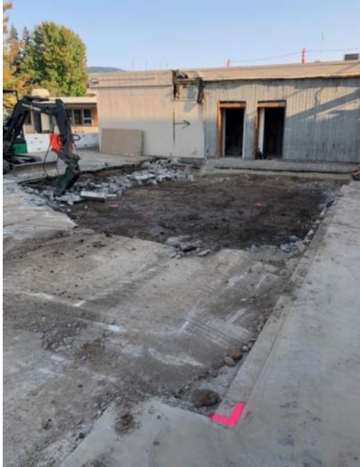
Demo of existing slab at old locker rooms
