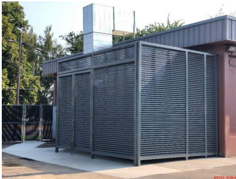
Dust Collector Screen Wall - current configuration
