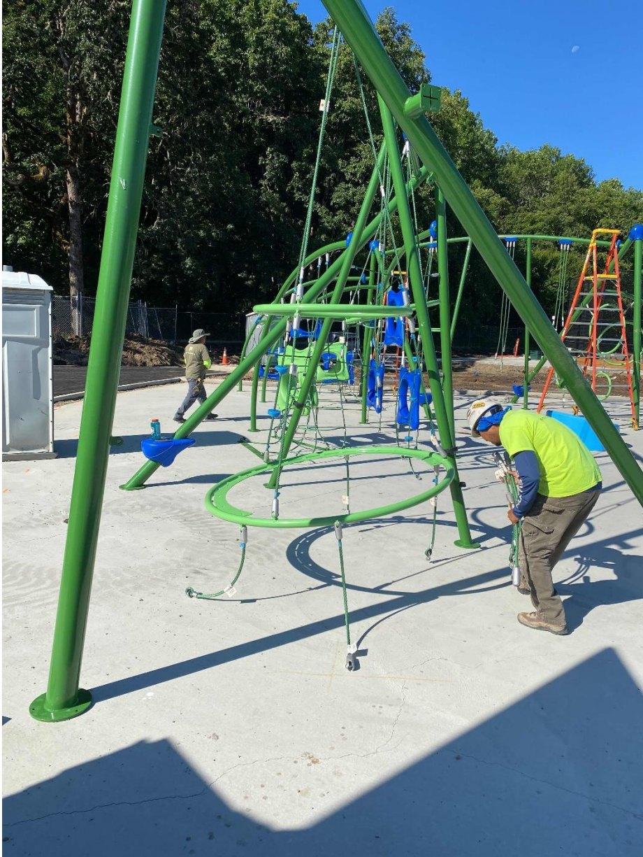
Playground Installed - Awaiting Play Tile Crews
