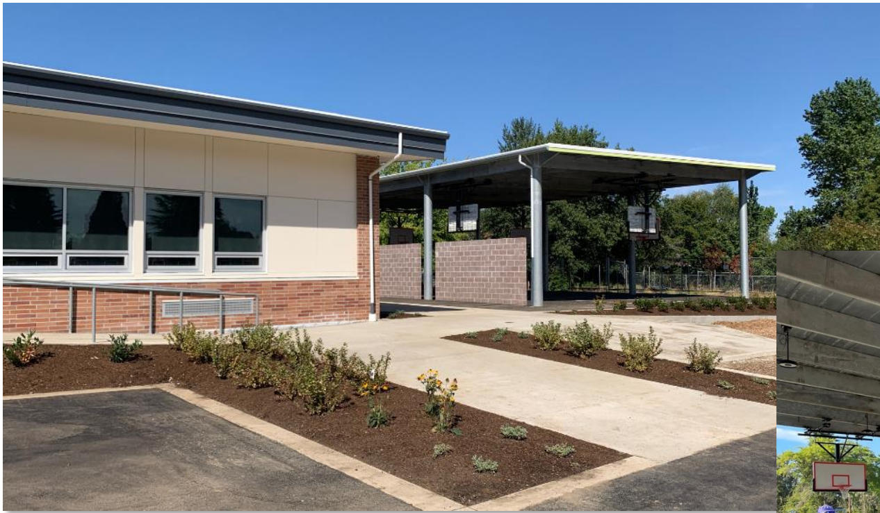
Play Structure and New Addition
