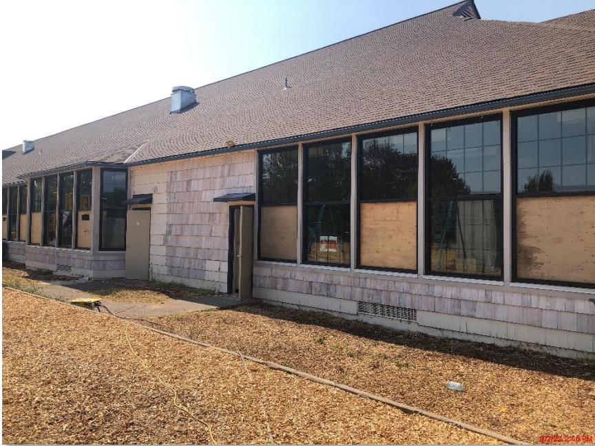
New Windows are in, Waiting for Opening Sections
