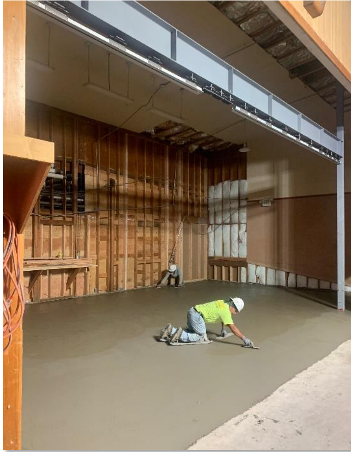
New Music Room Under Construction
