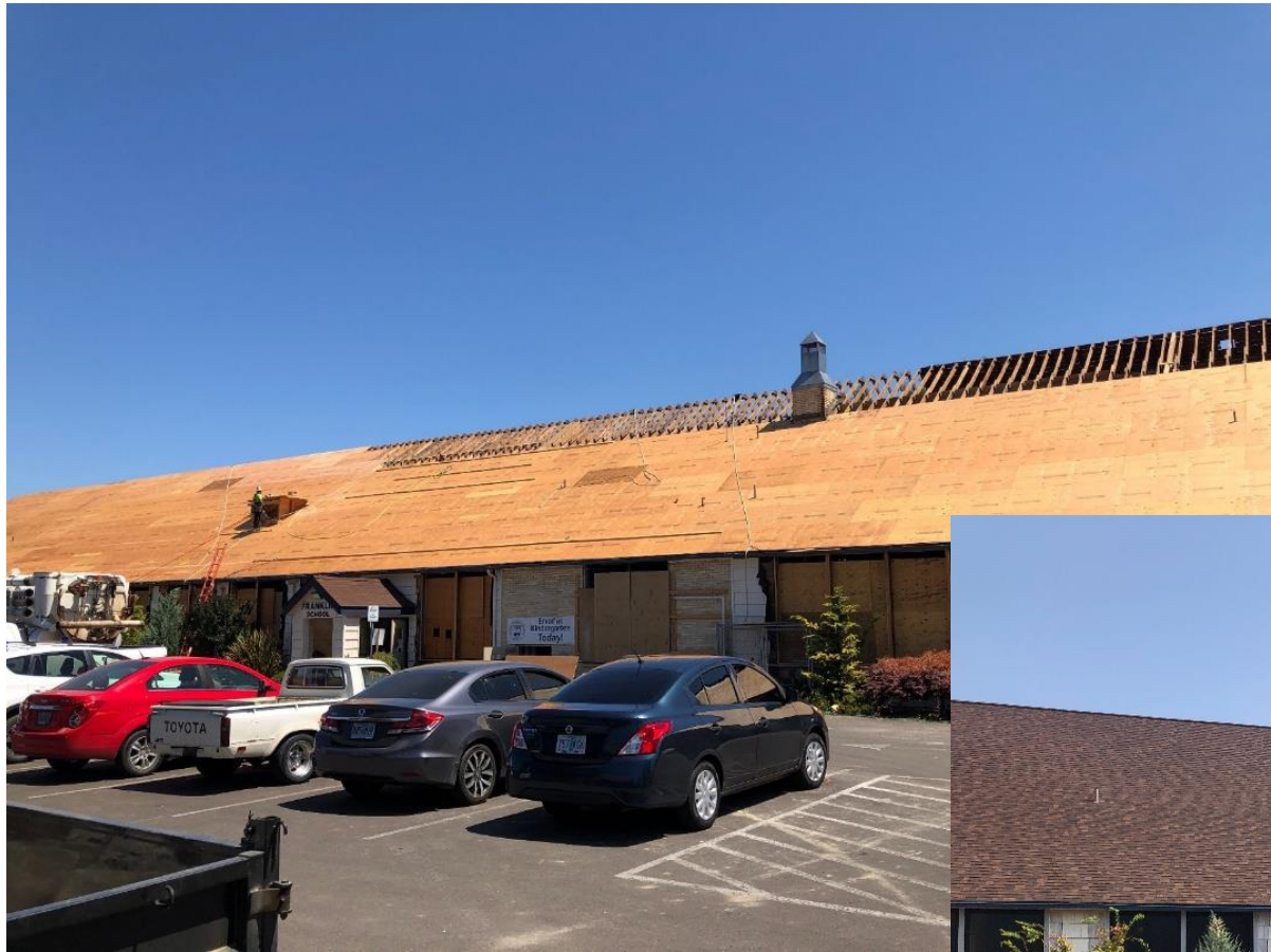
Roof Replacement - What a Difference a Month Makes!
