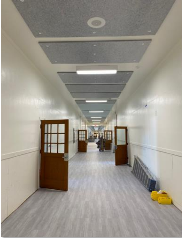
New Hallway Floors and Ceiling – Wainscots Yet to Come!
