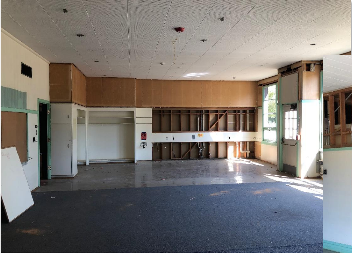
Demolition is underway!
