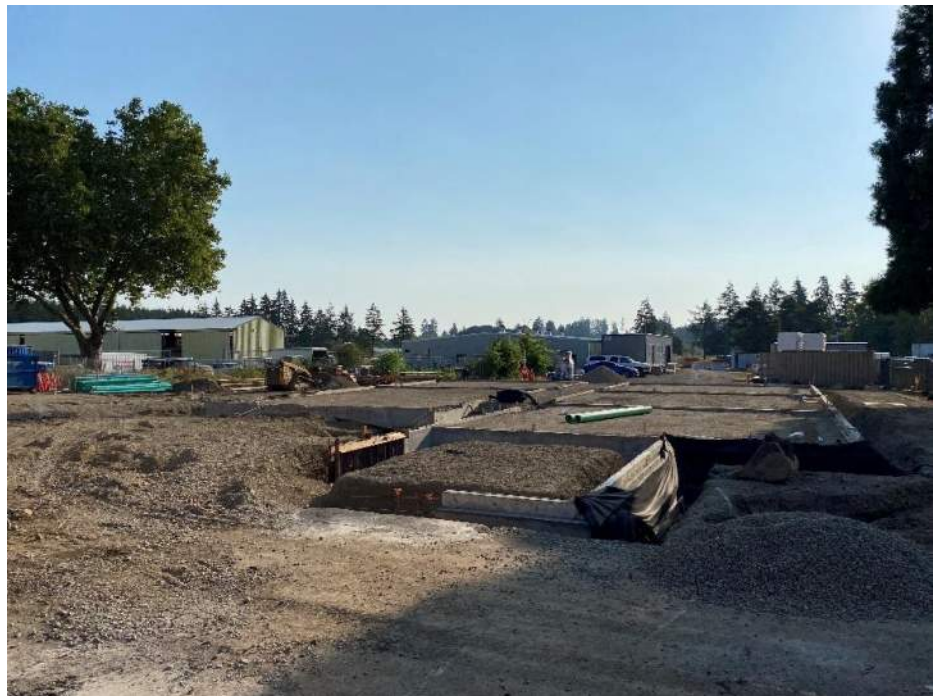
Addition ready for concrete slab
