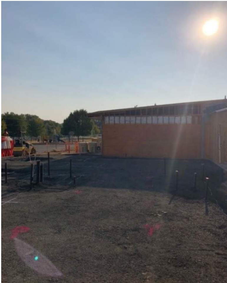
Admin Suite underground work
