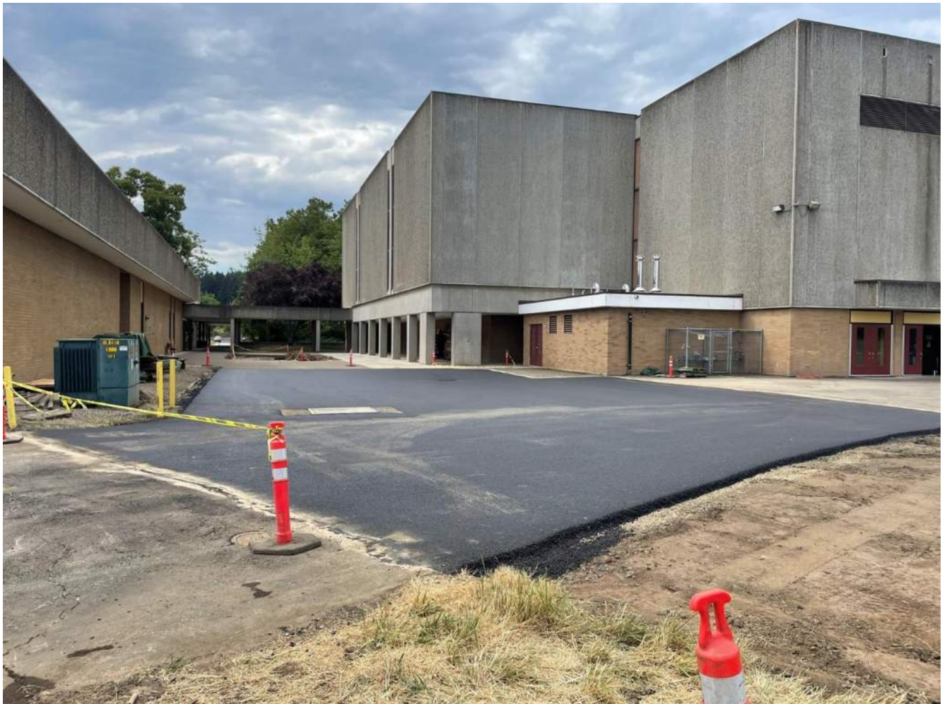
Bldg. A – B Replacement asphalt
