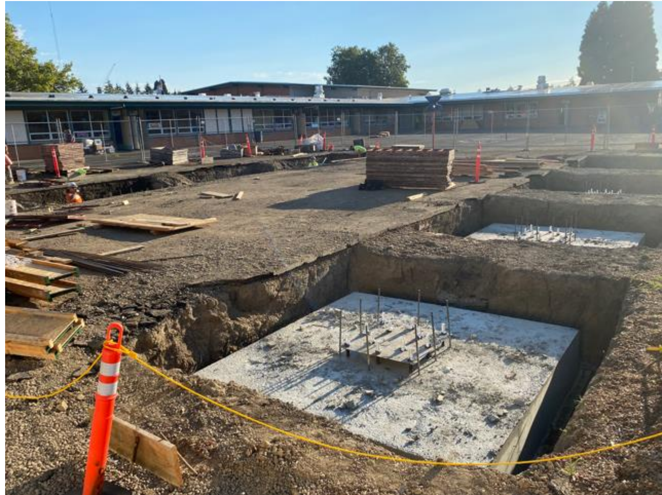
Concrete Footings for Covered Play Structure
