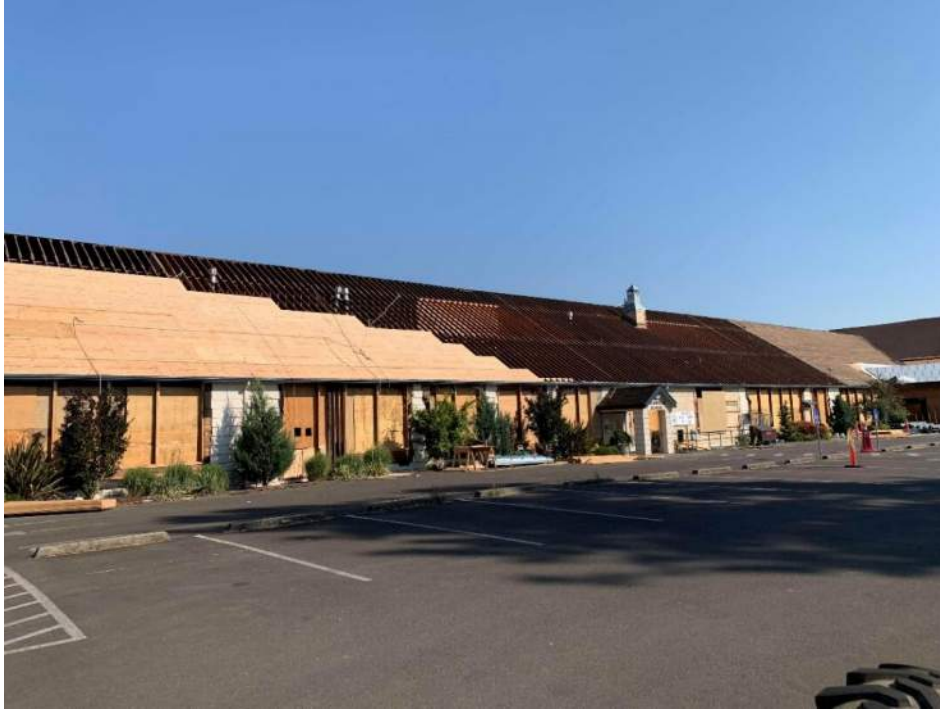
Existing roofing and roof deck demo and new plywood installation
