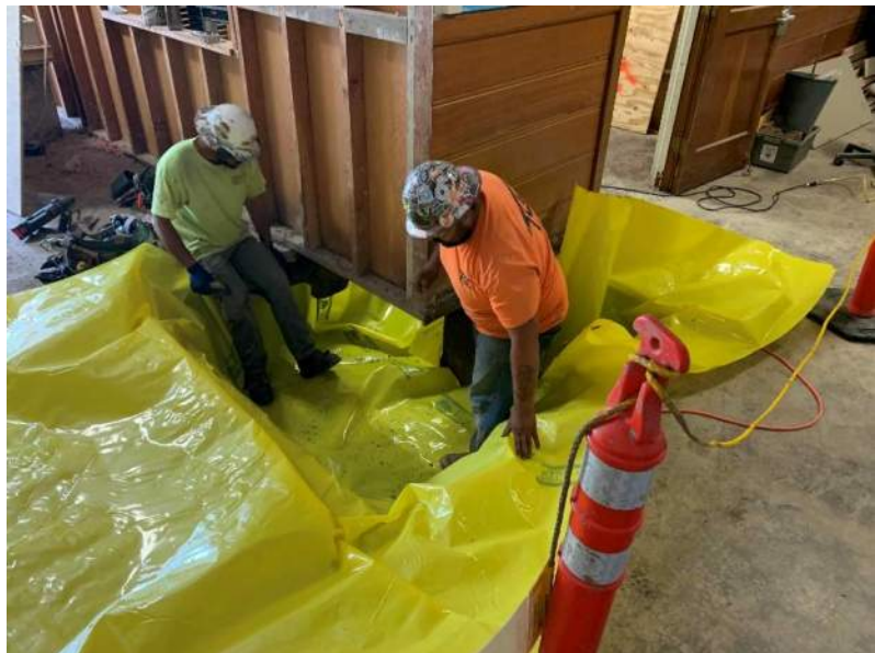
New interior footing work
