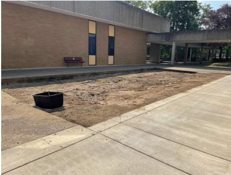
Progress toward restoring subgrade and landscaping between Bldg. A & B
