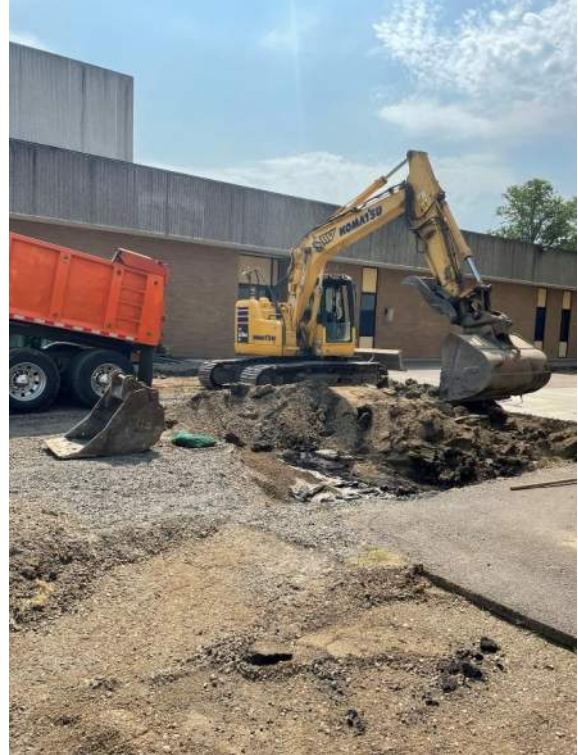
Cleanup between Bldg. A & B
