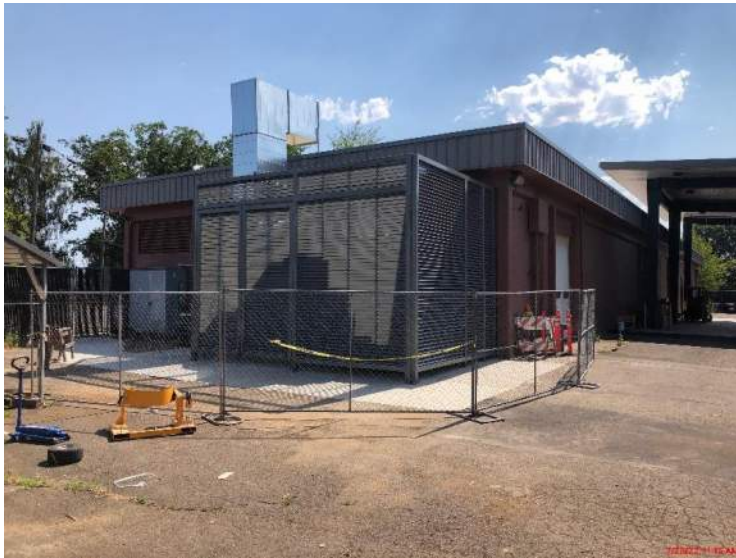
Dust collector screen
