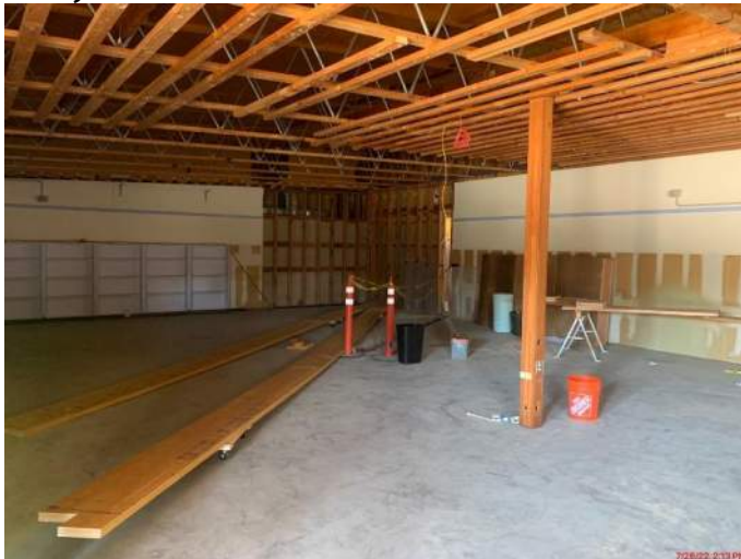
Seismic work at library
