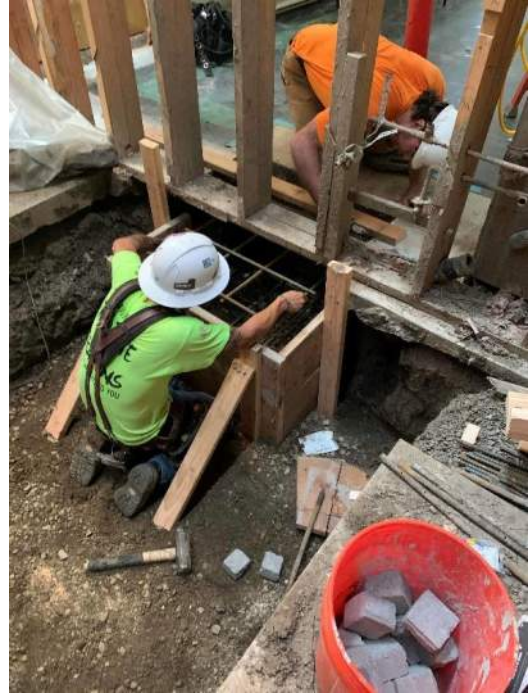
New interior footing work
