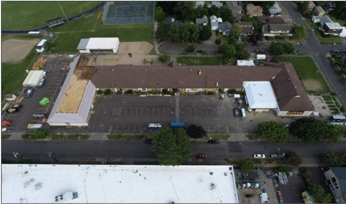
Aerial of Franklin site in mid-July
