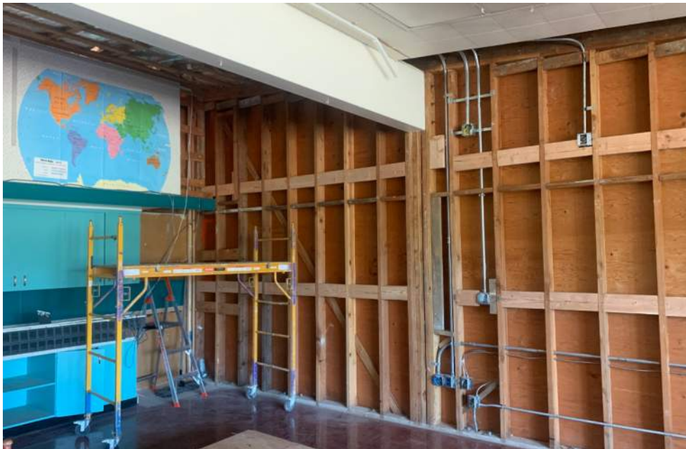
Classroom seismic blocking and technology rough-in
