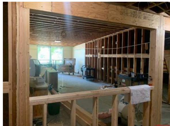
Framing for new offices
