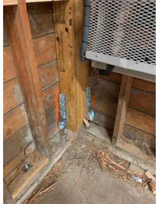
New seismic hold downs in existing walls
