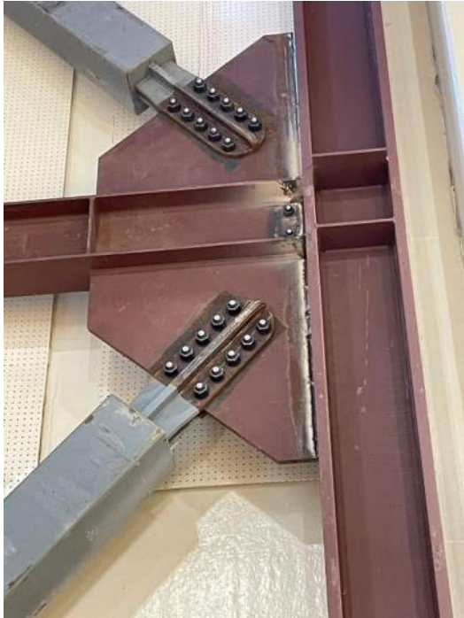
Bldg. A – Brace frame up close
