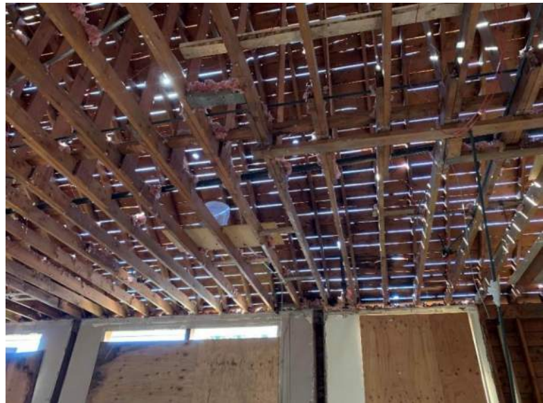
Office Ceiling demo progress
