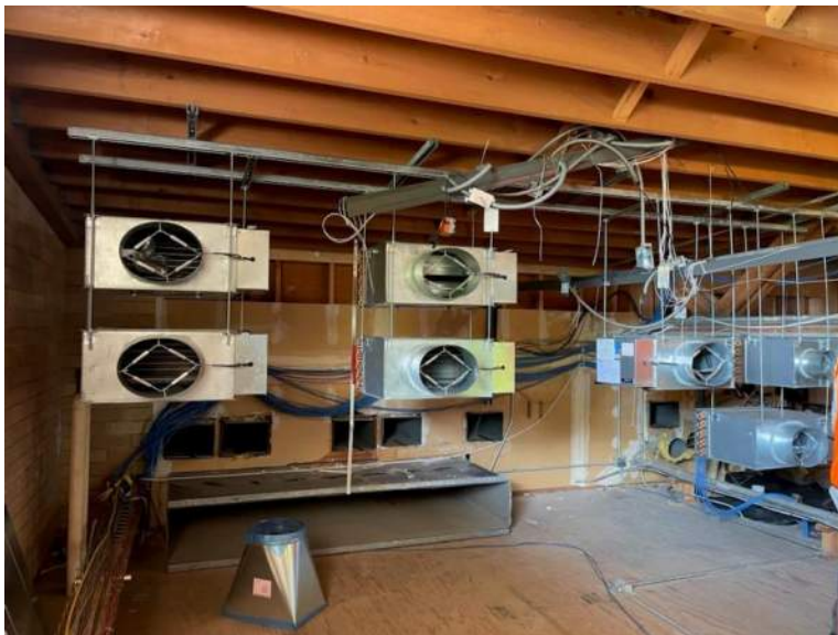
CMS – Classroom wing mechanical room HVAC rebuild
