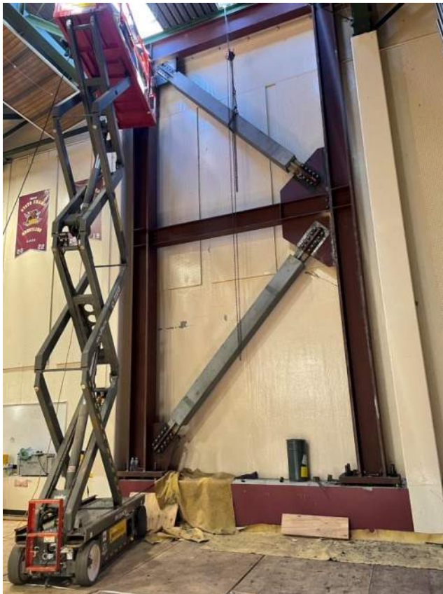
Bldg. A – Brace frame installed
