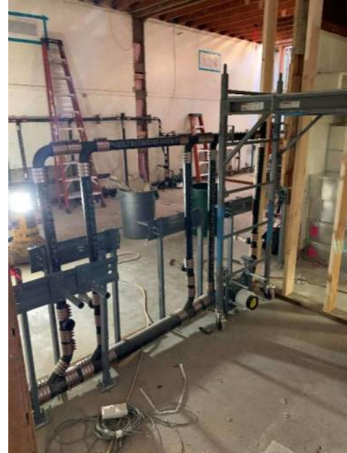
New plumbing rough-in
