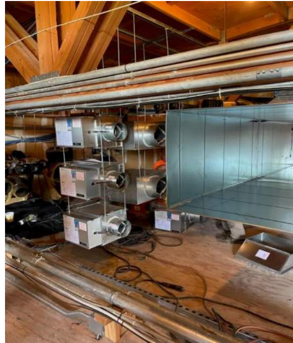
CMS – Mechanical room reconstruction progress
