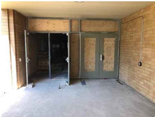
CMS – Progress on new ADA double entry to classroom wing
