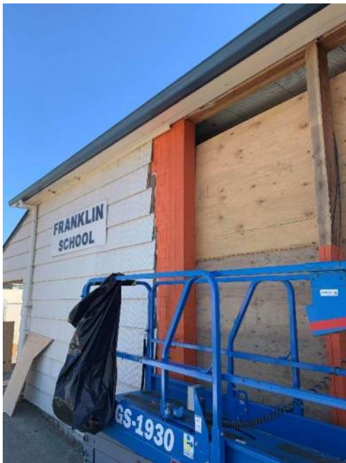
Windows removed and waterproofing installation
