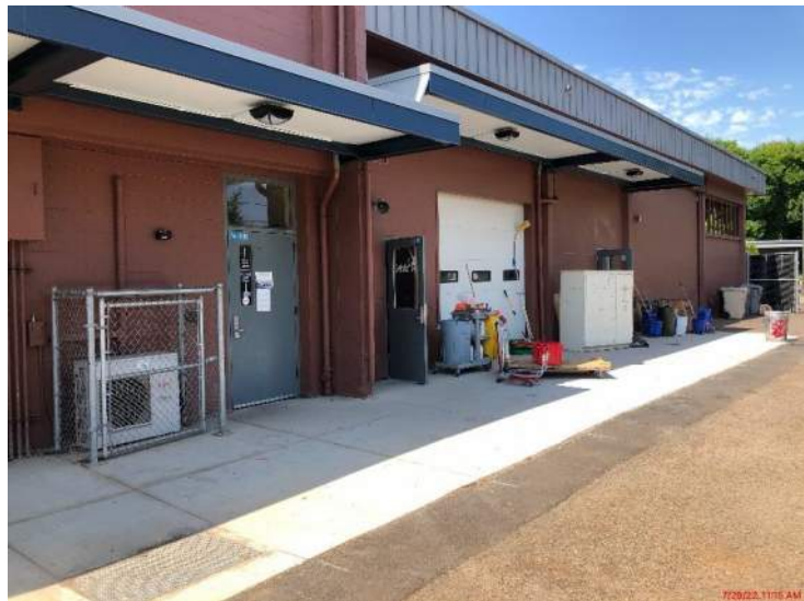
AT south canopies complete
