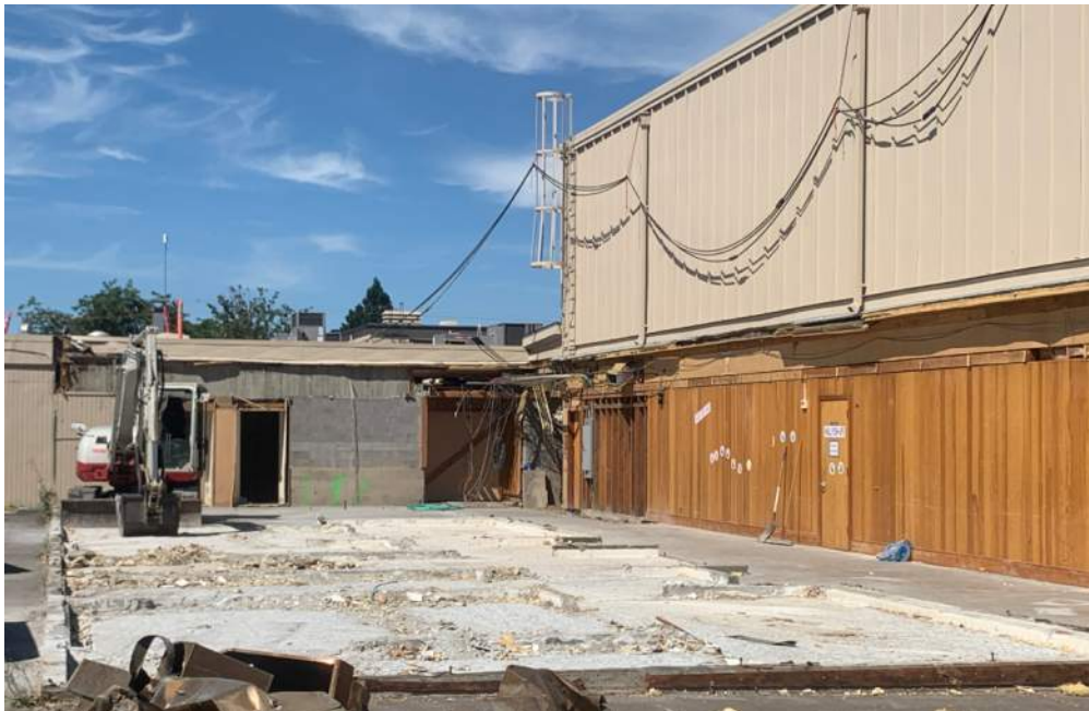
Locker room demolition
