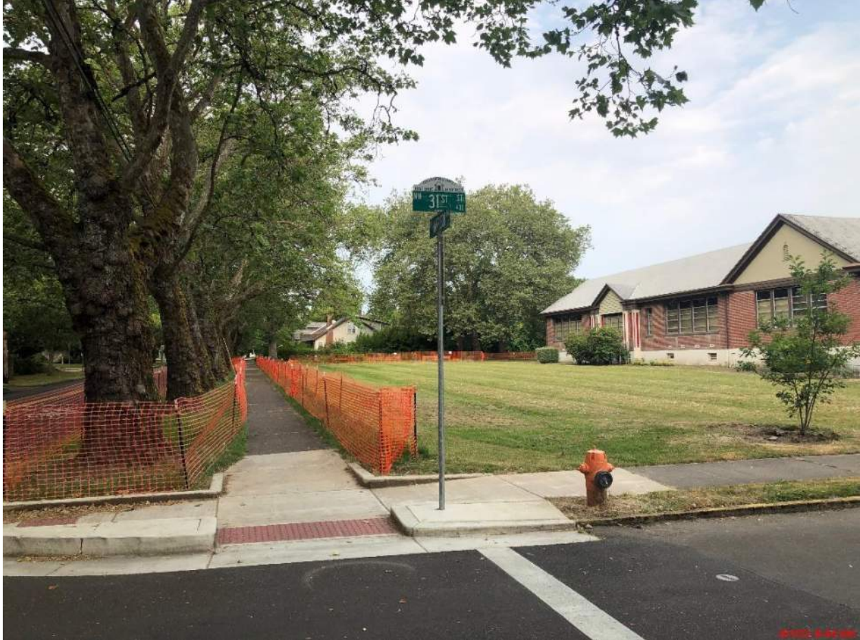
College Hill – Tree protection installed ahead of permit issuance as required
