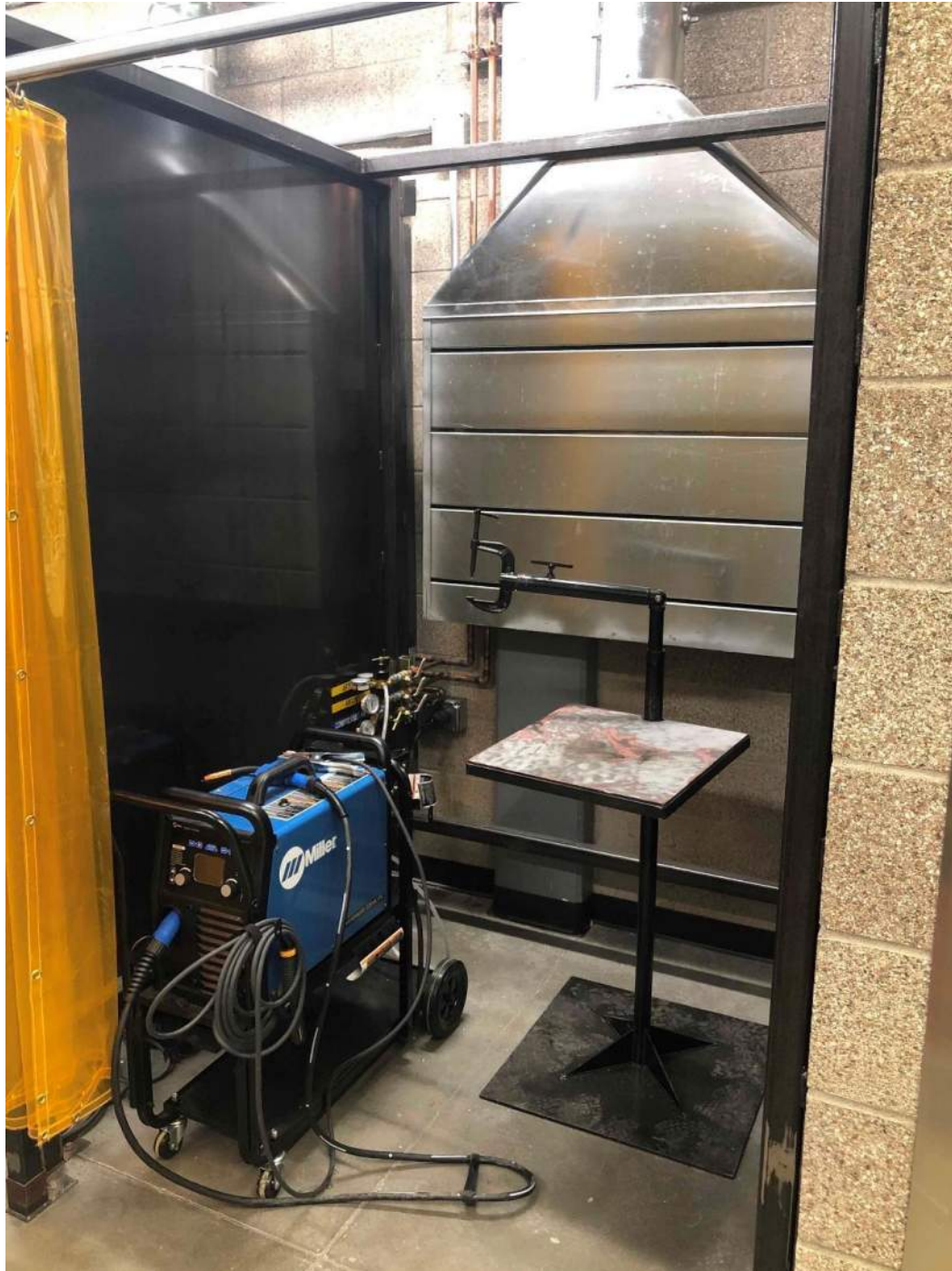
Completed Welding Booth
