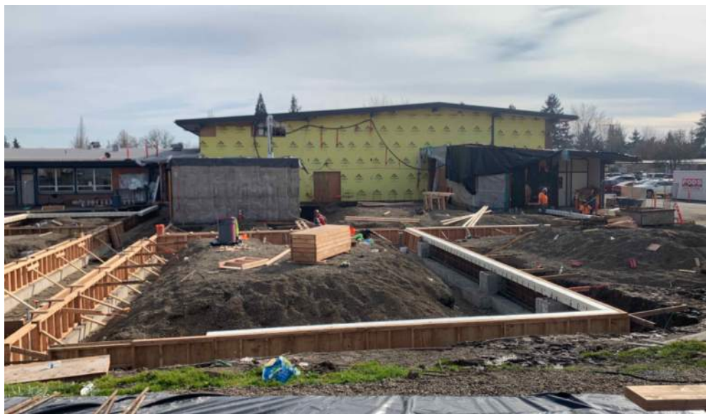
Footings for new classroom addition
