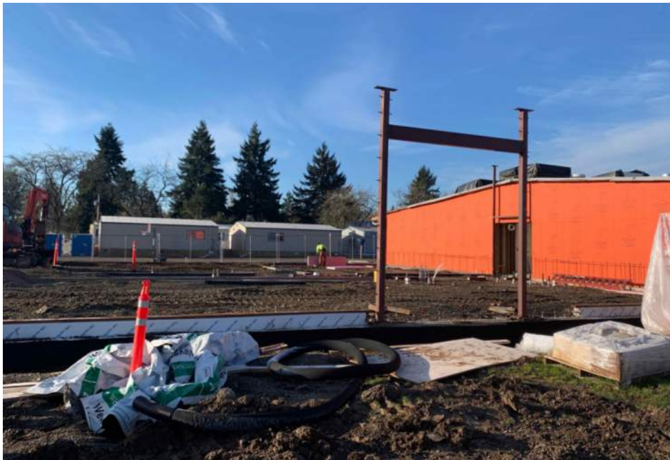
Slab Prep at Classroom Addition
