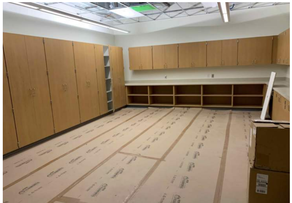
Staff Work Room
