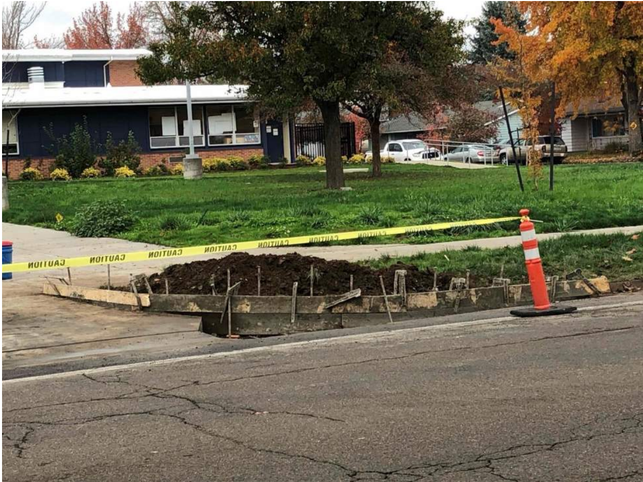
Final construction for driveway approach
