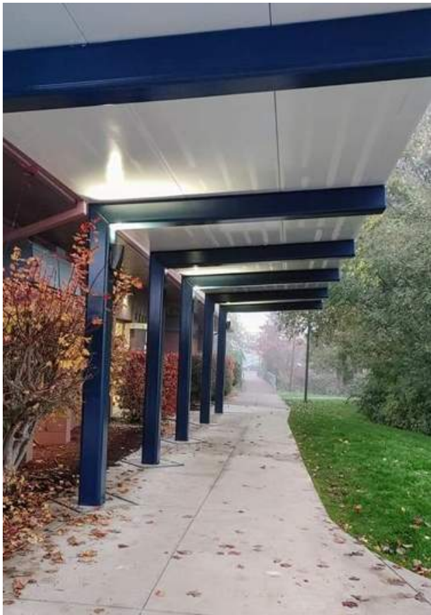
Covered walkway nearing completion
