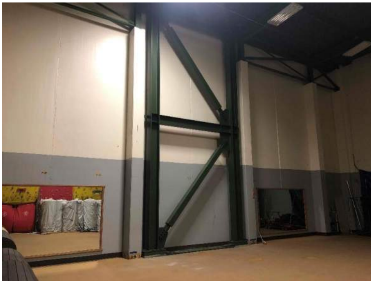
CVHS – Building A - gymnastics seismic frame 100%
