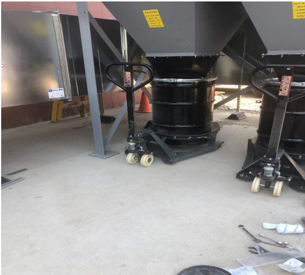
CHS – New dust collector special pallet jacks for changing barrels
