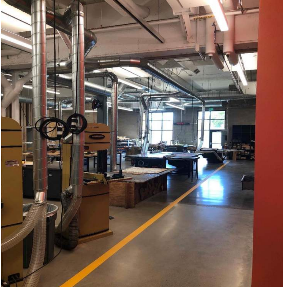
CVHS Building F – Wood shop with dust collector and power connected
