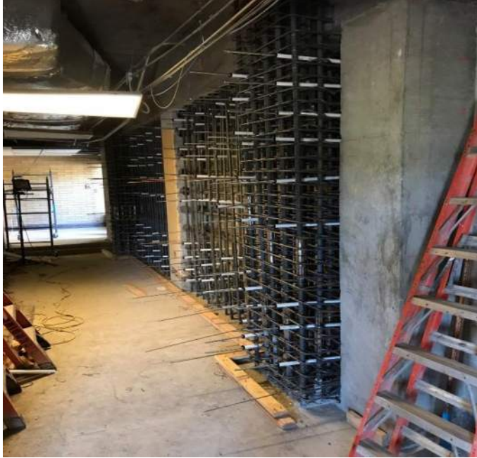
CVHS Building A - Shearwall rebar and formwork
