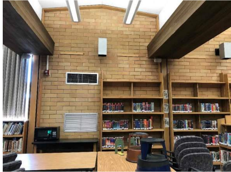
CMS - Previous library ceiling and lighting
