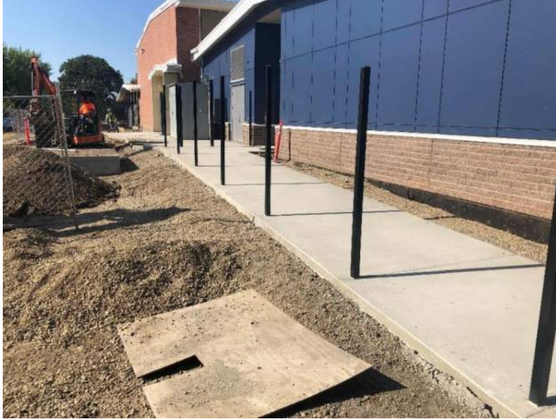
GES – East side ramping and fencing progress
