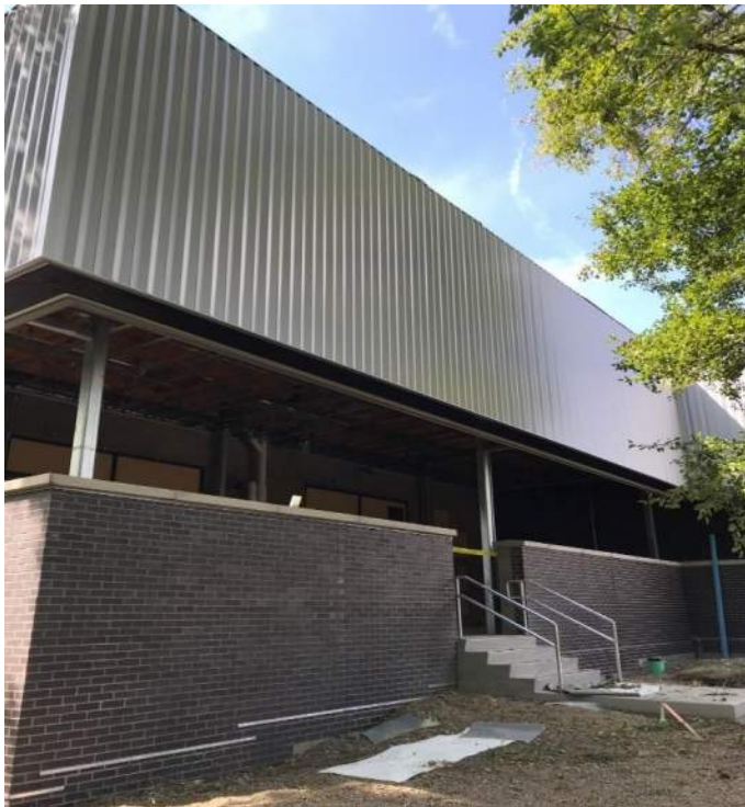
CVHS Building F – Outside of outdoor classroom kiln area
