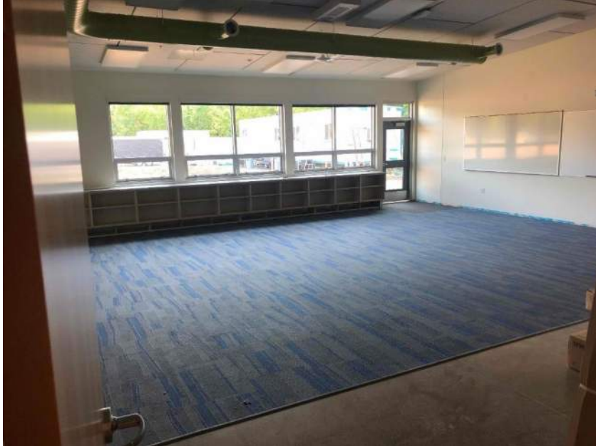
GES – Area C Classroom looking north
