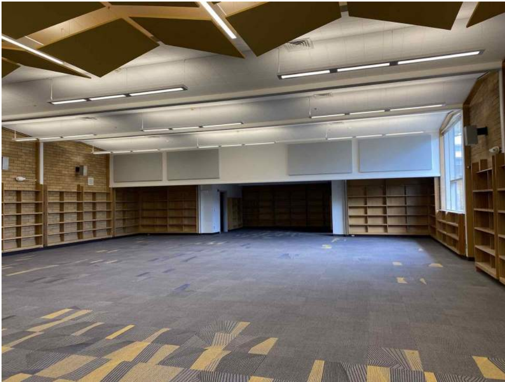
CMS - Front wall & acoustical panels
