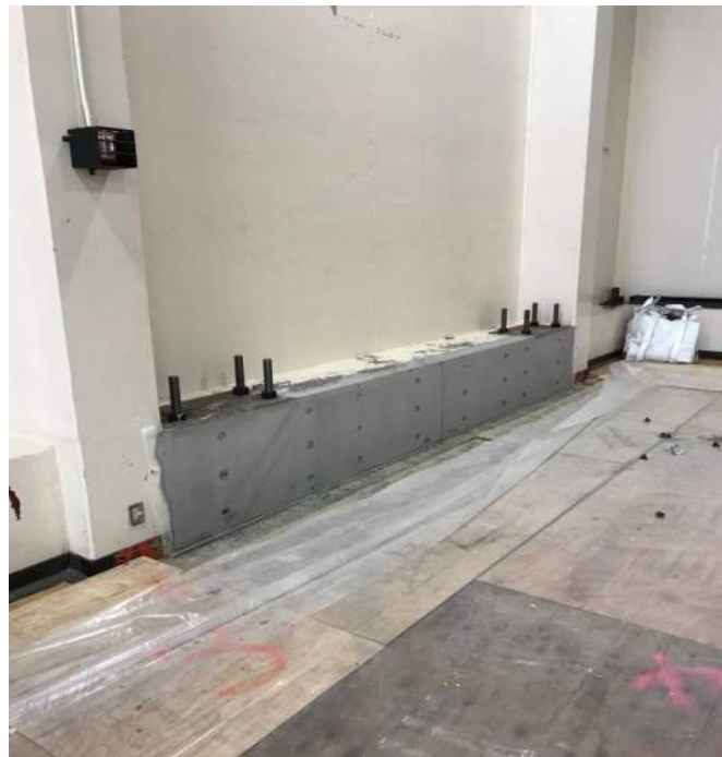
CVHS – Building A Seismic – interior gym improvements placed
