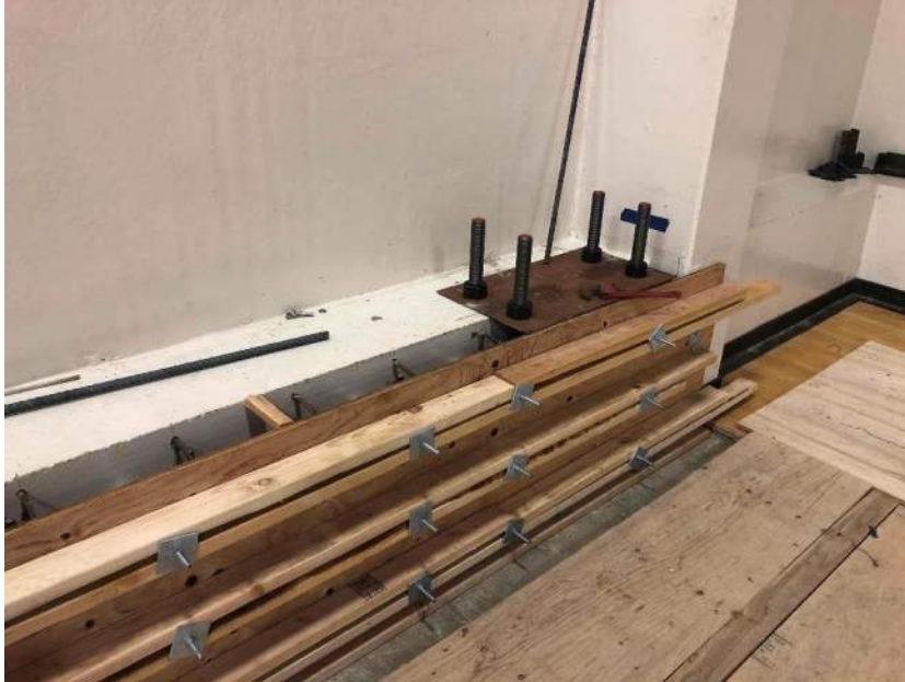
CVHS – Building A Seismic – interior Gym improvements formed
