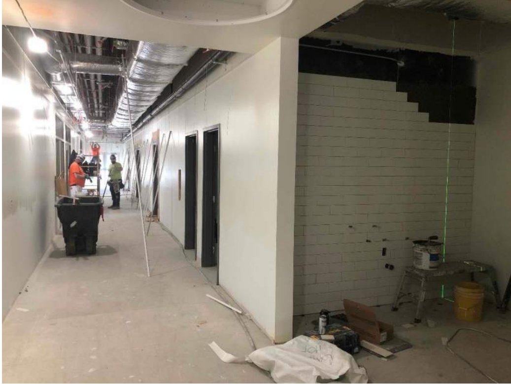
Garfield Area C – finish paint, ceiling grid and tiling
