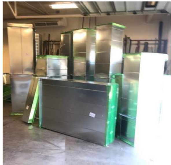
CHS- ductwork staged onsite
