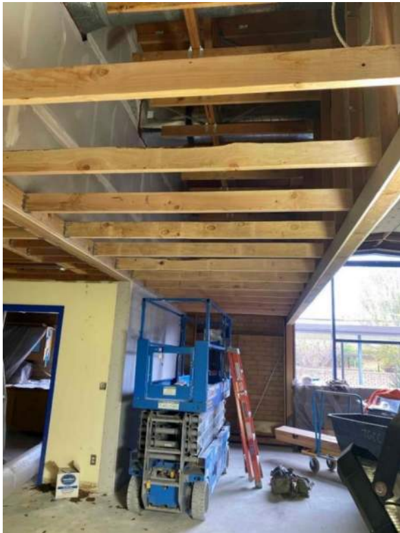
Library HVAC installed and framing going back in
