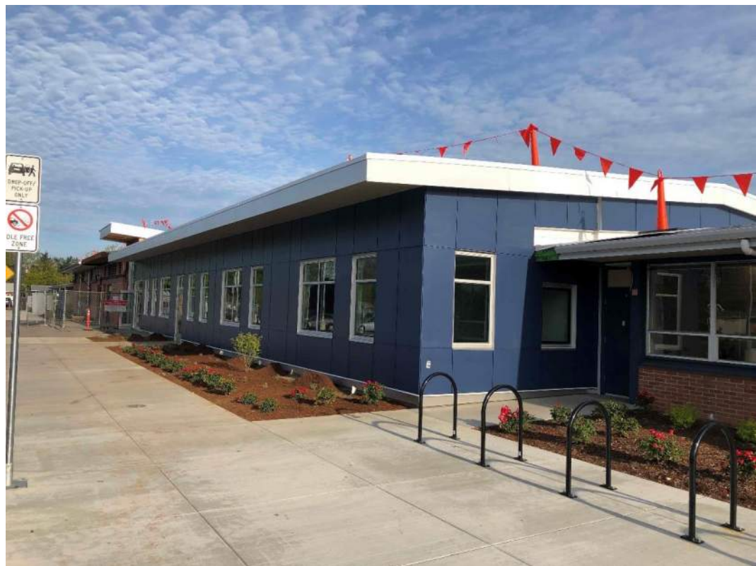
Garfield New Admin exterior
