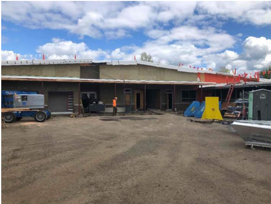
Garfield – West elevation Area C
