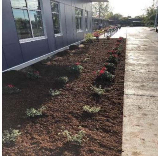
Front office landscaping proceeding now that siding is installed
