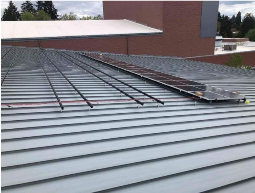
CHS Solar array progress over cafeteria
