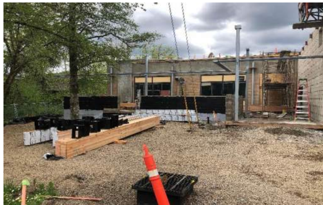
CVHS Outdoor work area – brick & roof framing to start
