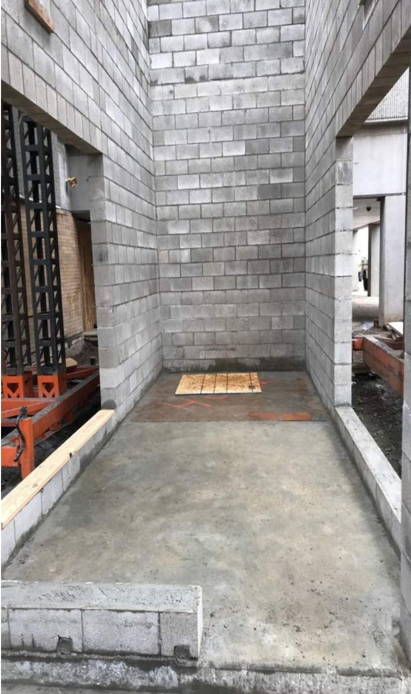
CVHS new elevator walls
