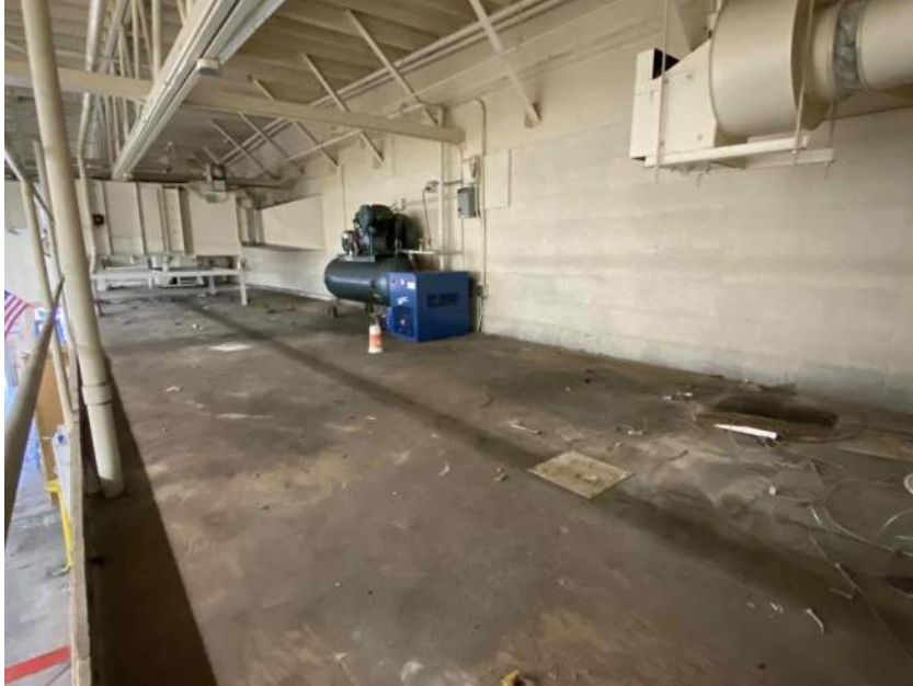
CHS Autos mezzanine ready for new construction work
