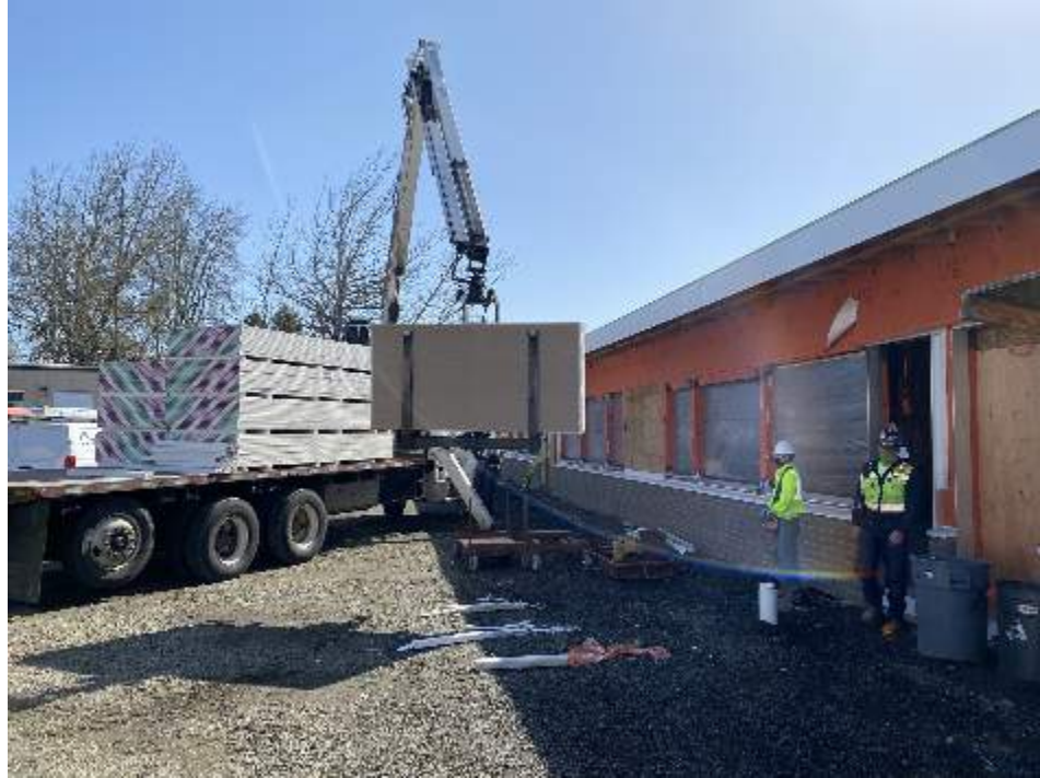
Garfield Areas C – drywall delivery at the new classroom addition
