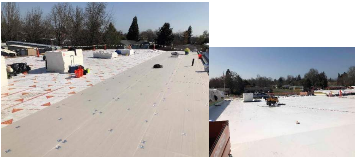
Garfield Area C – Roofing progress photo North (left) south (right)
