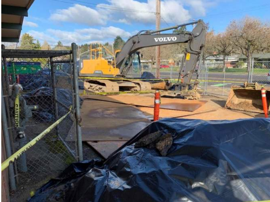
Oil Tank Removal
