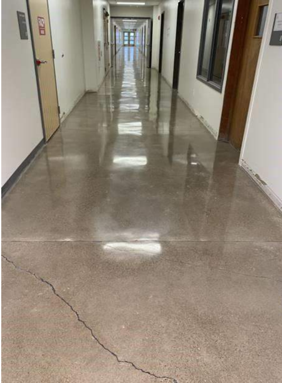
Garfield – Existing concrete, now polished and sealed
