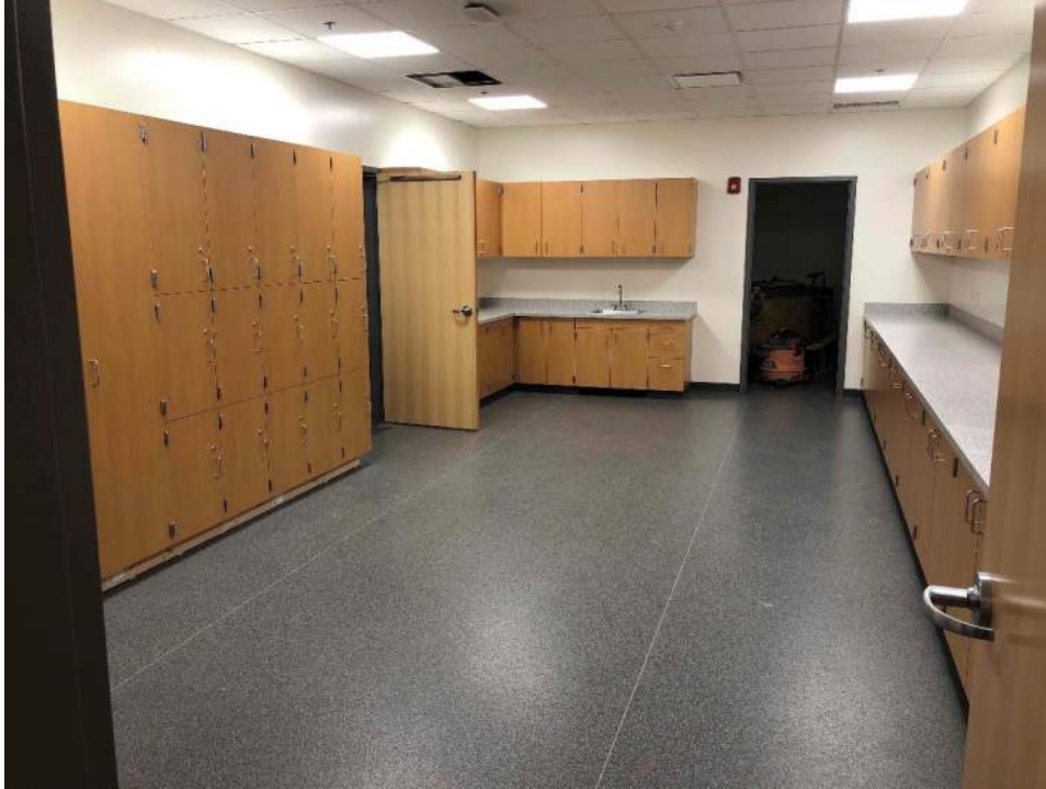
Staff work room - casework done
