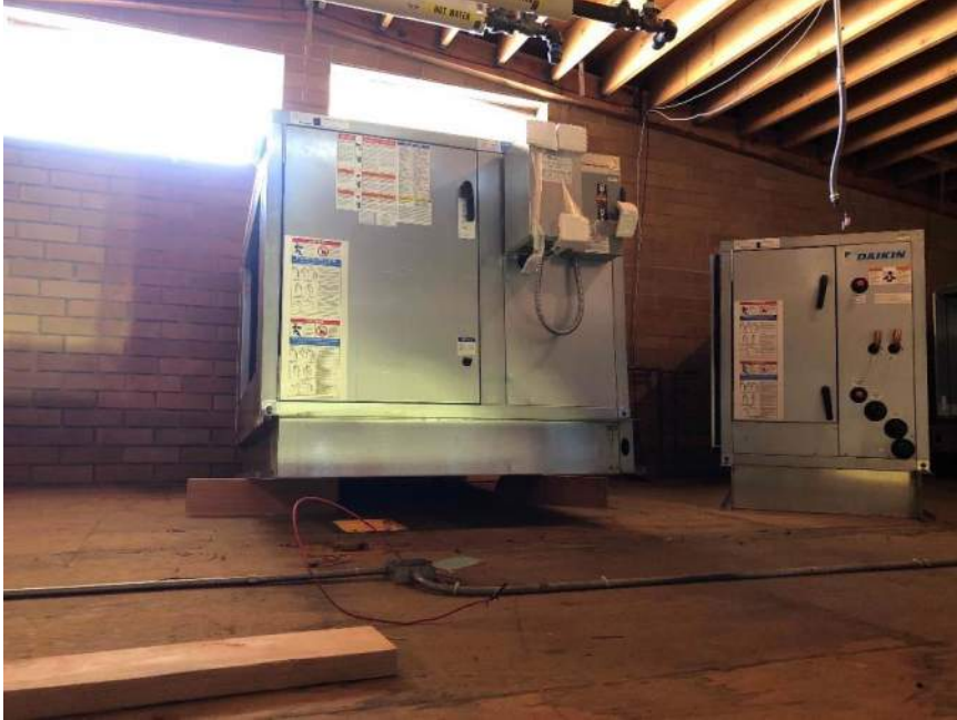
New HVAC installing at north mechanical mezzanine
