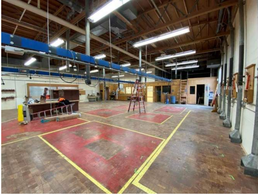
CHS woods ready for construction
