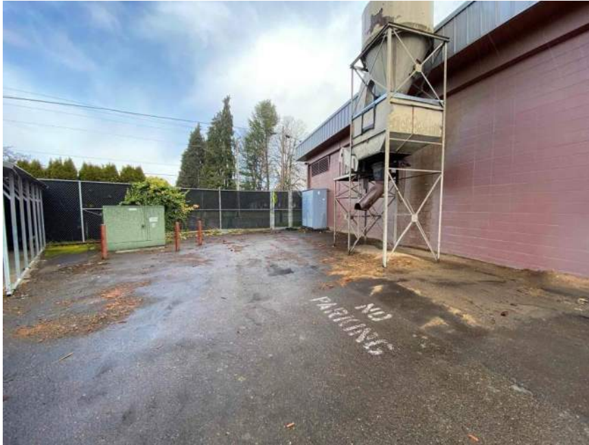
CHS dust collector yard area cleared
