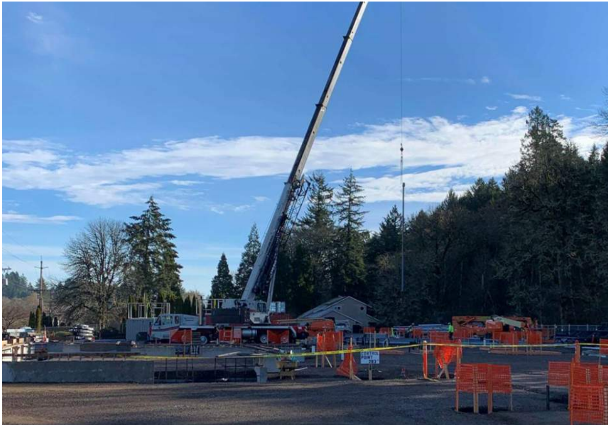
First steel column being set
