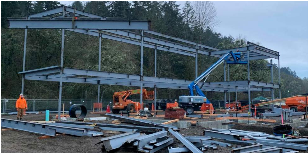
Ongoing structural steel erection
