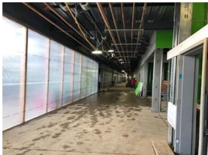
Interior framing and mechanical work underway
