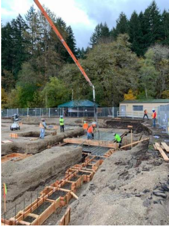
Pumping concrete into footings
