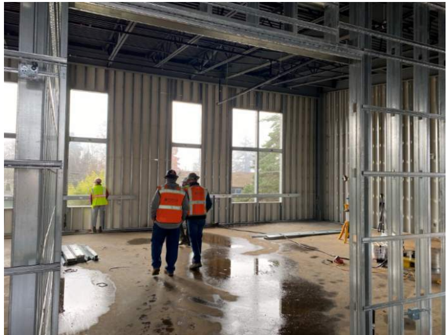
Second Floor Classroom taking shape – lots of natural light
