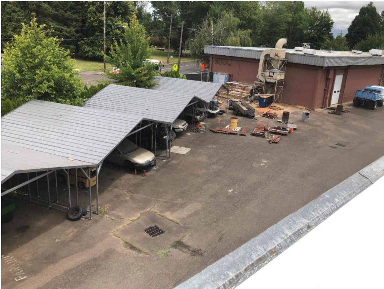
Current view of the CHS CTE yard
