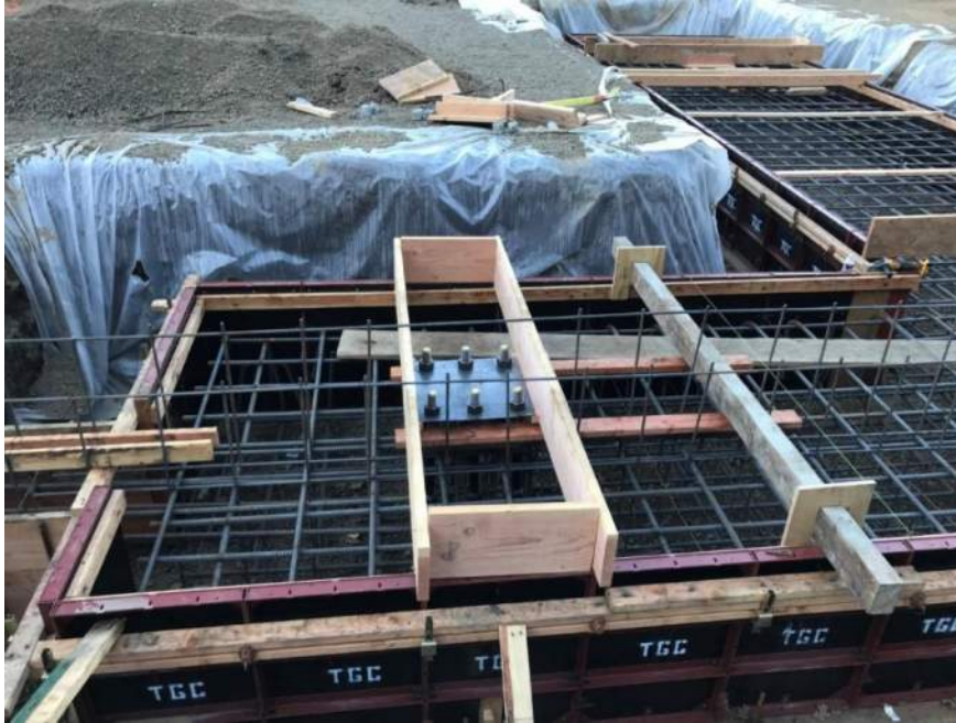
A close-up view of the formwork and rebar
