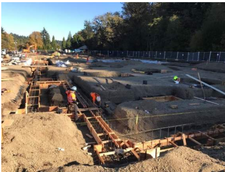
A view of the formwork and rebar
