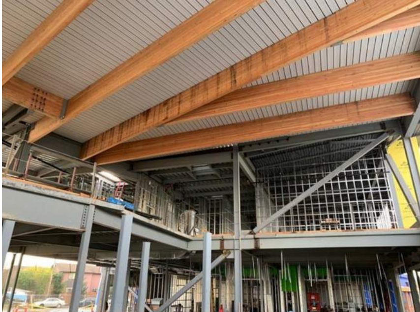
Commons area with exposed wood beams
