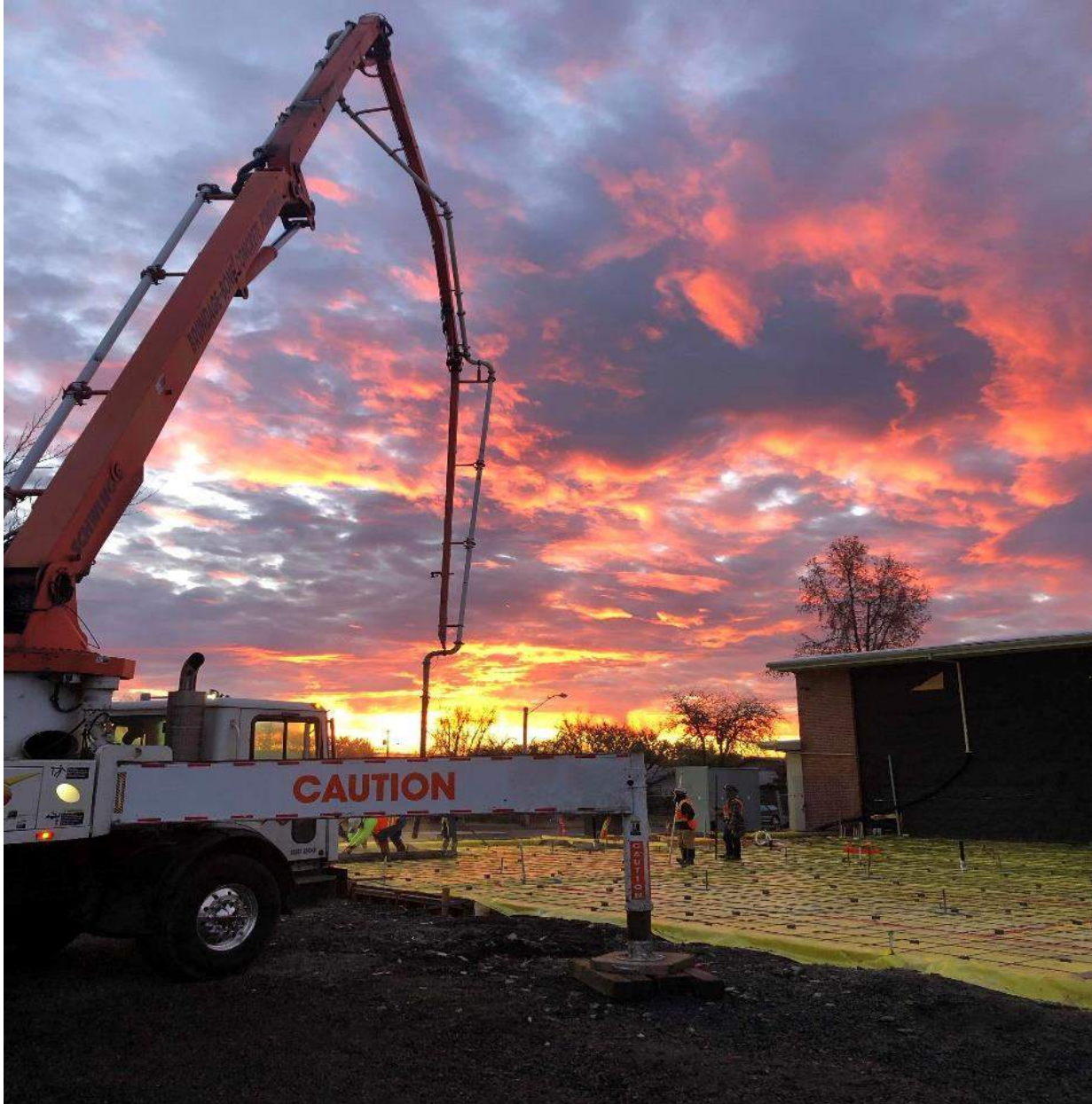
Early morning Area C final concrete slab placement
