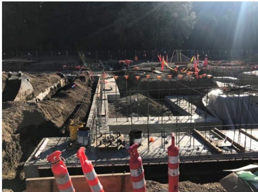
A view of the footings after a concrete pour
