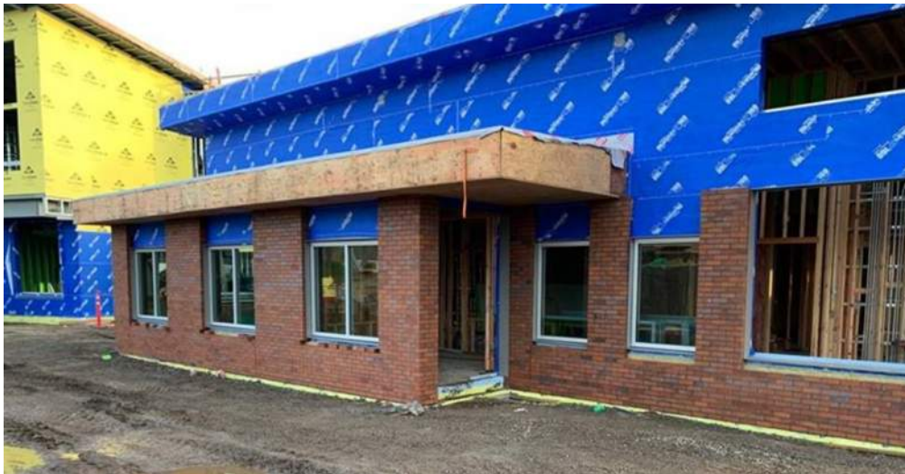
Benton County Lincoln Health Center making great progress
