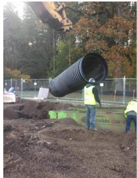
Large storm drainage piping being placed
