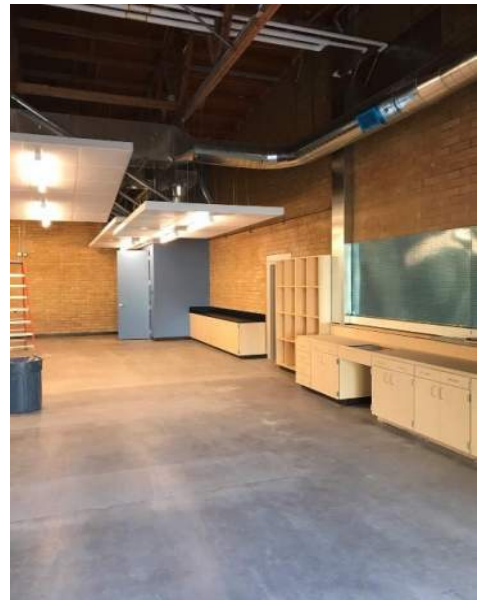
More STEAM Lab area progress
