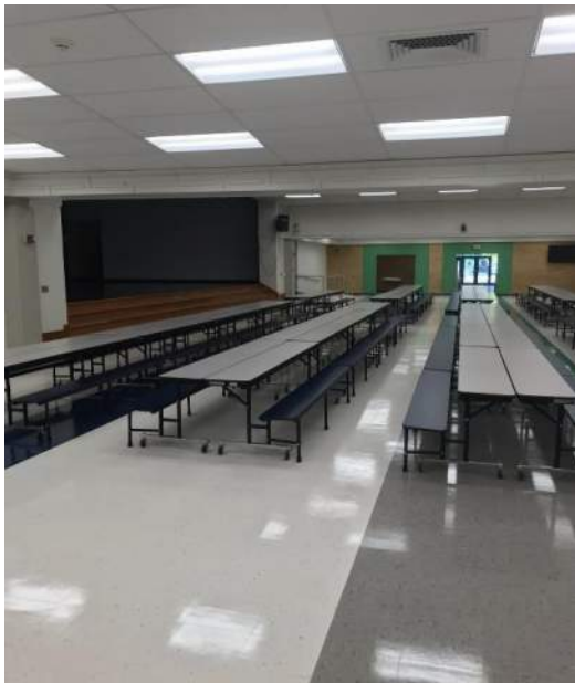
Cafeteria flooring installation & wax complete & tables back in
