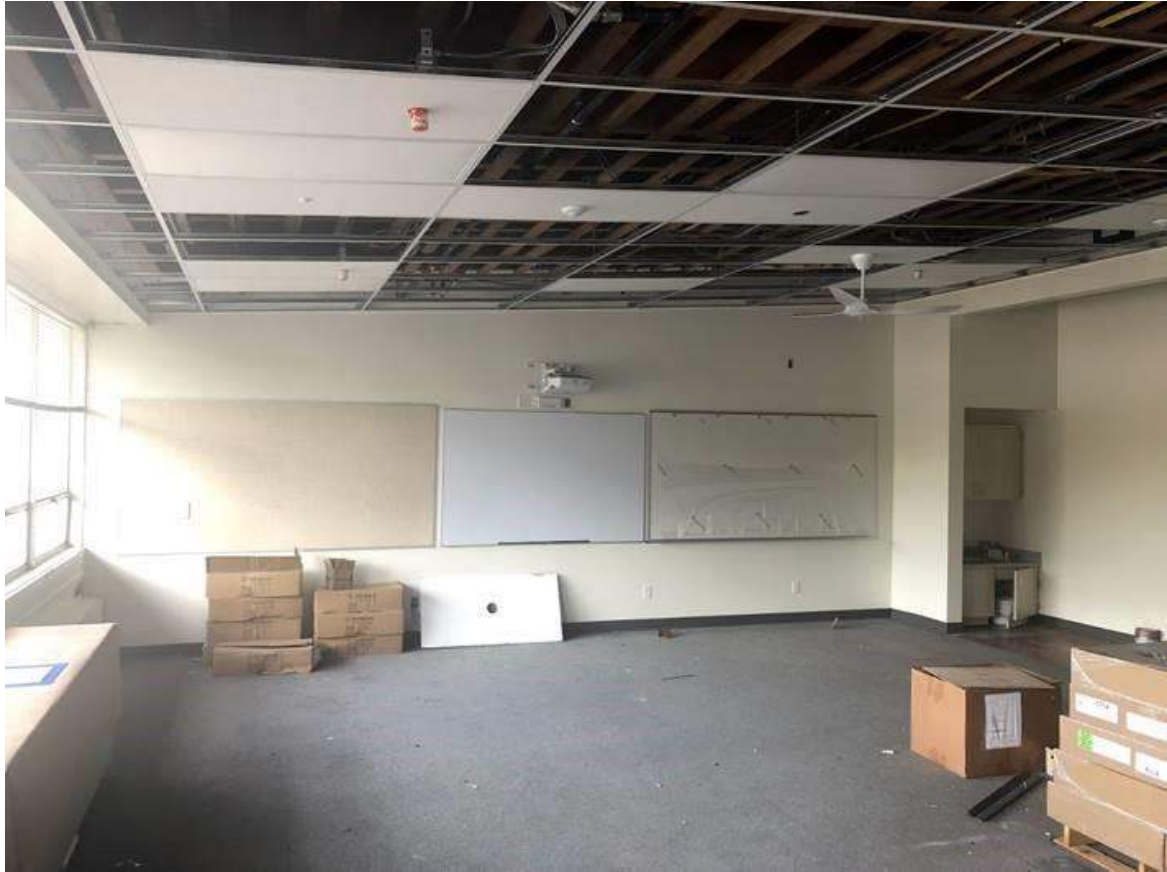
New teaching wall and new ceilings – construction progress
