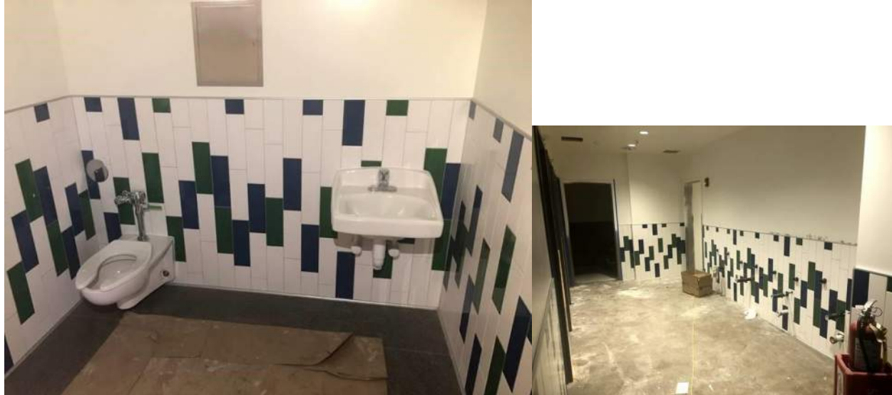
New restrooms – construction progress
