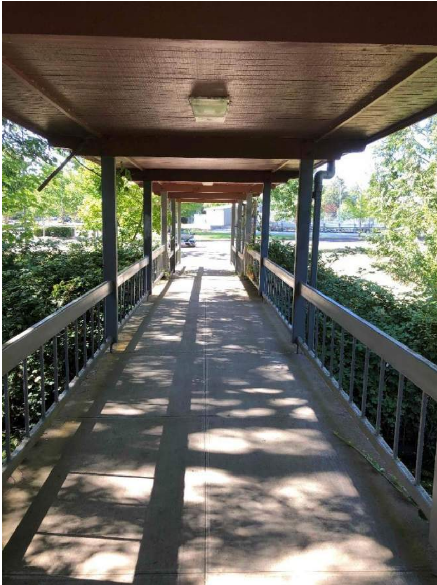
Future connection point (east bridge looking south) for new covered walkway
