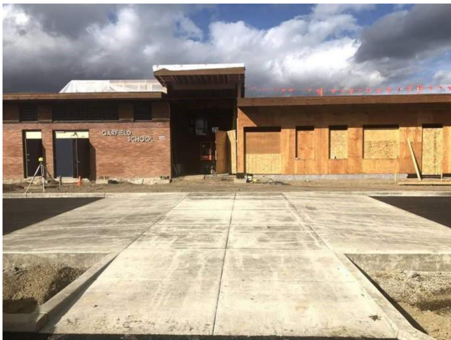
New front entry approach construction progress
