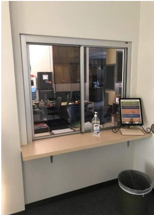
New front office transaction window (from lobby side)
