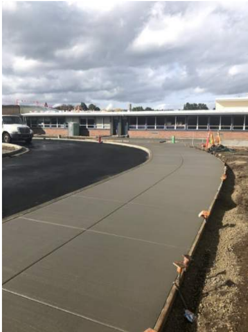
New sidewalk coming into front of the school
