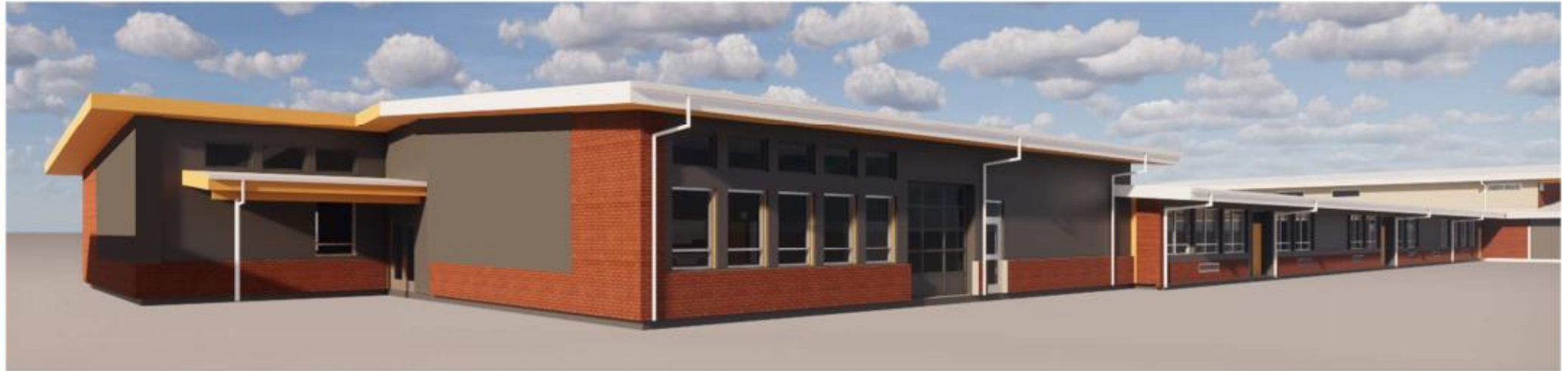
Learning Wing Addition
