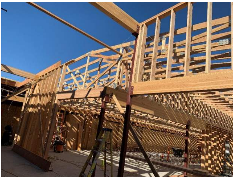
New office framing
