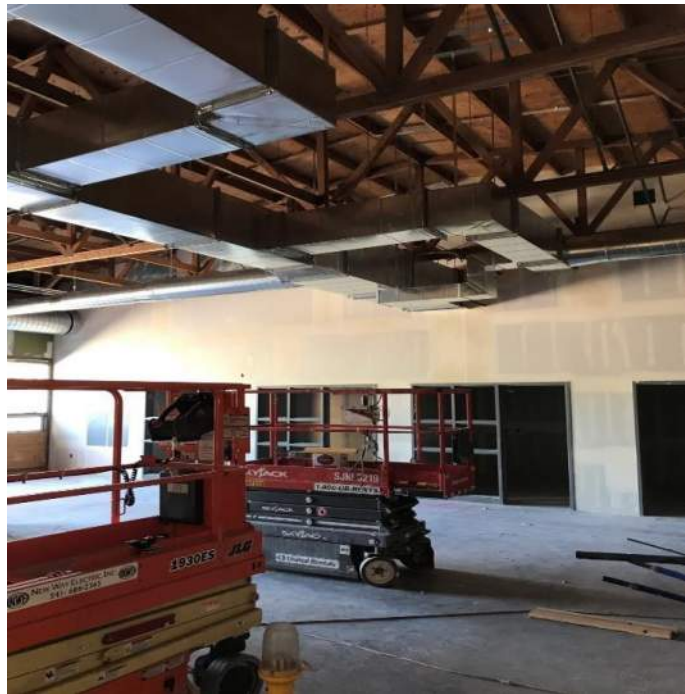
STEAM Lab area progress
