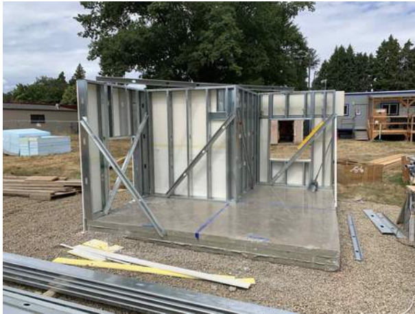
Mockup of polished concrete slab and framing
