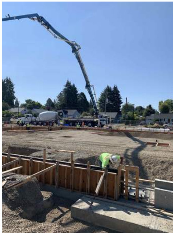
Concrete pump in action for placing wall concrete
