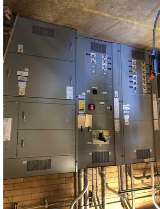
Cheldelin new switchgear installation
