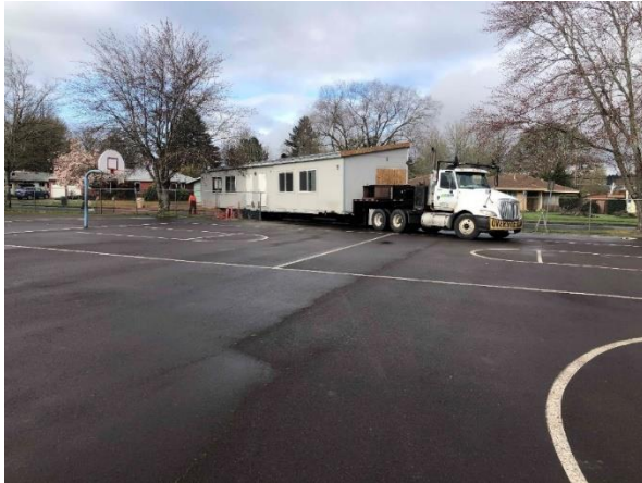
Garfield Modular Classrooms are moved in place
