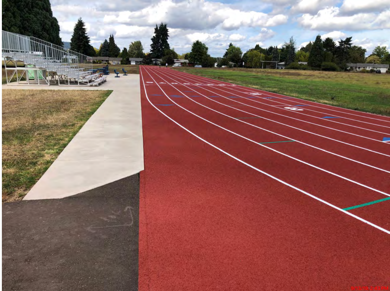
Track Resurfacing completed
