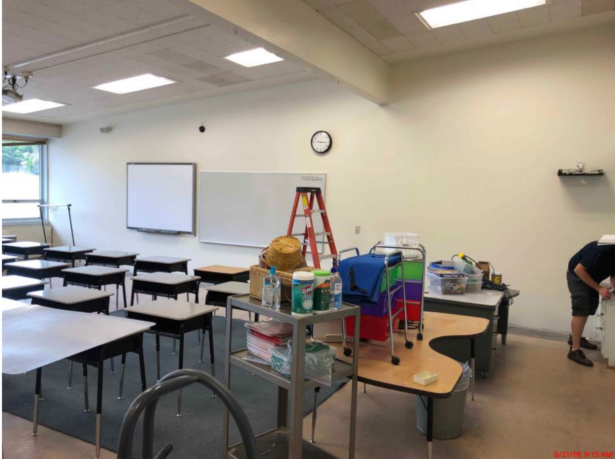
New classroom wall finishes
