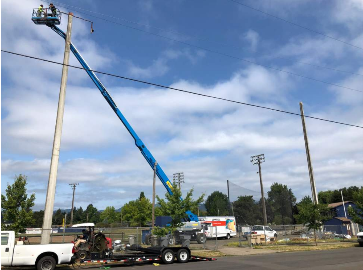
Taylor Field Light replacement
