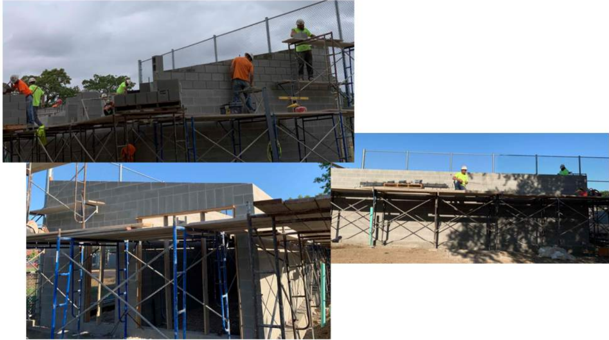
Masonry construction is underway at the CHS Softball dugouts
