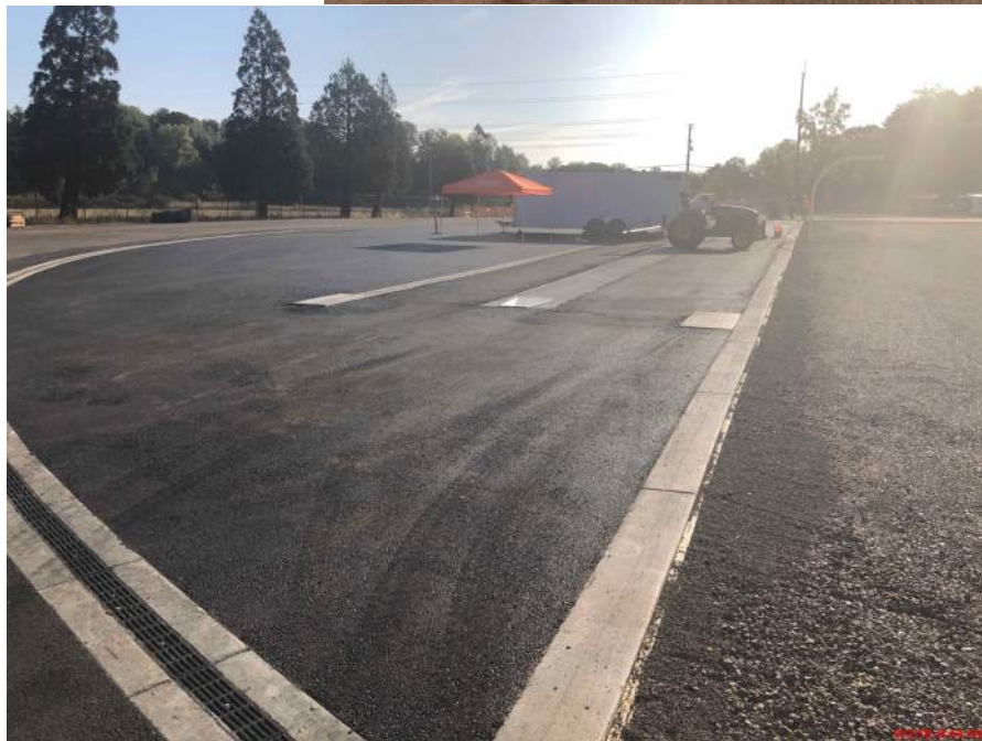
CVHS D Zone paving completed
