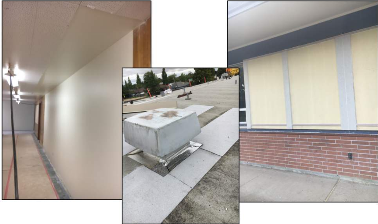
Hallway, roof, and window infill seismic upgrades are completed
