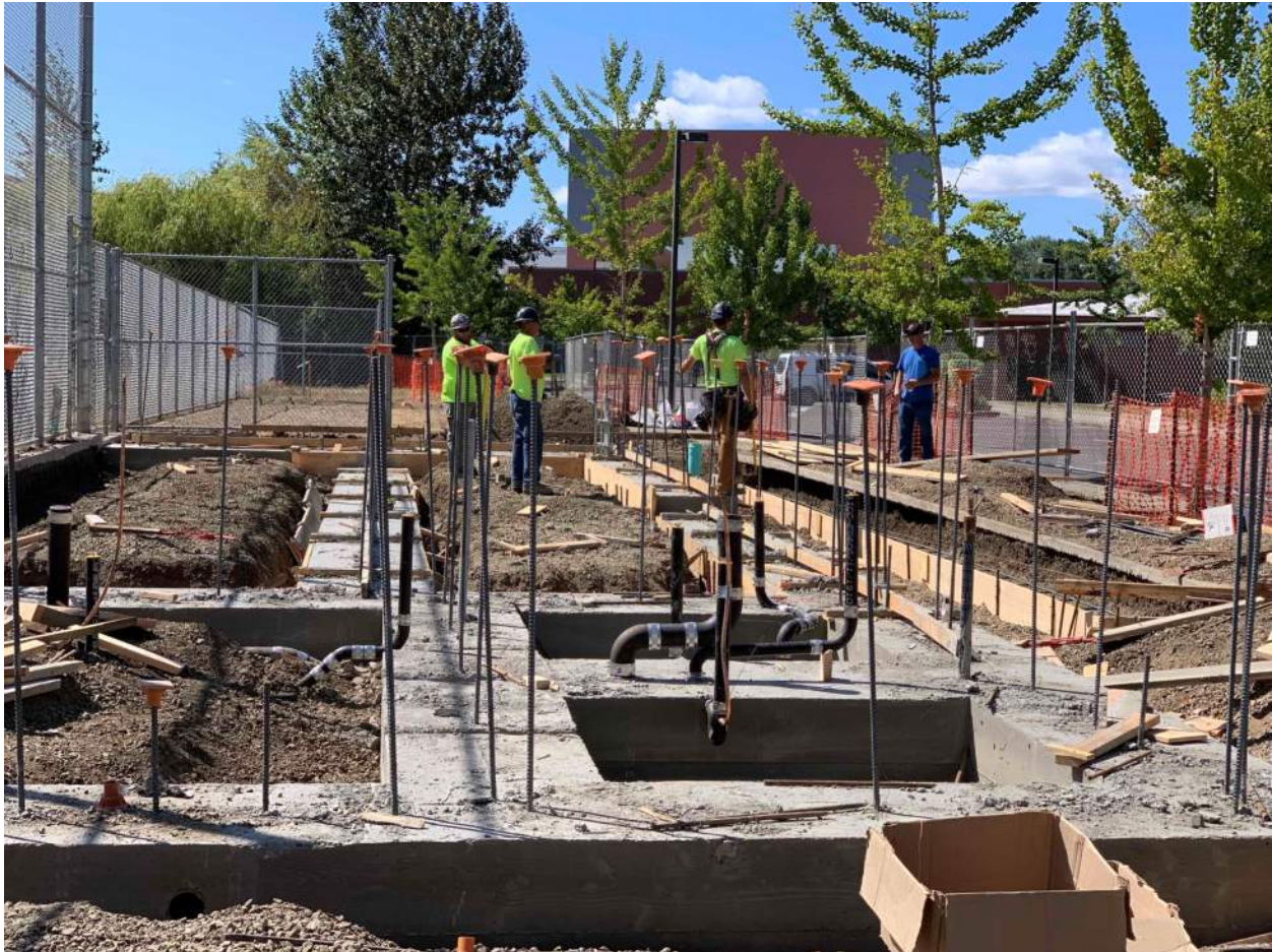
CHS Softball footings, rebar and underground plumbing ready for masonry installation
