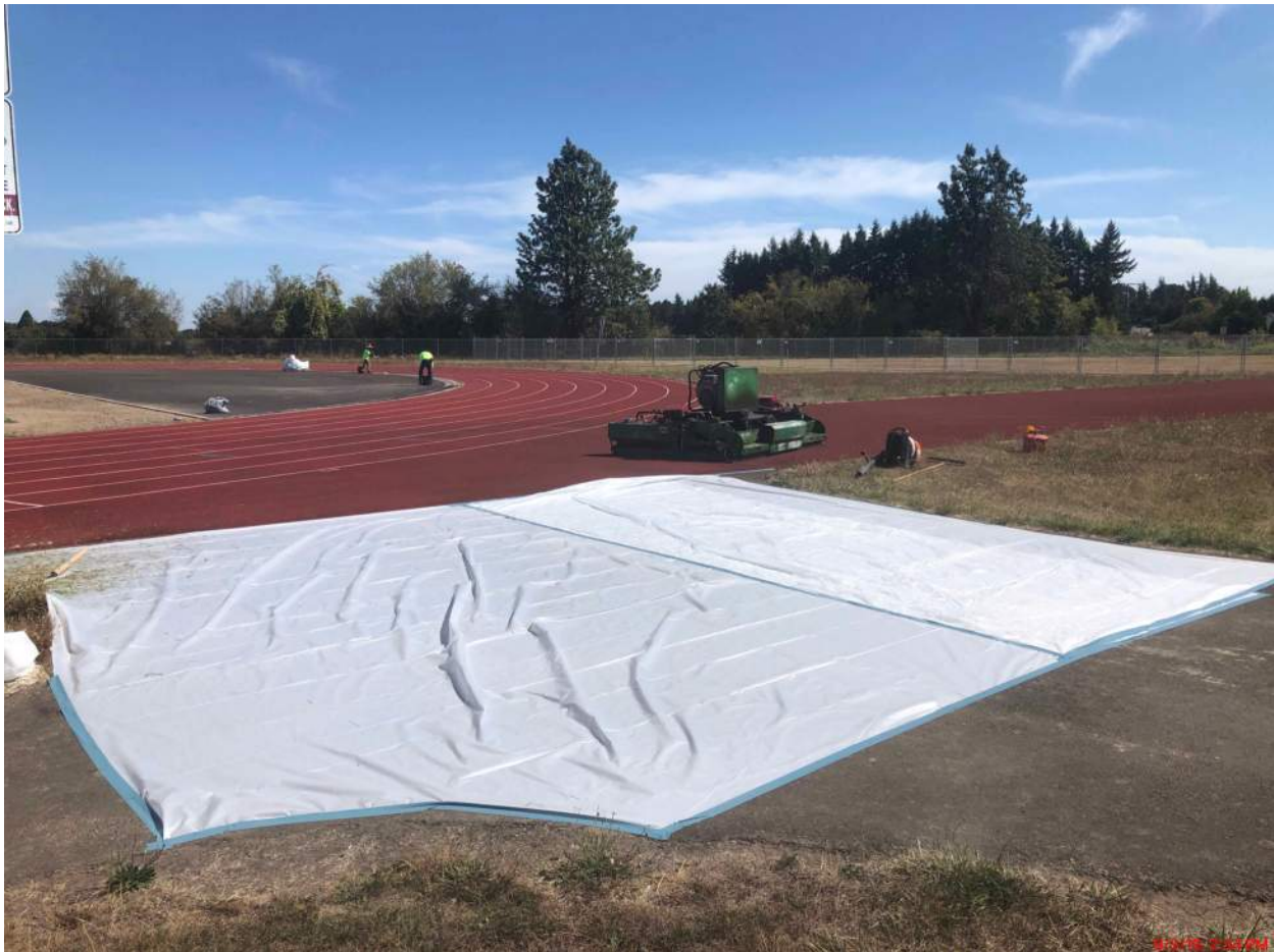
Track Resurfacing begins
