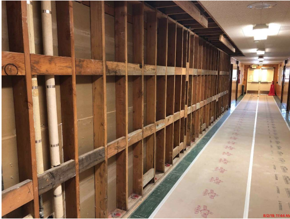
Jefferson hallway work
