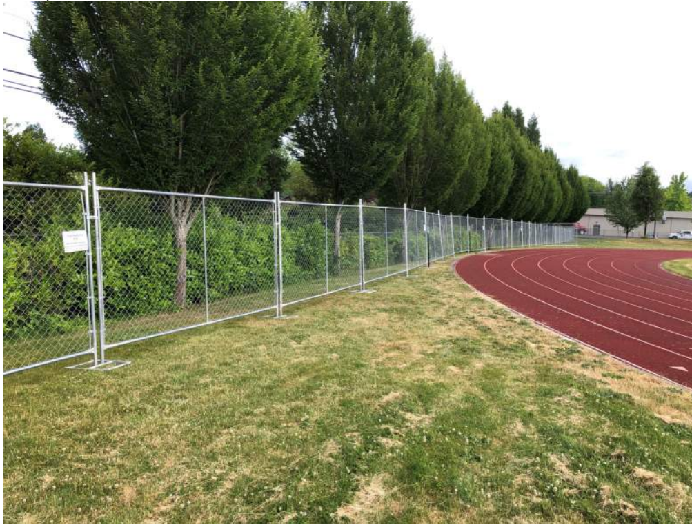
Tree Protection installed
