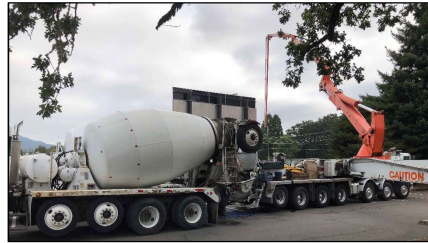
Pumping concrete curbs at track
