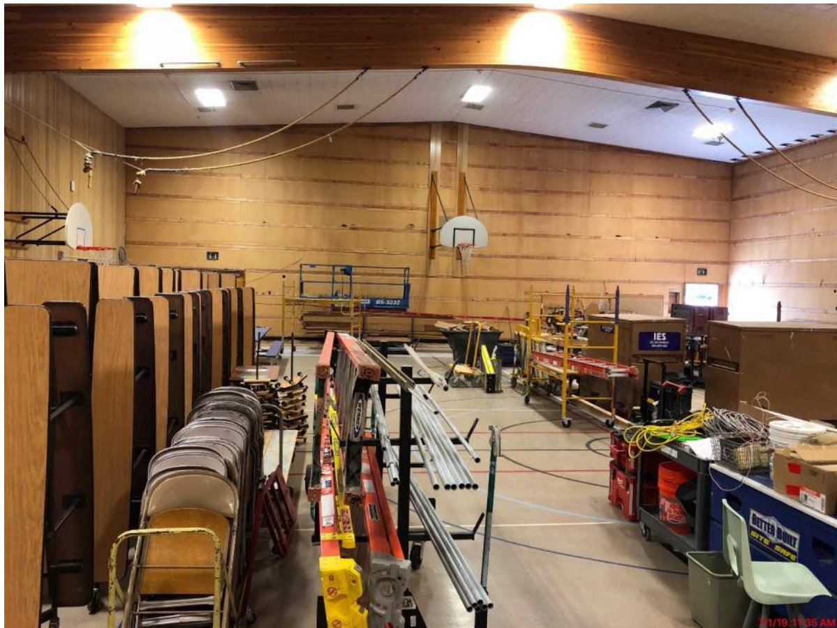
Staging begins for Jefferson summer seismic work
