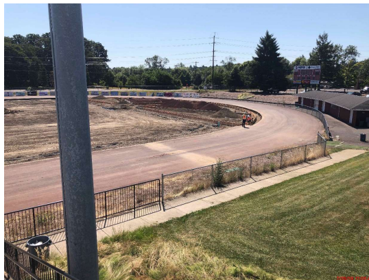
Track and athletic field work underway
