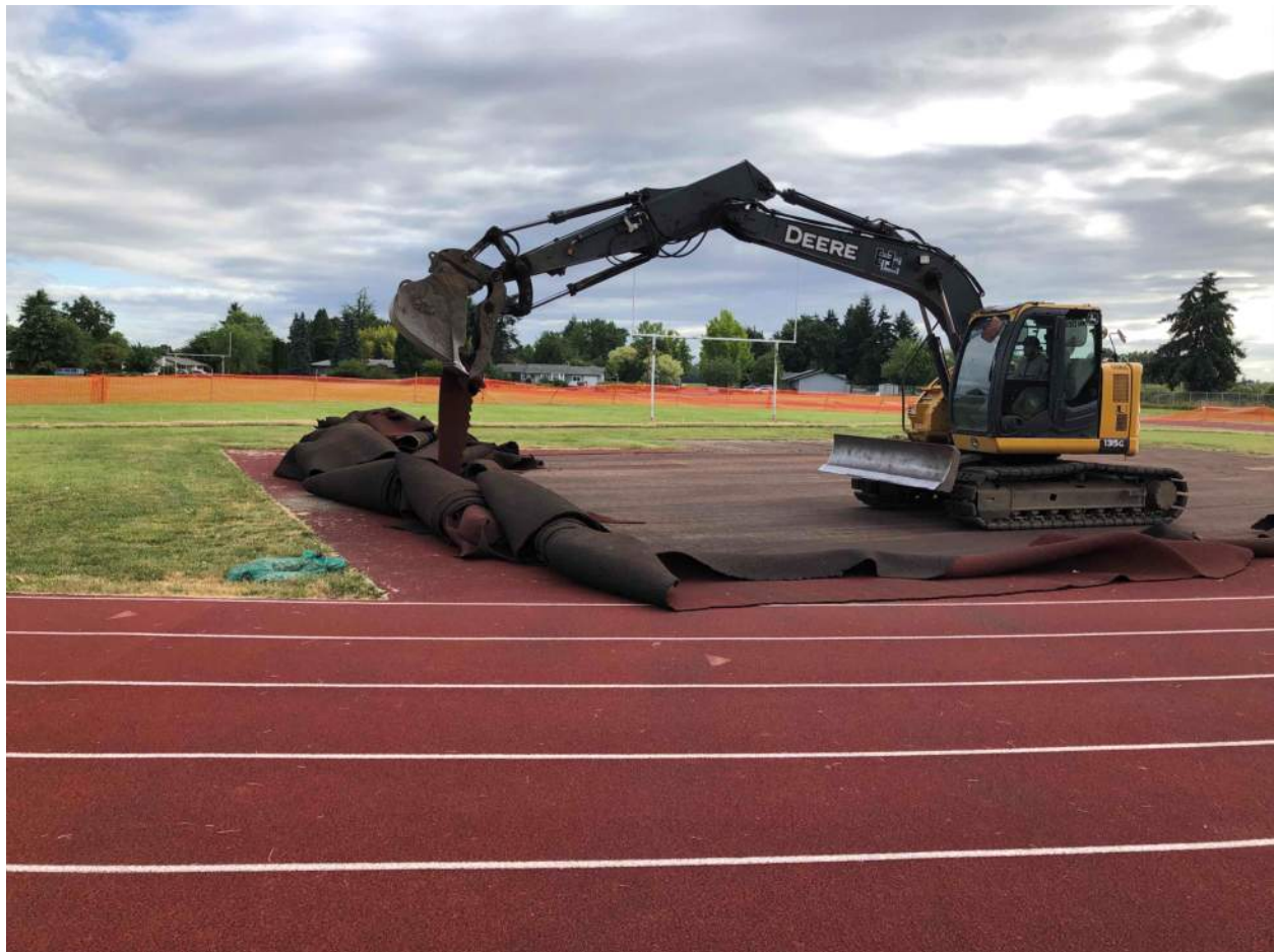
Track Demolition begins
