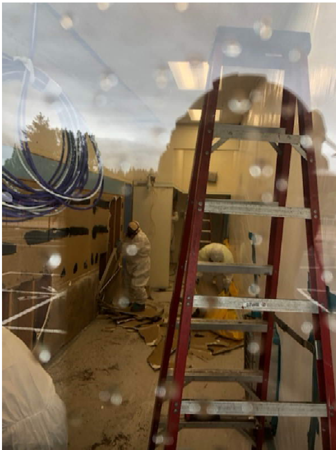
Abatement work in progress, photo through glass
