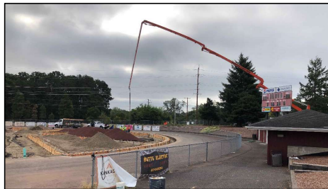
Pumping concrete curbs at track
