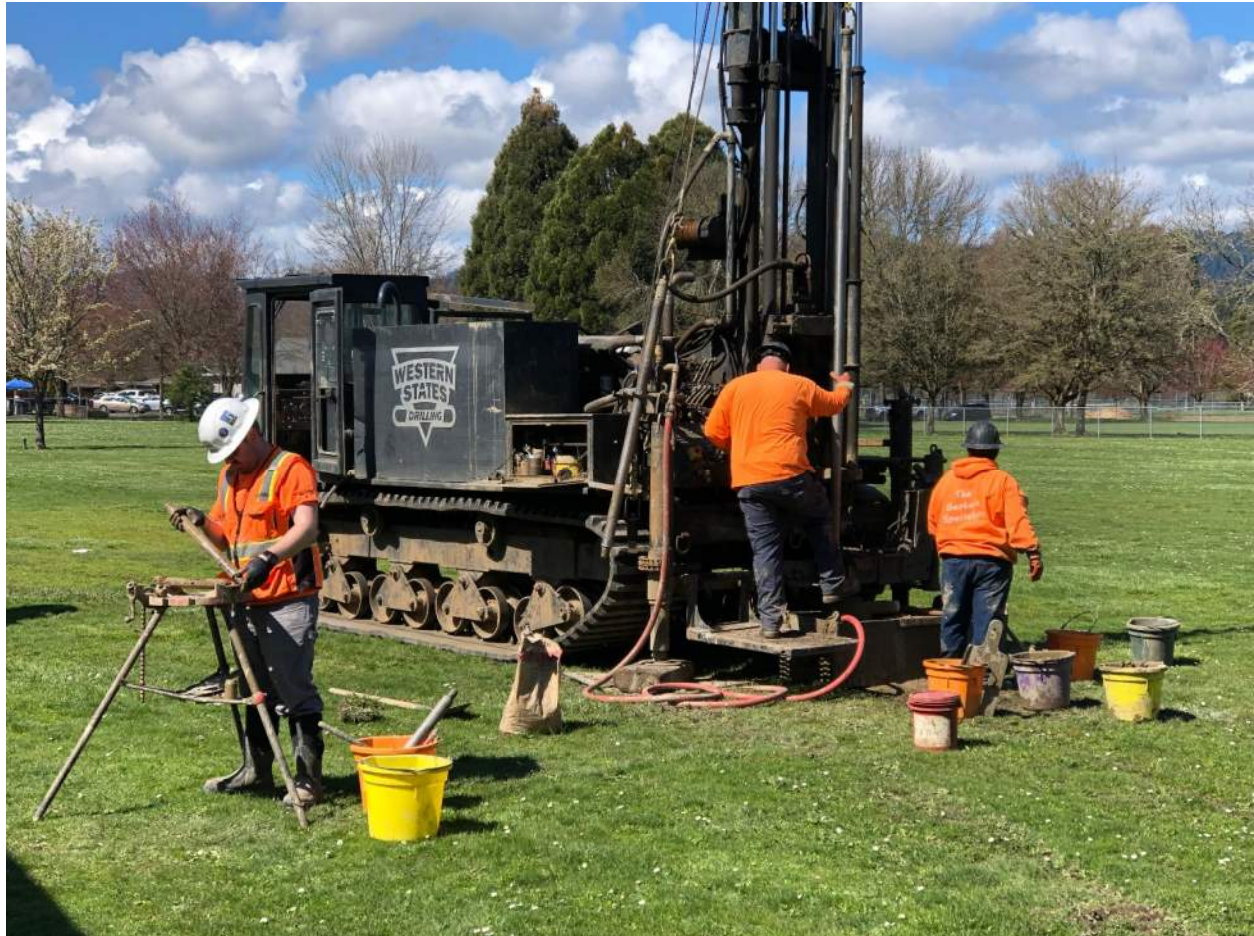
Workers from PBS Engineering and Environmental and Western States Drilling performing the geotechnical survey and associated drilling
