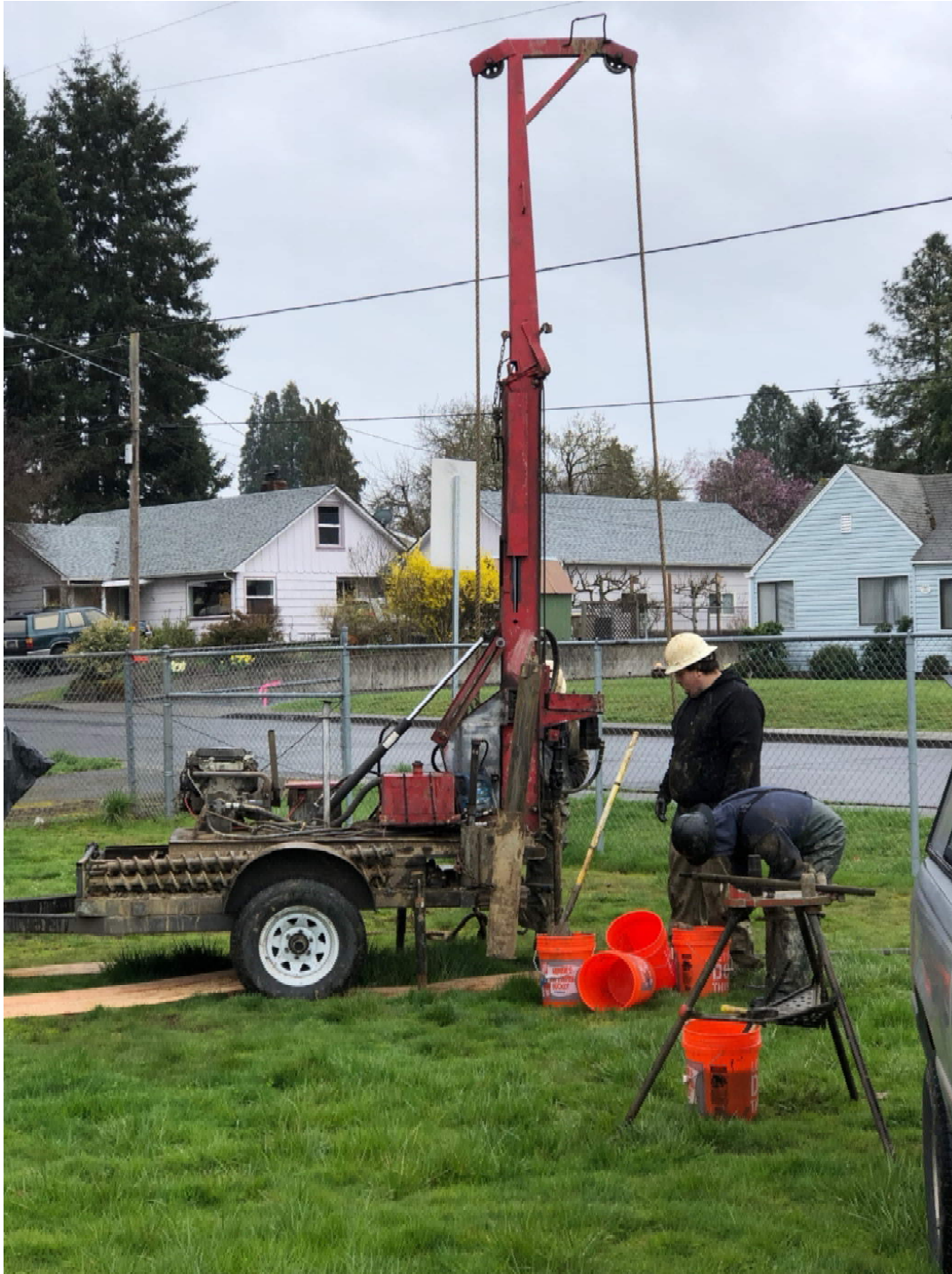
Drilling for the geotechnical survey
