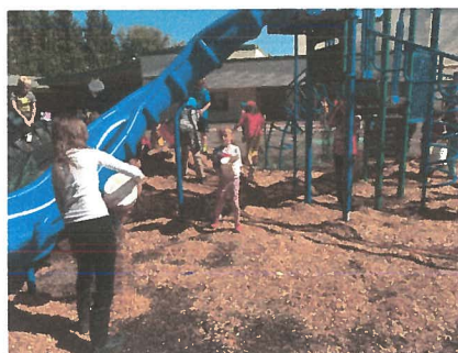
Students helping finish the slide installation.
