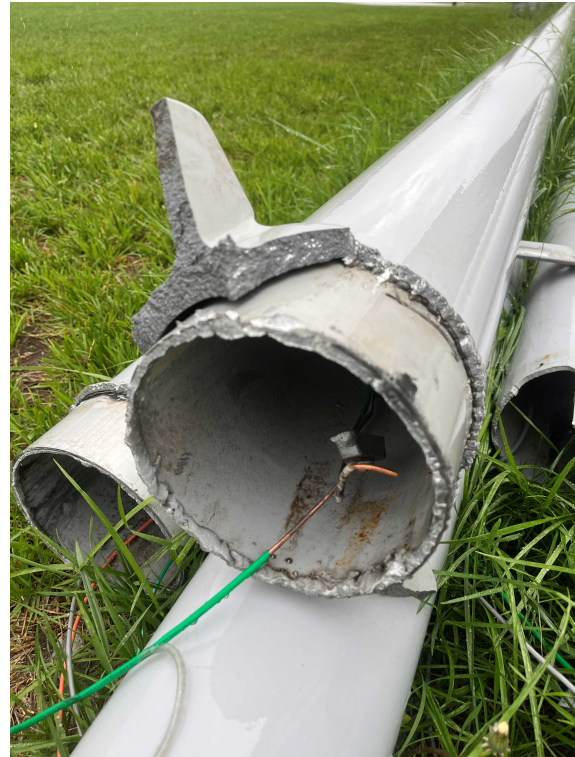
Failed light pole bases and base castings
