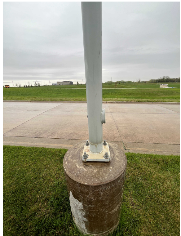
Reinstalled light pole with new base plate
