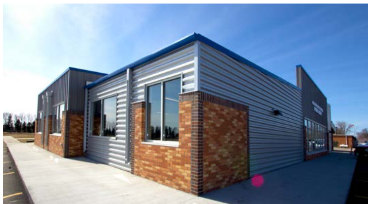
Fitness Addition Exterior
