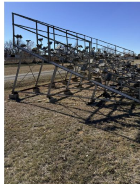
General condition of bleachers located at the JR High Campus Track
