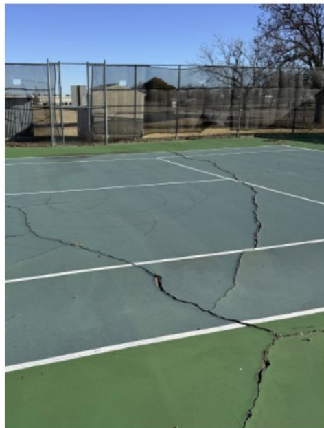
Deteriorating finishes at the Field House at Junior High
