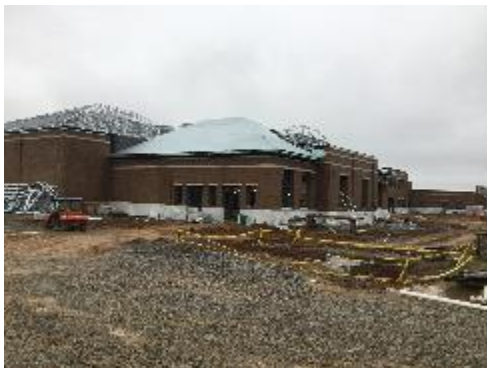
Roof decking on A has begun
