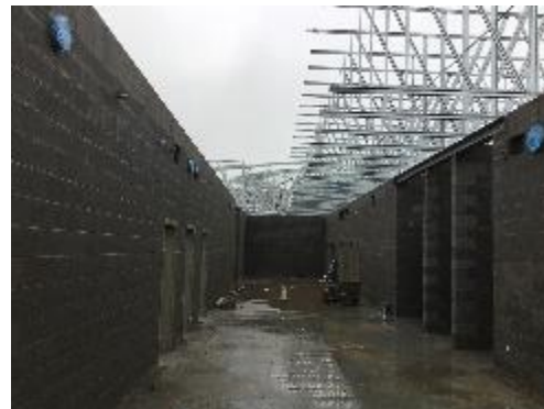
Roof trusses in A continue
