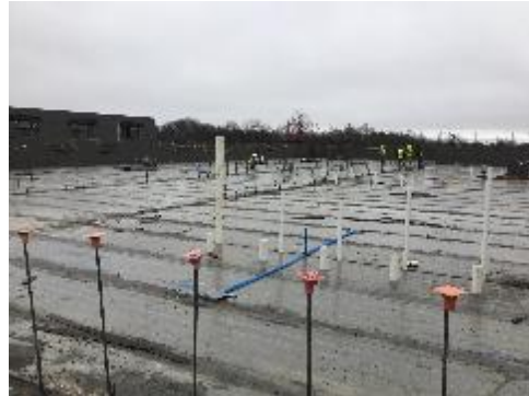
Plumbing rough-in on second floor cont.
