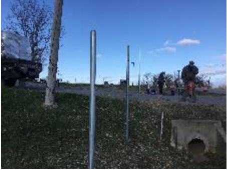
Fence poles and gate being installed
