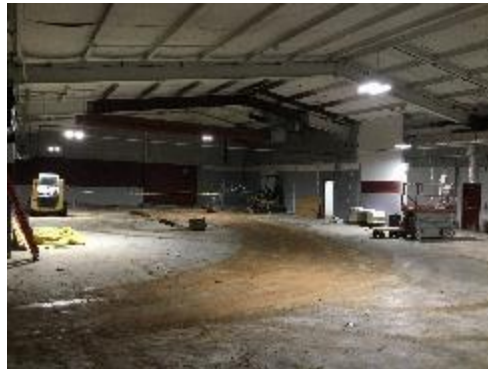
Interior demo of athletic building
