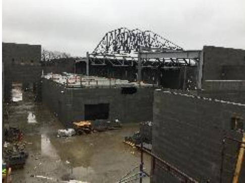
Roof trusses over the gym have begun
