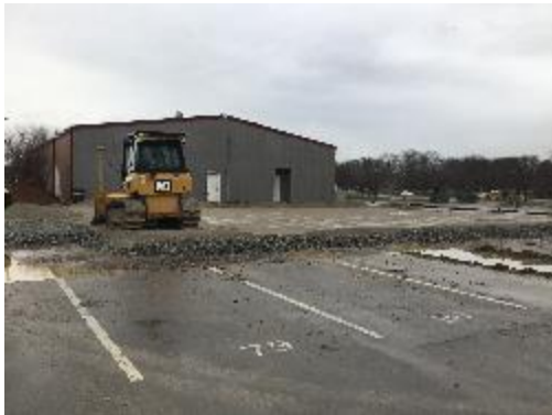
Building pad for athletic expansion
