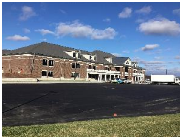
Front of Building
