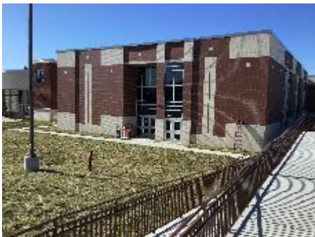
New entrance facing front parking lot
