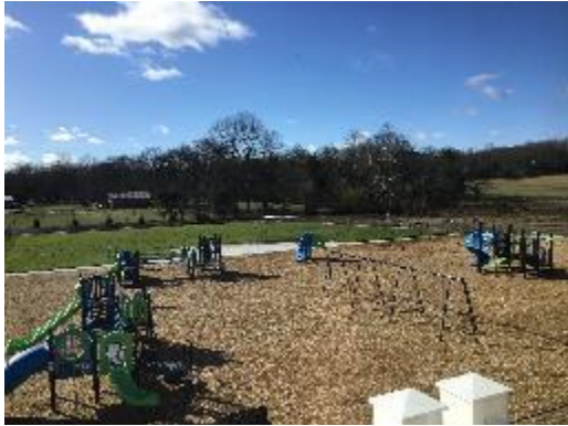
Playground equipment is installed
