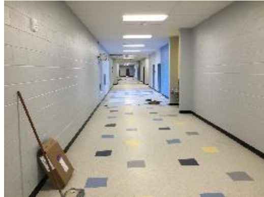
Second floor hallway ready for wax
