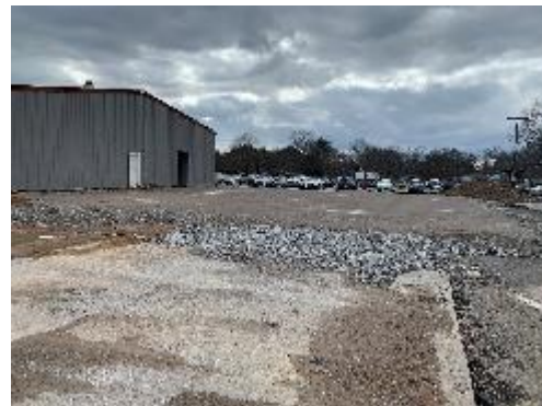
North end building pad complete
