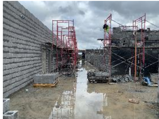
Corridor walls on second floor continue.
