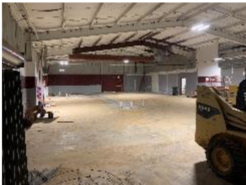
South end underground plumbing is complete
