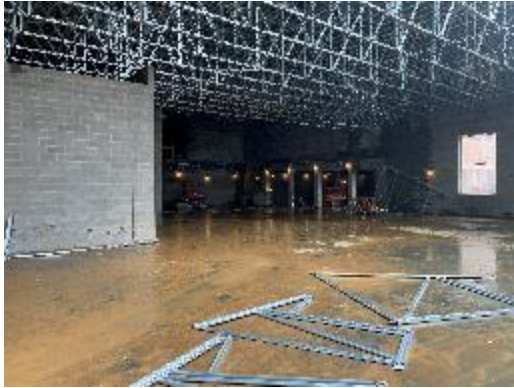
Roof decking on A has begun
