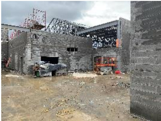
Roof trusses over the gym continue
