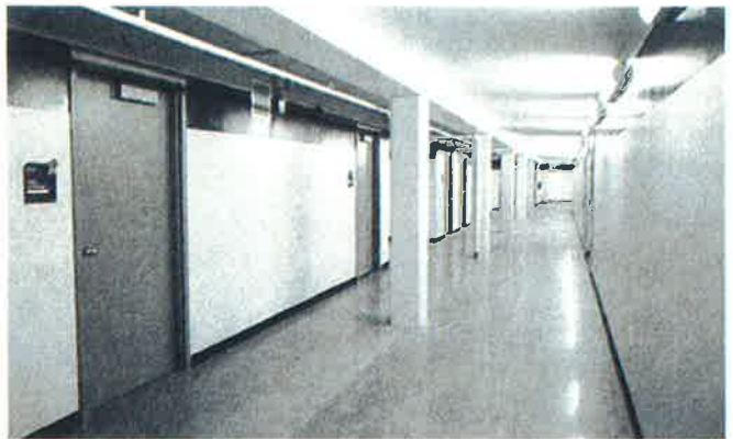
AFTER widened hallway, new lighting and paint with finished concrete
