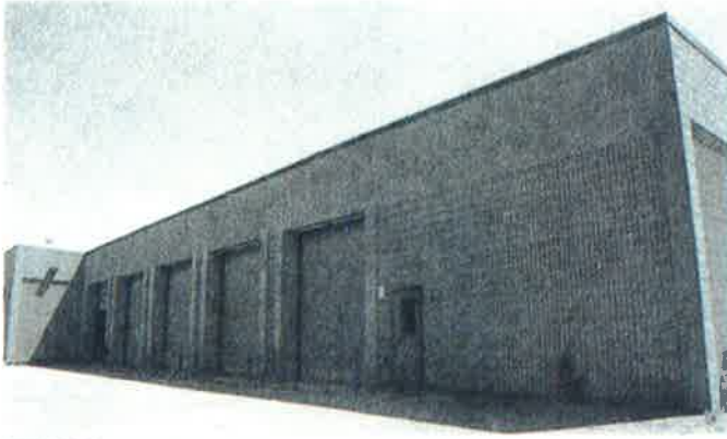
BEFORE auto classrooms
