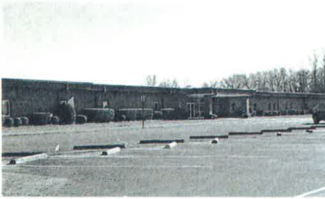
BEFORE front entrance
