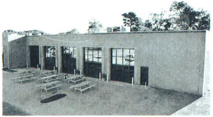
AFTER cafeteria windows
