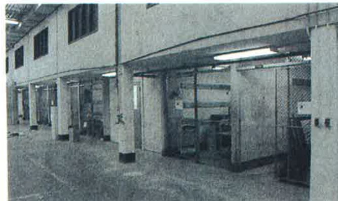
BEFORE classroom storage cages
