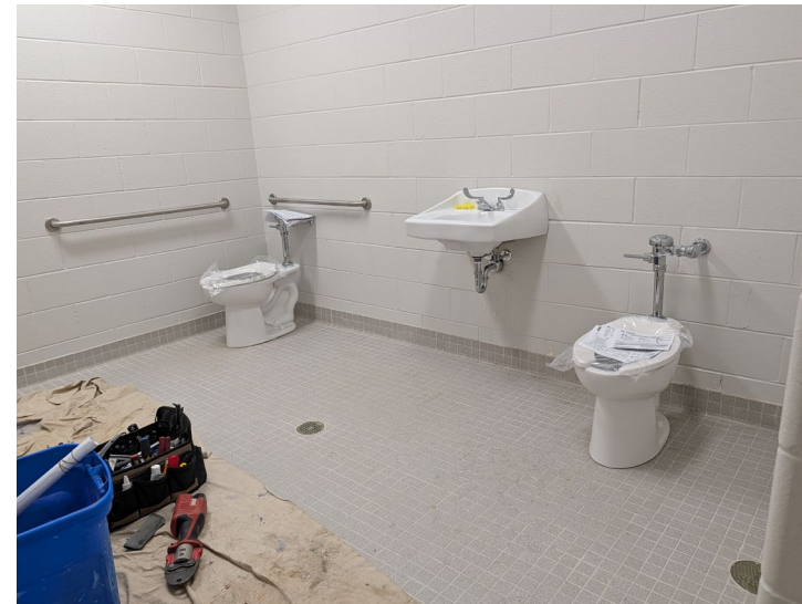
Toilet Room Renovation
