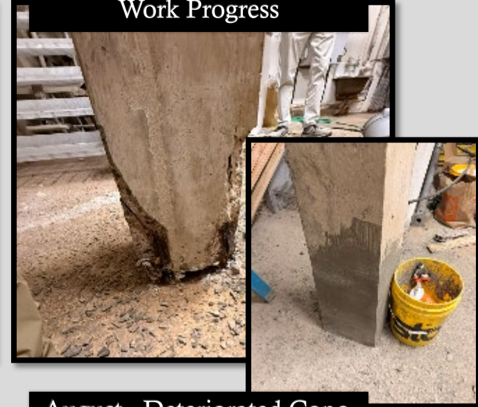
August - Deteriorated Conc. Work Progress
