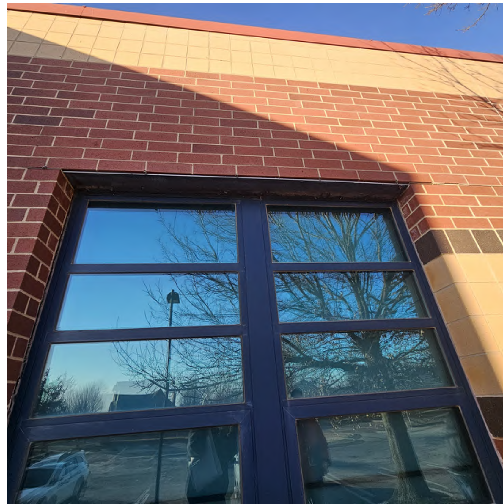
5 EXISTING TYPICAL WINDOW CONDITION G120
