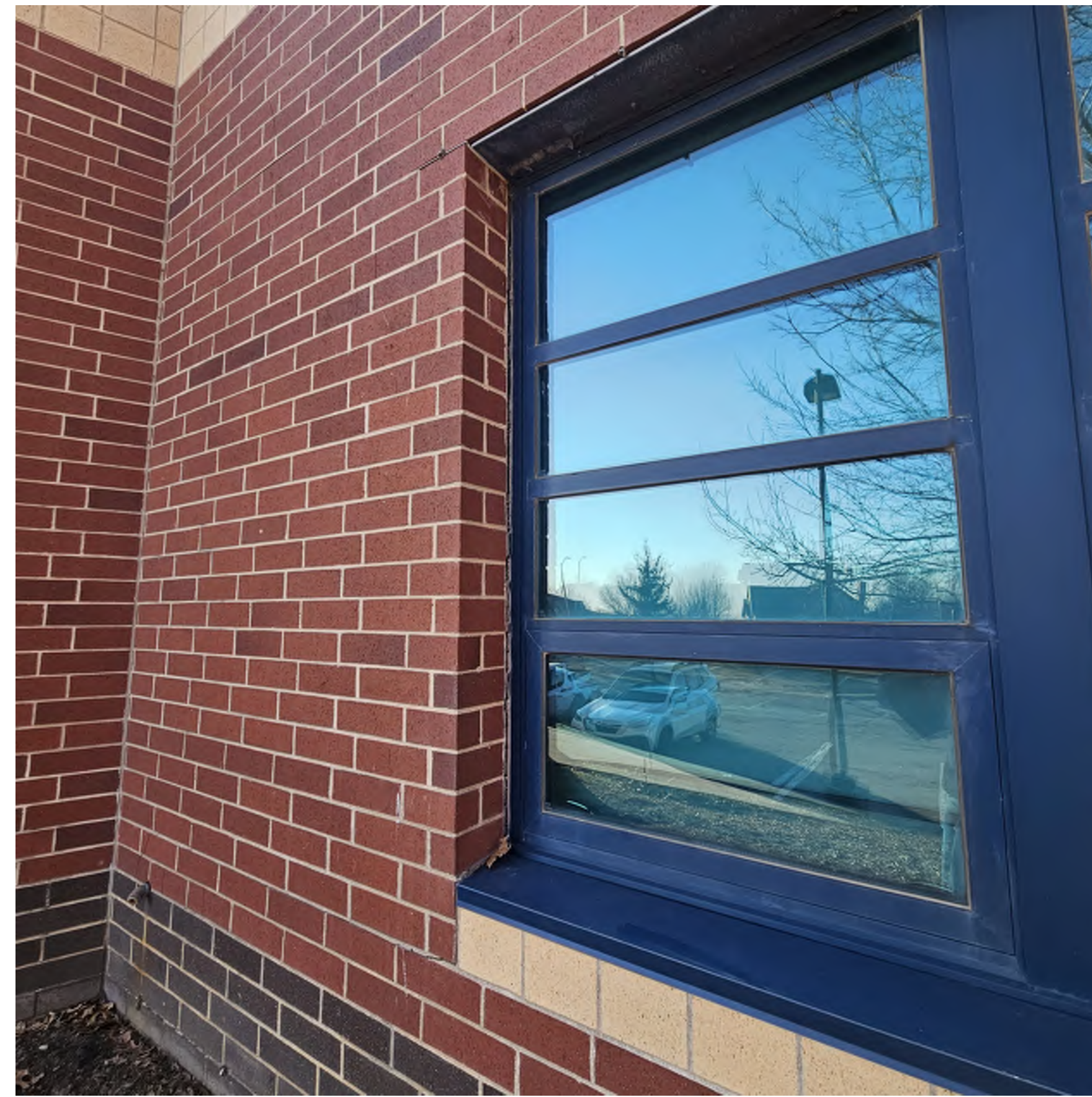
2 EXISTING TYPICAL WINDOW CONDITION G120
