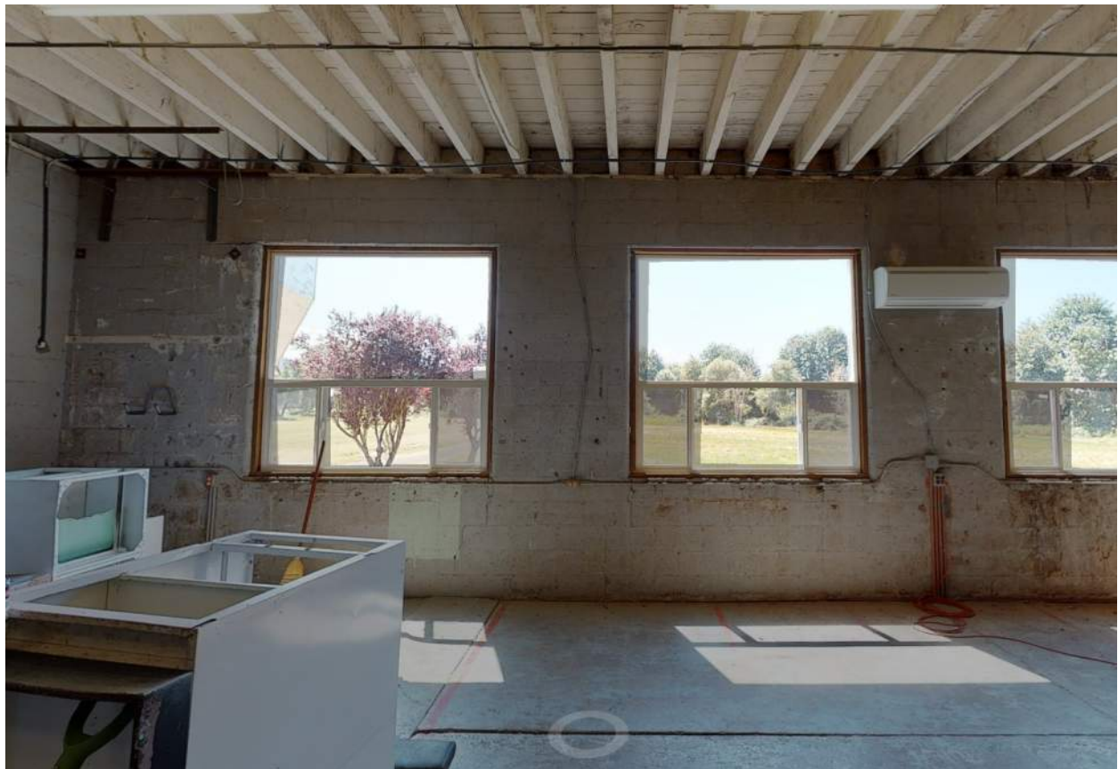
Photo 4: North Wing – Wood Shop – CMU Wall – 2x Roof Joist
