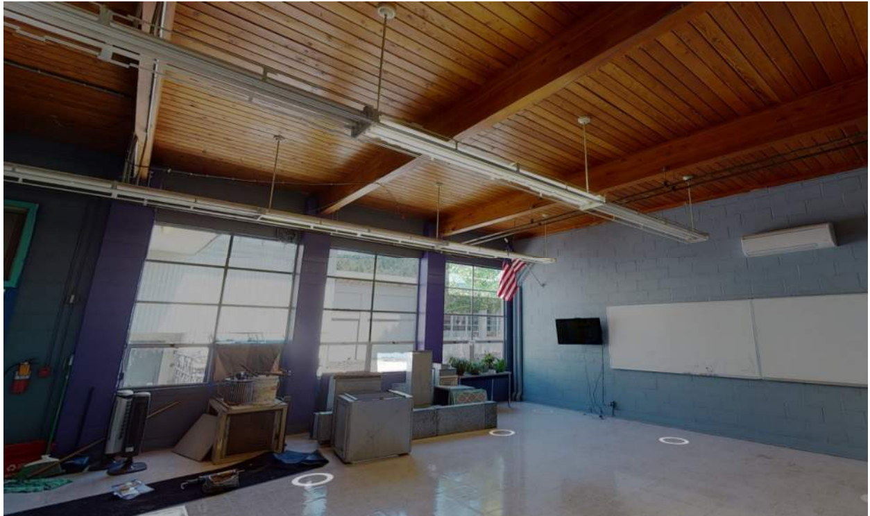
Photo 3: Northeast Corner North Wing – Wood Shop – CMU Walls, Glulam Roof Beams
