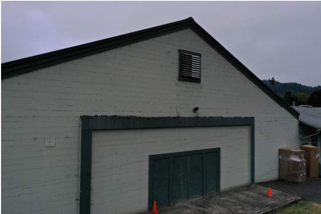
Photo 6: Exterior Gym Wall – Concrete Wall to CMU wall transition
