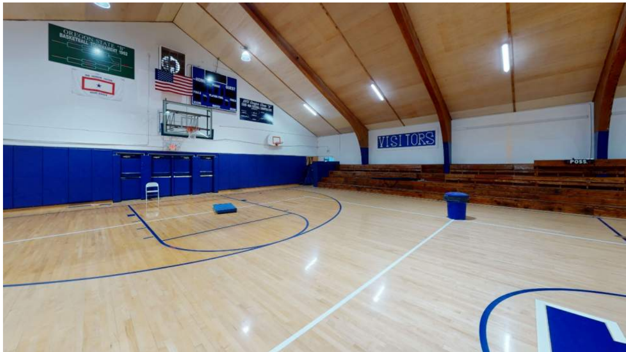
Photo 2: Northeast Corner of Gym – Tudor Arches, Concrete/CMU Walls
