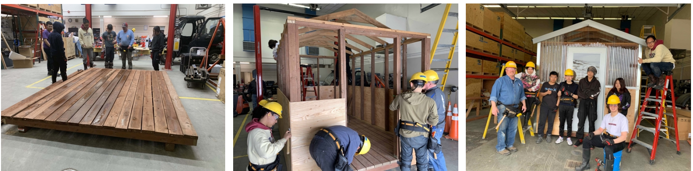
Introduction to Construction Course: Greenhouse Project Pics (April 15-26, 2024)
