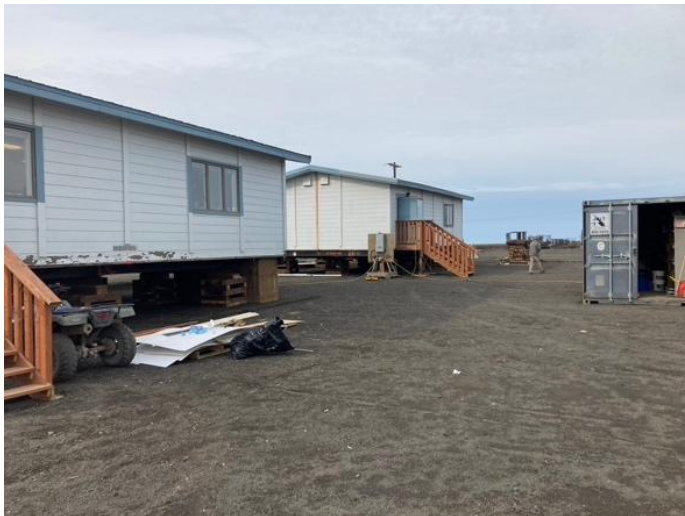
Stebbins new temporary campus under construction
