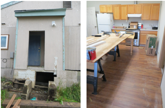
660 661 Koyuk 7-plex renovation under construction
