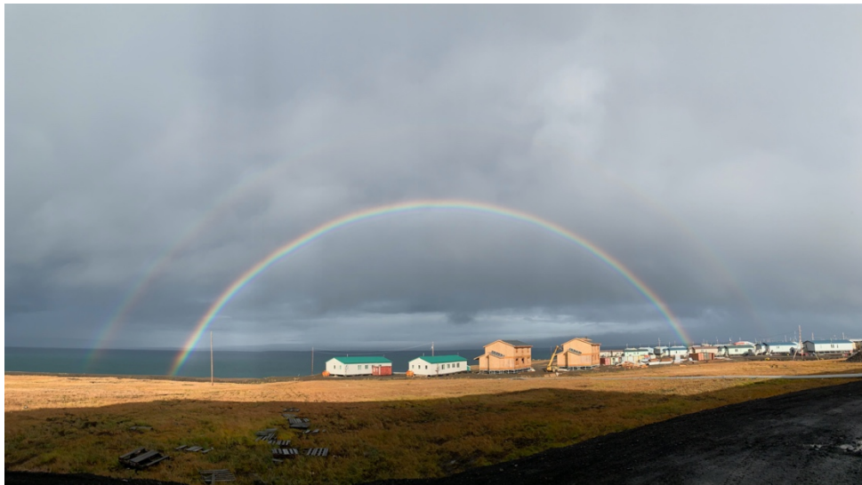
The 2-tan buildings are the Savoonga triplexes under construction
