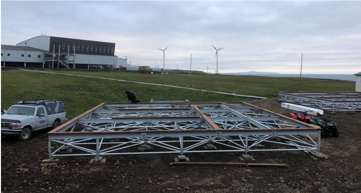
684 685 Triplex foundations under construction, Savoonga
