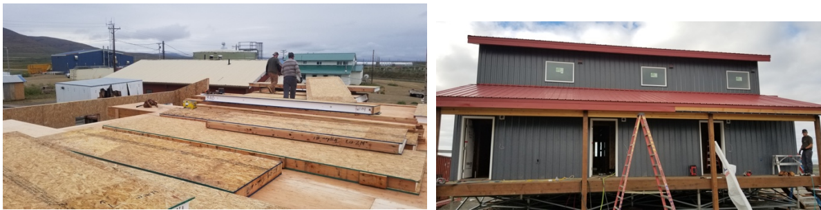
Brevig Mission triplex construction
