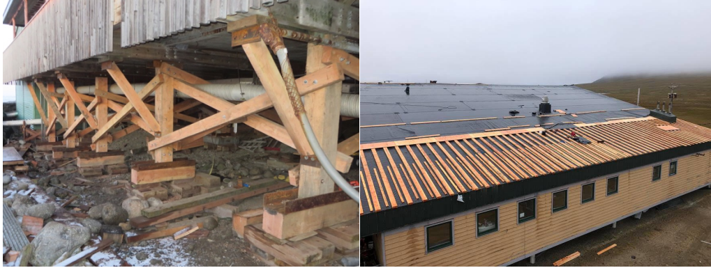
Diomedea Elementary building foundation repair, Wales roofing project
