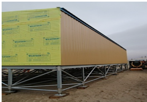
Wales Vocational/Tech Ed shop under construction
