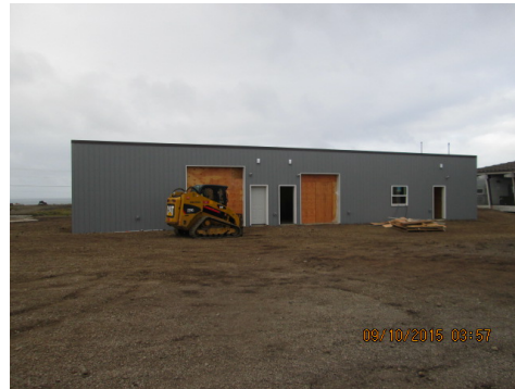
Savoonga school shop under construction
