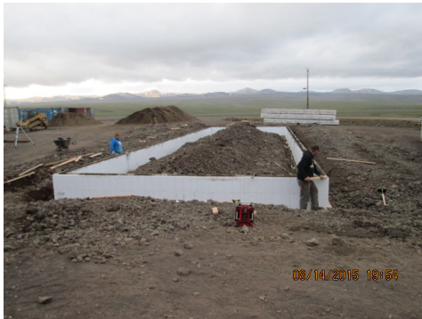
Breaking ground Savoonga school shop
