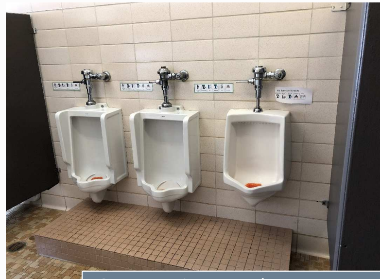
Opportunity to update restrooms, improve plumbing efficiency and provide ADA compliance
