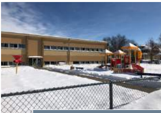
The playground is not ADA accessible and lacks sun shading structures
