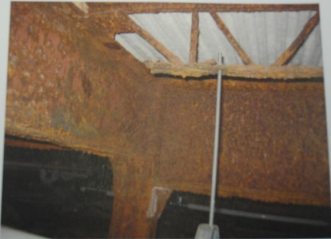
Photo No. 30. Girder/Column connection, Grid 7.
