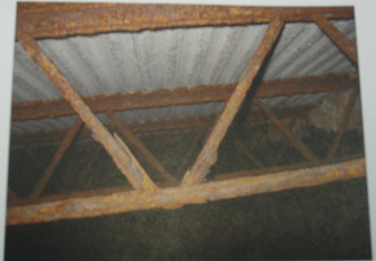
Photo No. 16. Joist, Grid 4.
