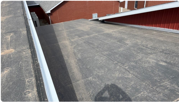
Photo showing additional overview of Area 04 roof.
