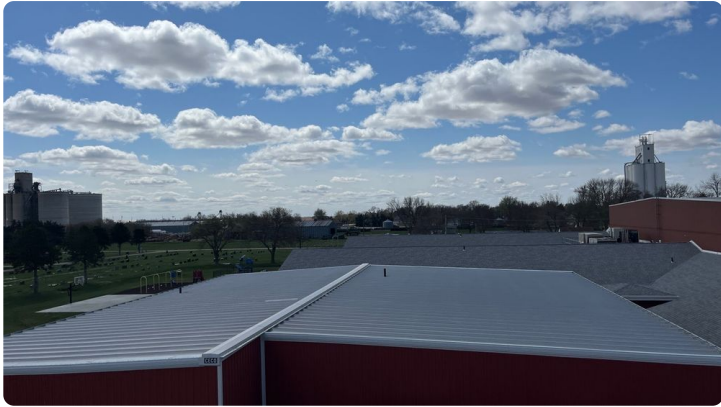
Photo showing overview of Area 17 roof.
