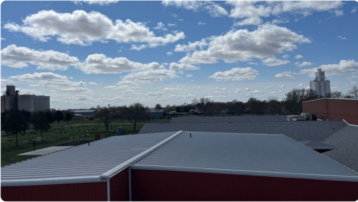
Photo showing overview of Area 17 roof.
