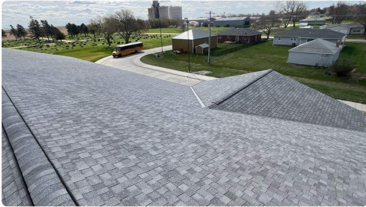
Photo showing overview of Area 01 roof.
