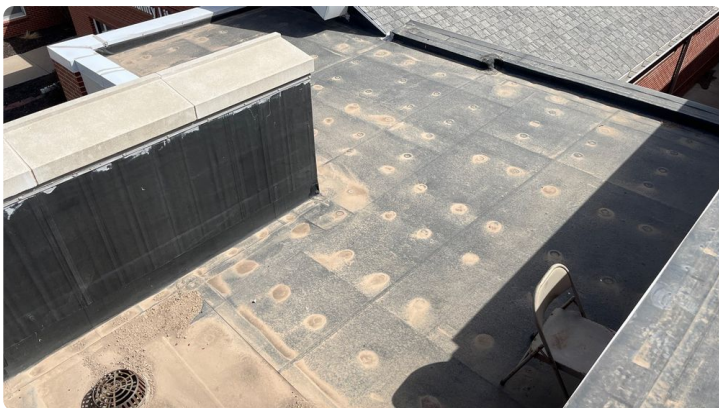
Photo showing additional overview of area 05 roof.
