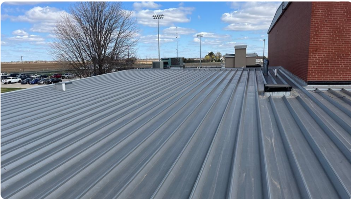
Photo showing additional overview of Area 08 roof.
