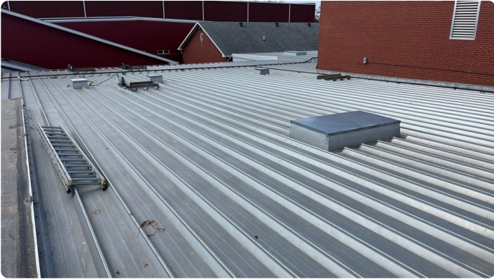
Photo showing overview of Area 13 roof.
