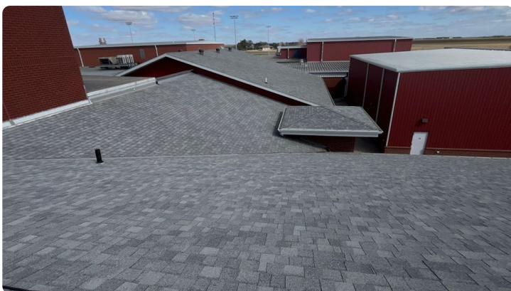
Photo showing additional overview of Area 01 roof.
