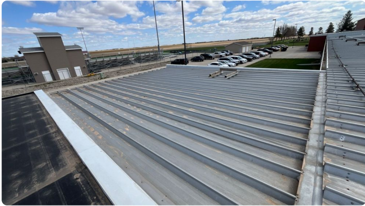
Photo showing overview of Area 11 roof.
