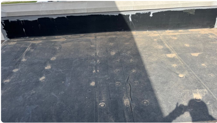
Photo showing overview of Area 05 roof.
