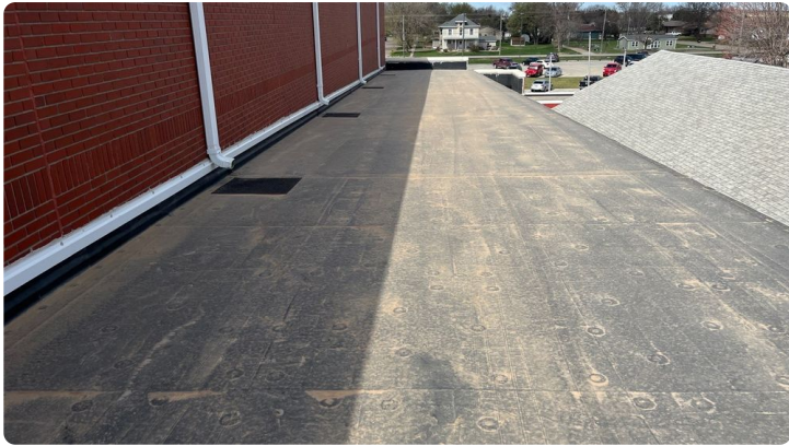
Photo showing additional overview of Area 04 roof.
