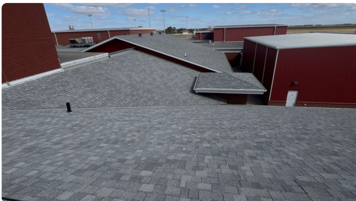
Photo showing additional overview of Area 01 roof.
