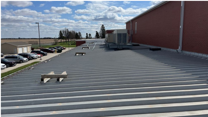
Photo showing additional overview of Area 09 roof.
