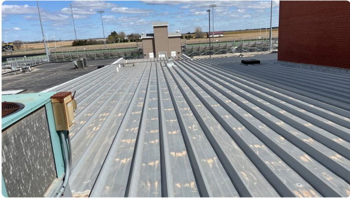
Photo showing overview of Area 09 roof.
