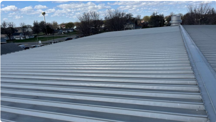
Photo showing additional overview of Area 16 roof.
