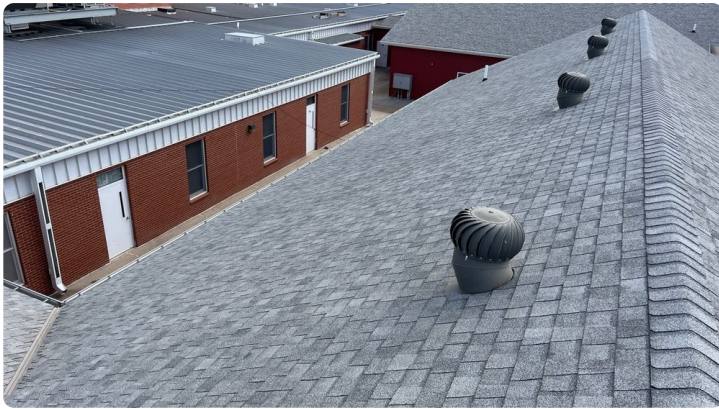
Photo showing overview of Area 07 roof.
