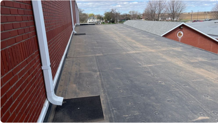
Photo showing overview of Area 04 roof.
