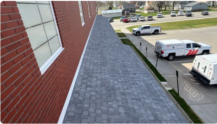
Photo showing overview of Area 06 roof.
