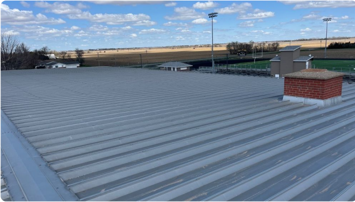
Photo showing overview of Area 16 roof.
