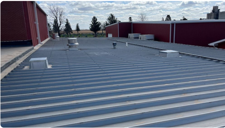
Photo showing additional overview of Area 13 roof.
