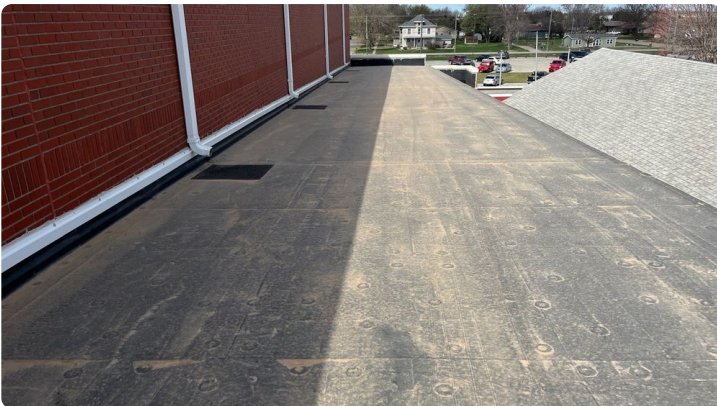
Photo showing additional overview of Area 04 roof.
