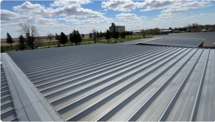
Photo showing overview of Area 15 roof.
