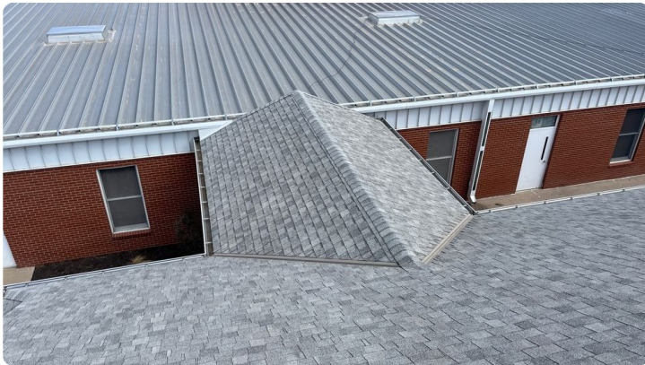
Photo showing additional overview of area 07 roof.
