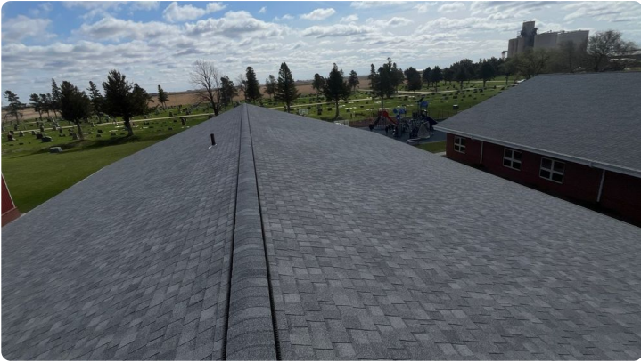
Photo showing additional overview of Area 01 roof.
