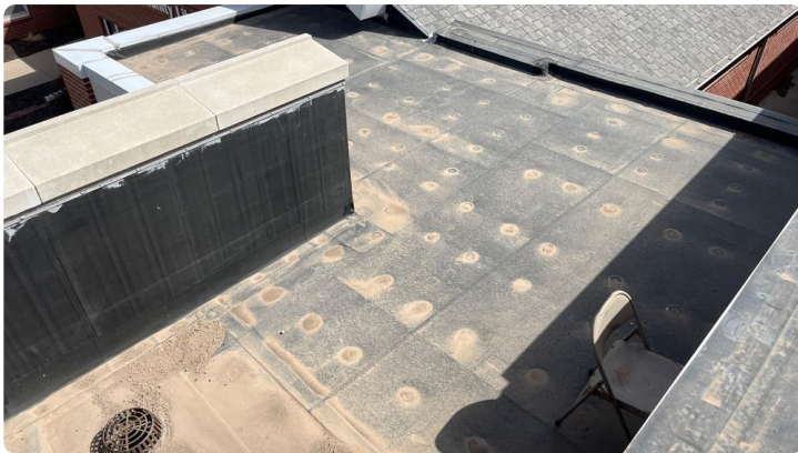
Photo showing additional overview of area 05 roof.
