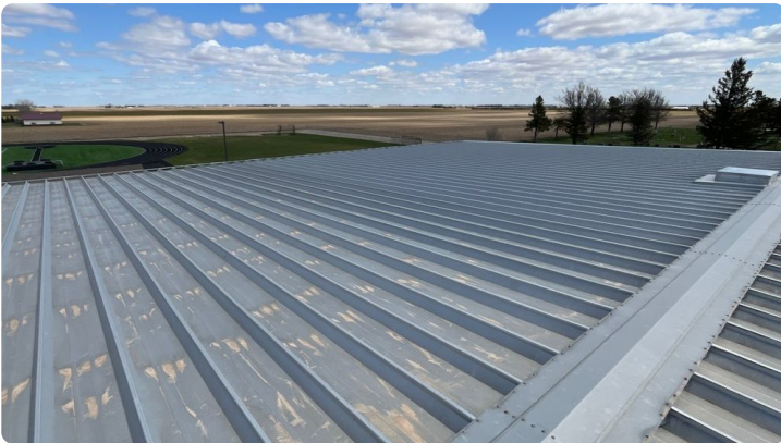
Photo showing additional overview of Area 15 roof.
