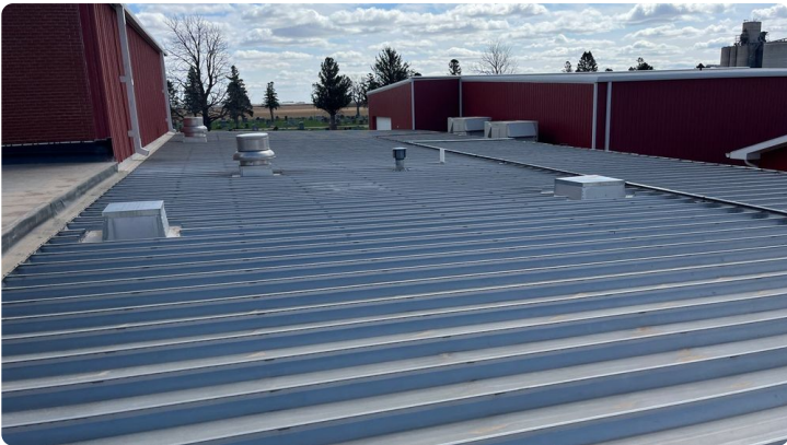
Photo showing additional overview of Area 13 roof.
