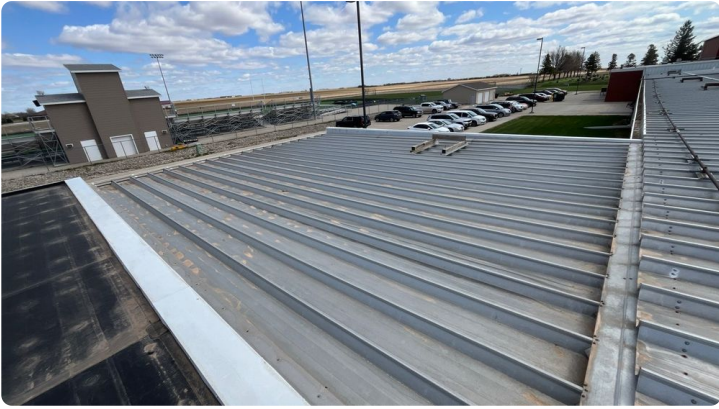
Photo showing overview of Area 11 roof.
