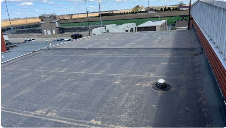
Photo showing overview Area 14 roof.
