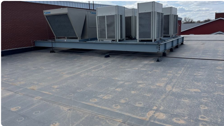
Photo showing additional overview of Area 12 roof.
