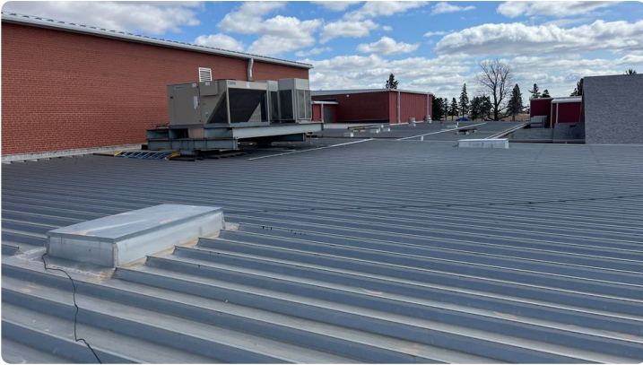
Photo showing overview of Area 08 roof.
