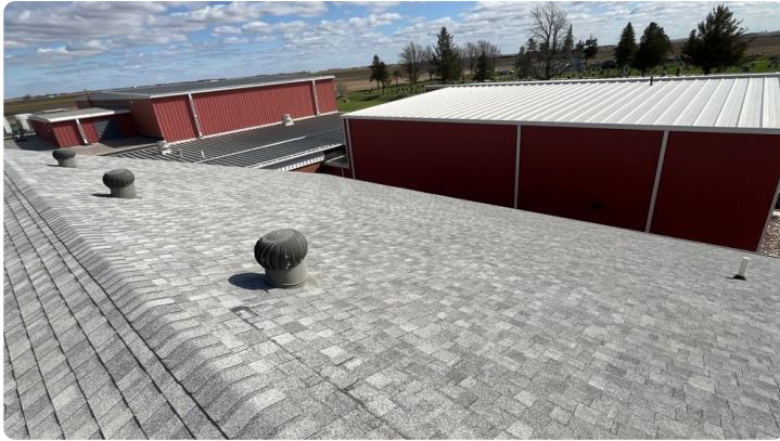
Photo showing overview of Area 03 roof.
