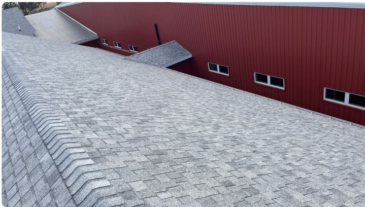
Photo showing additional overview of Area 07 roof.
