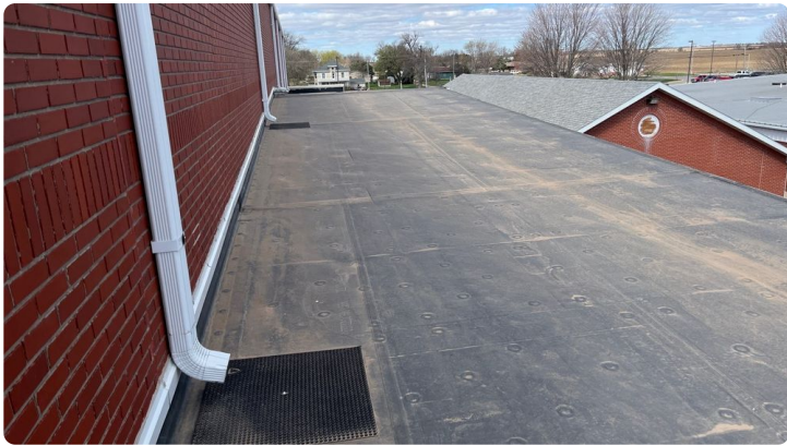
Photo showing overview of Area 04 roof.
