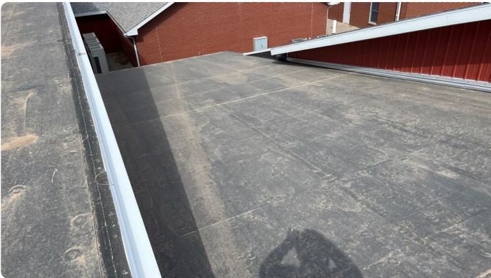
Photo showing additional overview of Area 04 roof.
