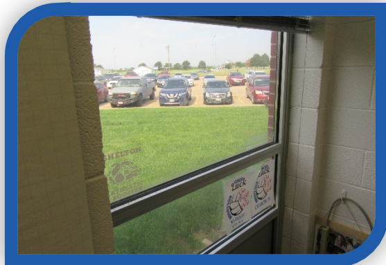
Original Window System
