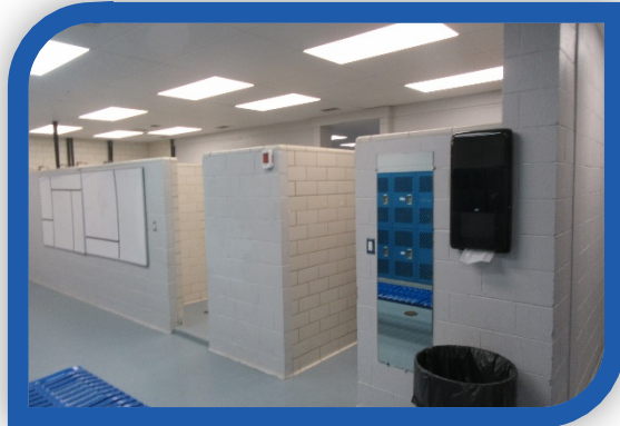
Remodeled Locker Room
