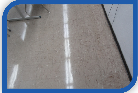
9" x 9" Asbestos Tiles
