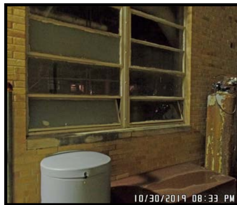
Windows open boiler area High School
