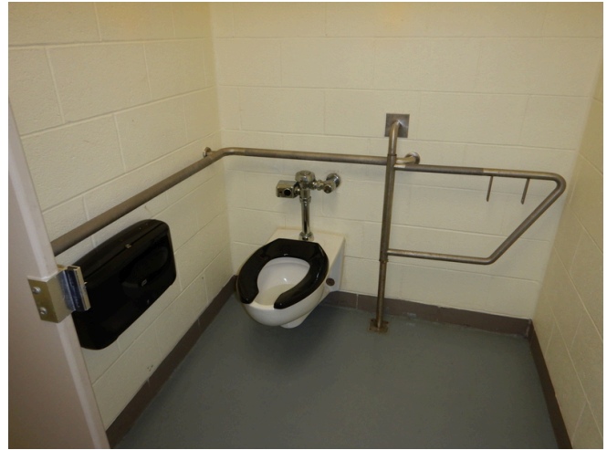
Boys locker room toilet.
