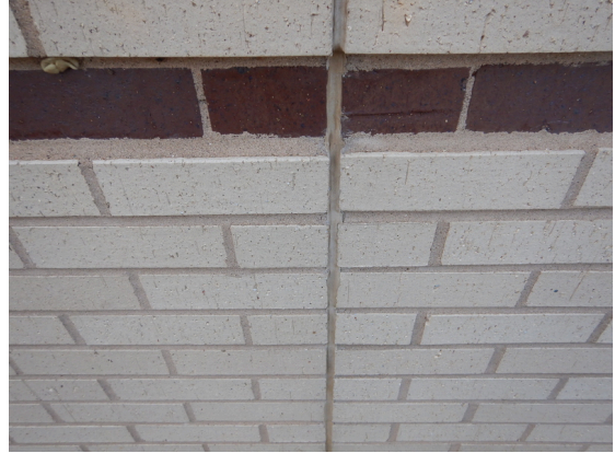
Photo 38: Elastomeric sealant.
