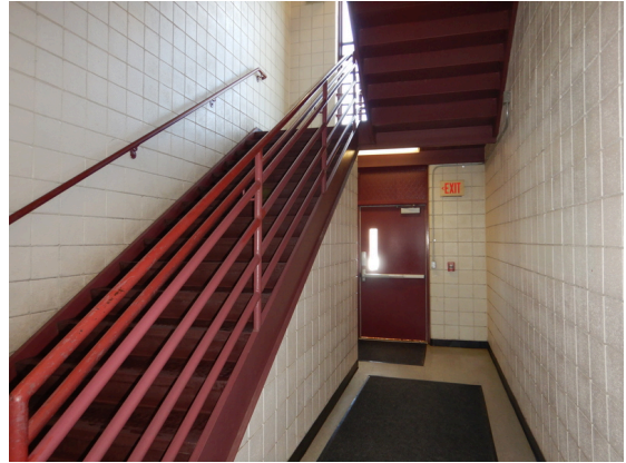
Photo 116: Typical egress stairway.
