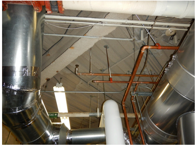
Metal roof deck.
