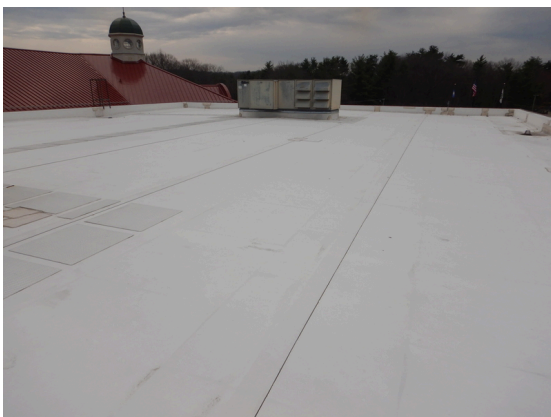
Photo 65: Gym: Roof overview facing southeast.
