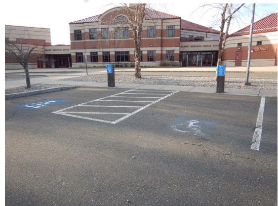
Photo 192: Accessible parking at the front elevation of the building.
