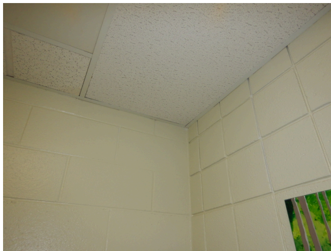
Typical 1st floor restroom wall and ceiling finishes.
