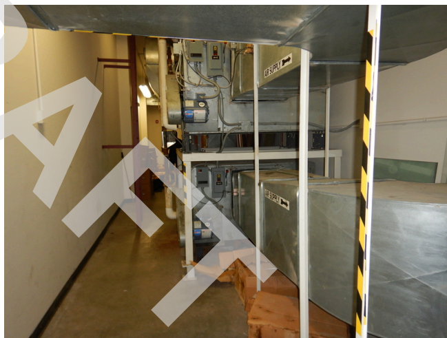
Second floor mechanical room.
