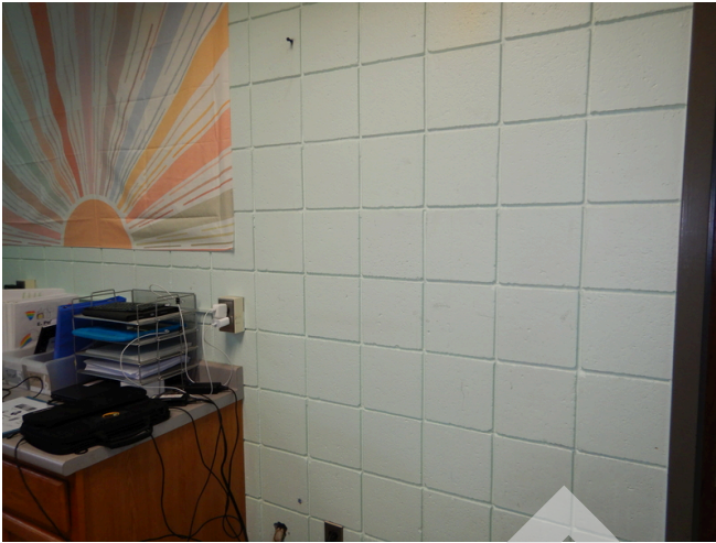
Typical painted CMU wall finish.
