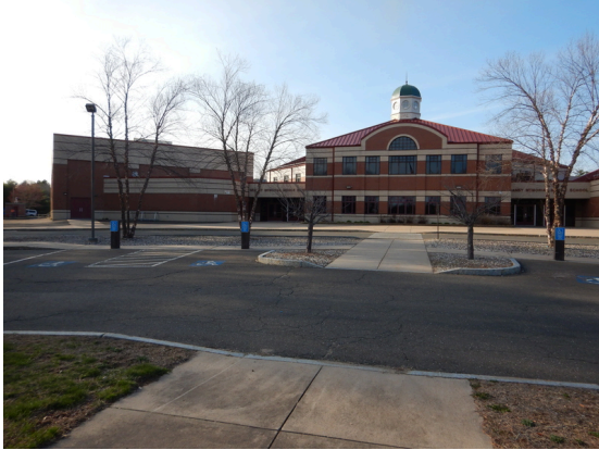
Photo 31: South (front) elevation of the building.
