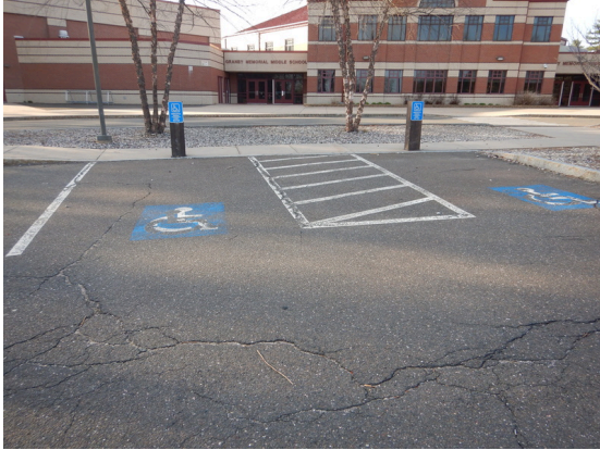
Photo 193: Accessible parking at the front elevation of the building.
