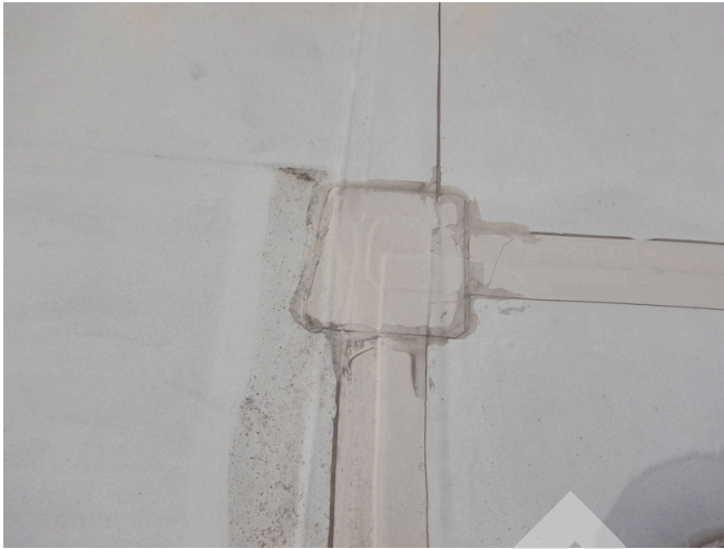
TPO membrane patch.
