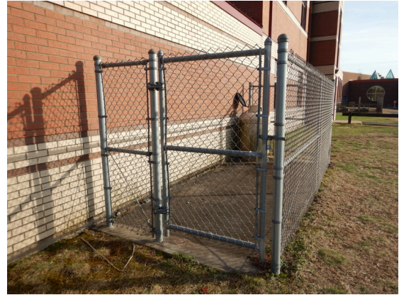
Photo 2: Chain link fence surrounding propane tank at the loading dock area.
