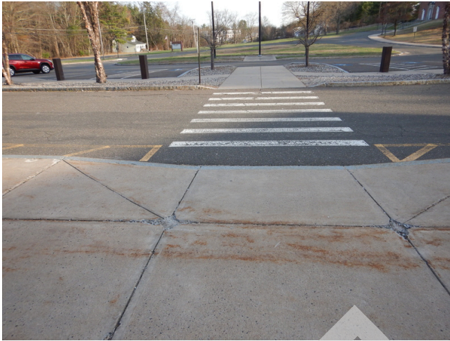
Route to an accessible building entrance.
