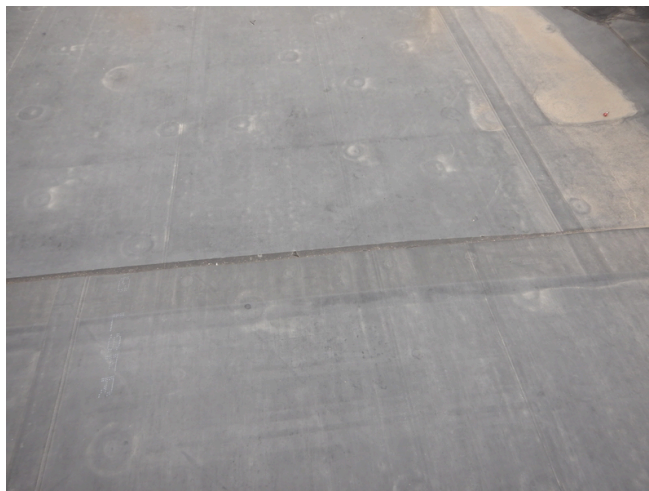
Close up of EPDM roof membrane.
