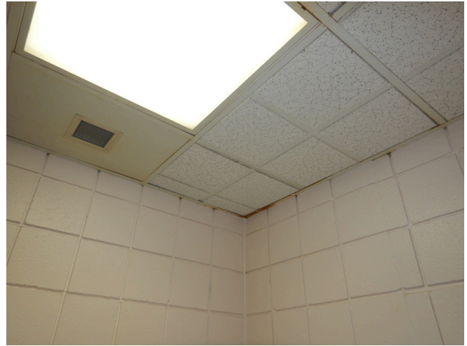
Clinic restroom wall and ceiling finishes.
