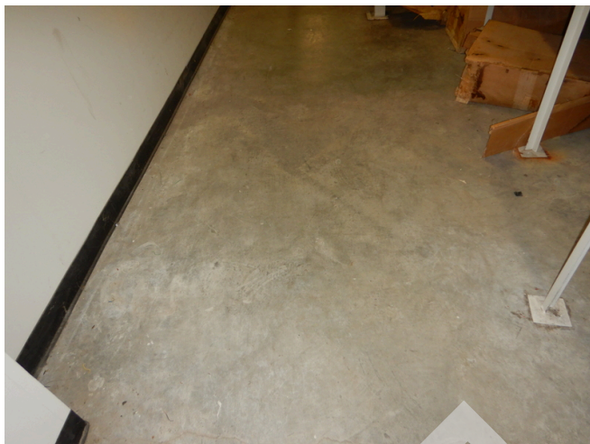
Concrete slab-on-grade.
