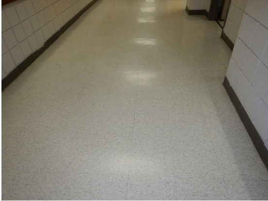
Photo 121: Technology wing corridor floor finish.
