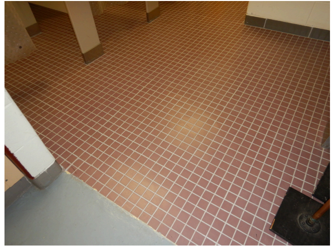
Locker room shower flooring.
