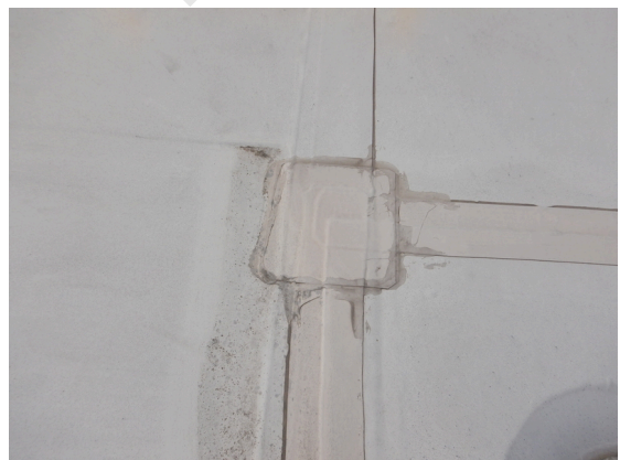
Photo 66: TPO membrane patch.
