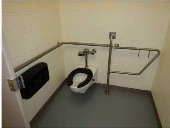
Photo 91: Boys locker room toilet.
