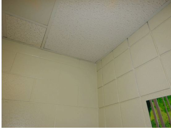
Photo 103: Typical 1st floor restroom wall and ceiling finishes.
