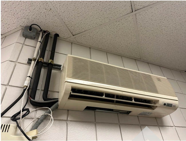
DX mini-split fan coil unit.
