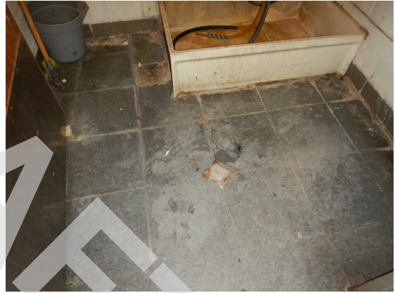
Photo 100: Custodian room. VCT flooring.
