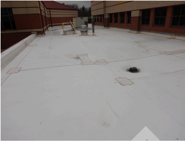
Gym: Lower roof overview.
