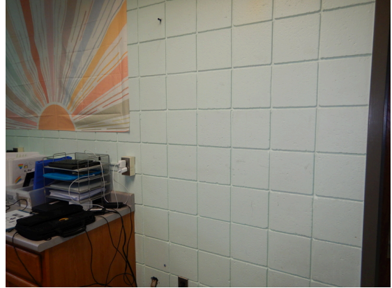
Photo 98: Typical painted CMU wall finish.
