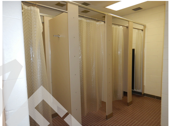
Photo 94: Girls locker room showers.
