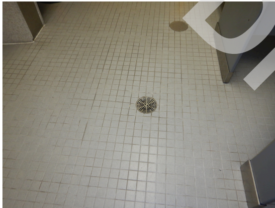
Photo 105: Typical 1st floor restroom flooring.
