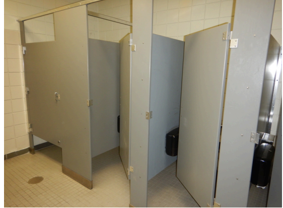
Photo 104: Typical 1st floor restroom toilet partitions.
