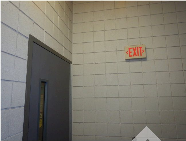
Painted CMU wall finishes.
