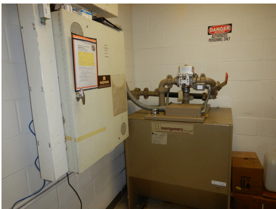
Photo 131: Elevator equipment room.
