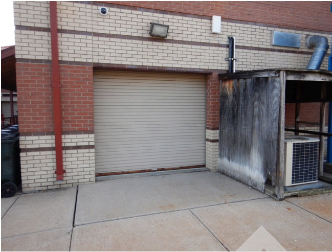
Drive-in loading dock door.
