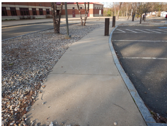
Photo 11: Concrete walkway at the front of the building.
