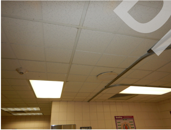
Photo 135: Clinic ceiling finishes.
