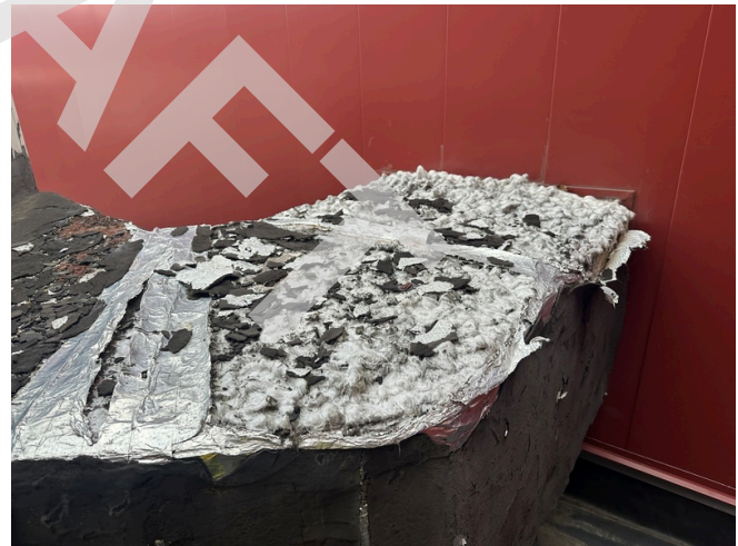
Typical condition of exterior ductwork.
