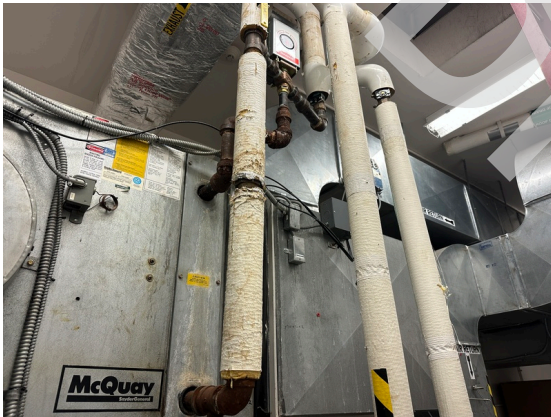
Photo 171: Typical condition of HHW piping, connections, and insulation.
