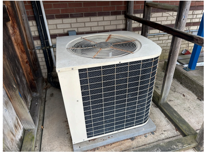
DX split-system condensing unit.
