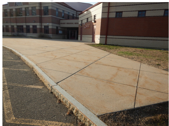
Photo 12: Concrete walkway at the main entrance to the building.
