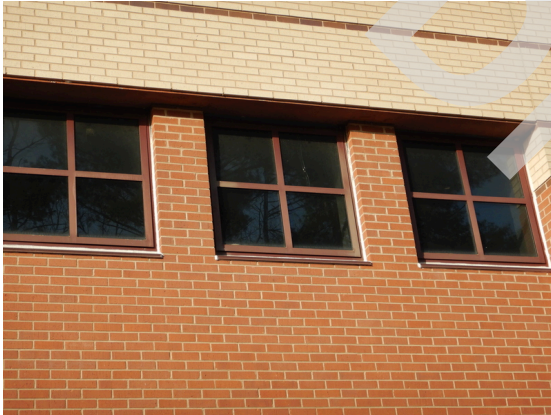
Photo 39: Upper level windows.
