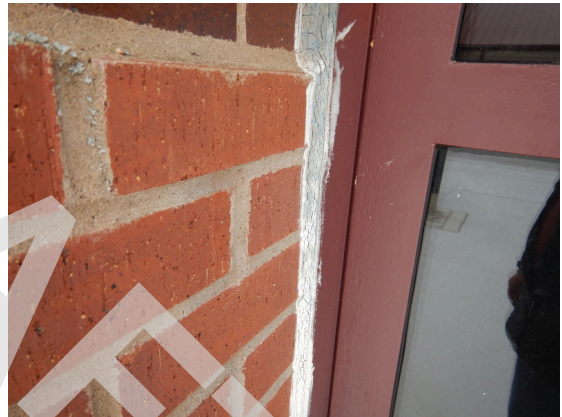
Photo 46: View of elastomeric sealant around the door.
