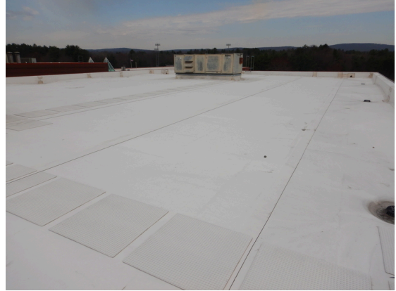
Photo 62: Gym: Roof overview facing northwest.
