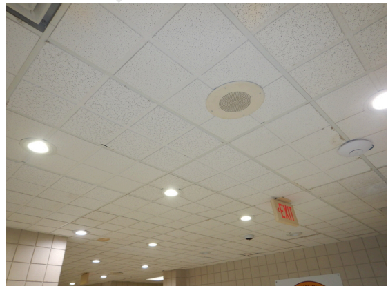
Photo 78: Acoustical ceiling finish.
