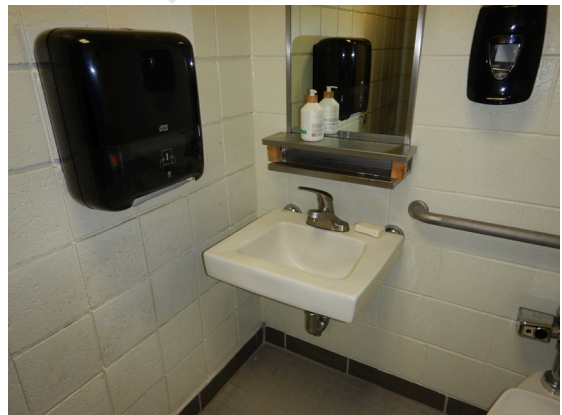
Photo 102: Typical 1st floor restroom sink.
