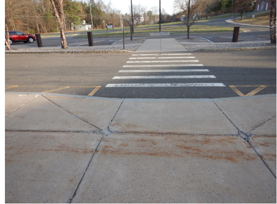
Photo 194: Route to an accessible building entrance.
