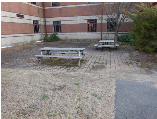
Photo 17: Outdoor rest area at the rear of the building.
