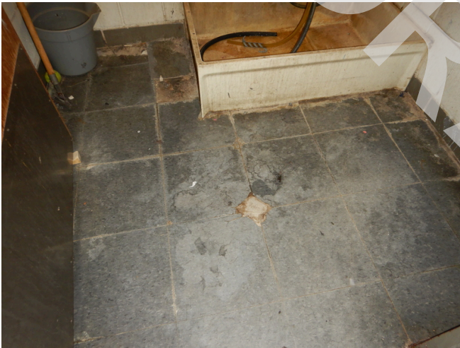
Custodian room. VCT flooring.
