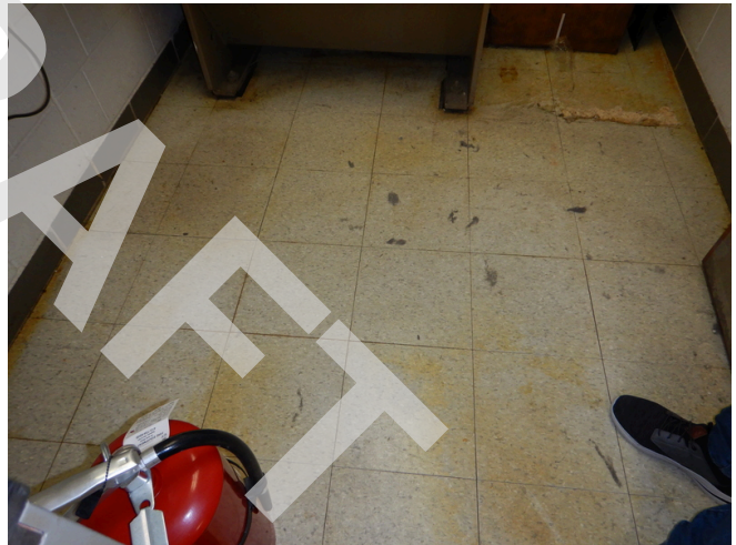
Elevator equipment room flooring.
