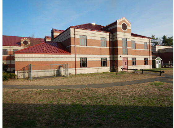
Photo 32: Partial west elevation of the building.
