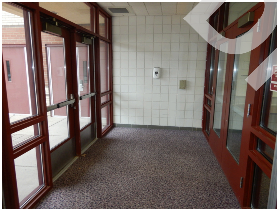
Photo 195: Accessible entrance doors in a series.
