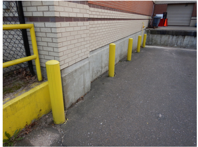
Painted plastic covered bollards located adjacent to the loading dock.
