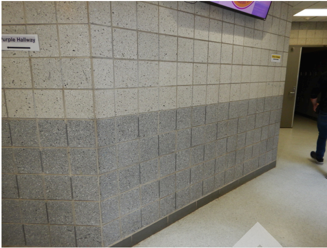
Upper level corridor wall finishes.
