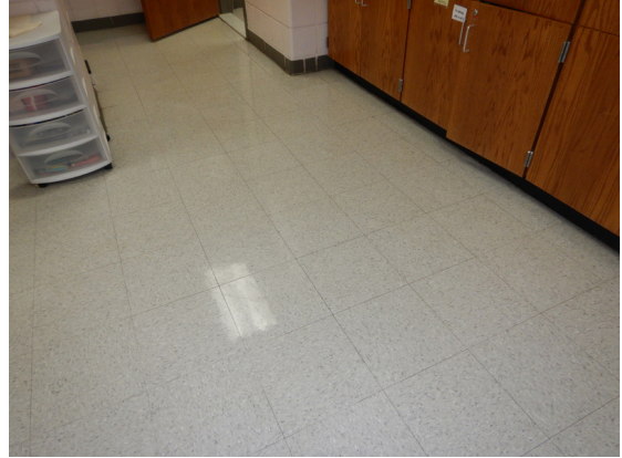
Photo 134: Clinic flooring finish.
