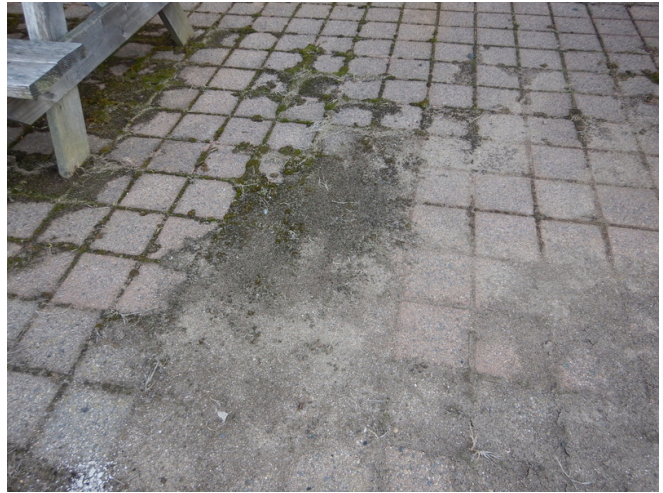
Brick pavers at the outdoor rest area.
