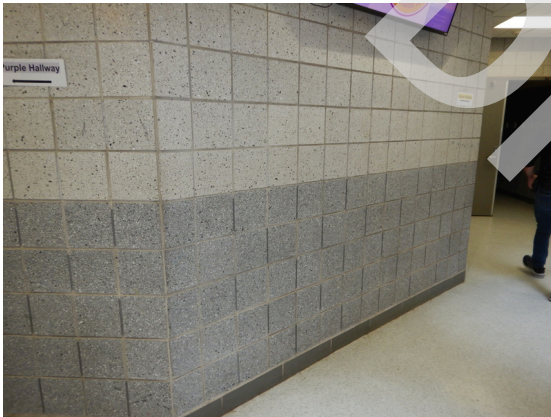
Photo 141: Upper level corridor wall finishes.
