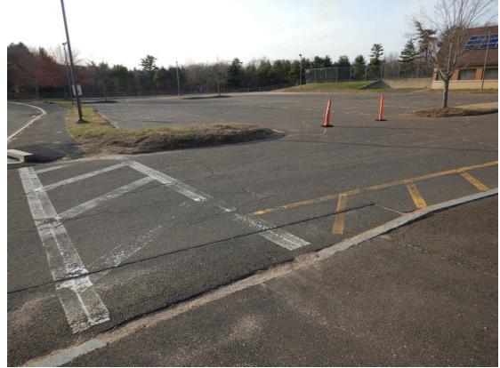
Photo 14: Overview of the main parking lot at the rear of the building.
