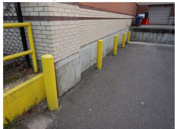
Photo 6: Painted plastic covered bollards located adjacent to the loading dock.
