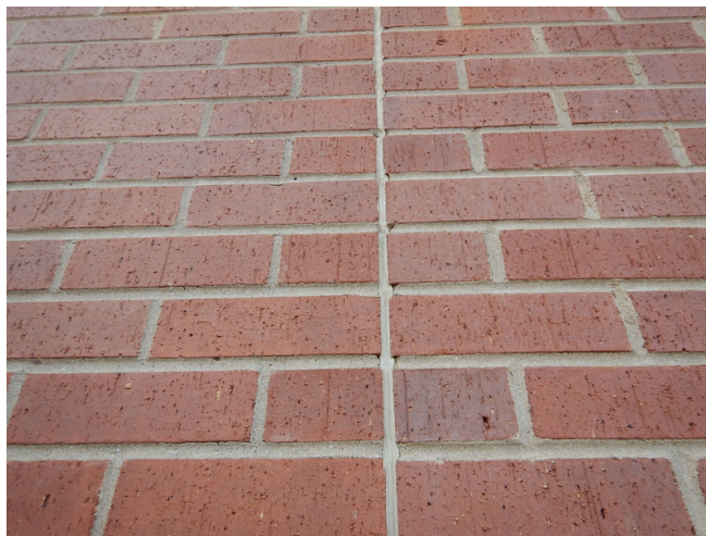
Elastomeric sealant.
