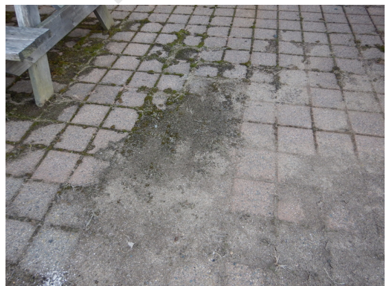
Photo 18: Brick pavers at the outdoor rest area.
