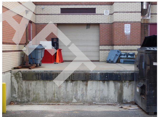
Loading dock steel overhead door.
