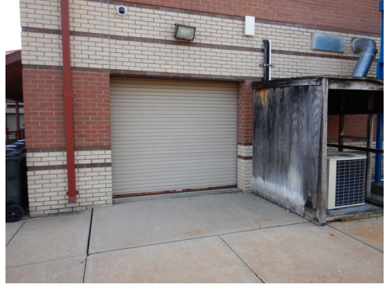
Photo 44: Drive-in loading dock door.
