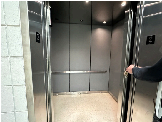
Photo 185: Elevator cab interior.
