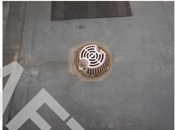
Photo 52: Internal drain.
