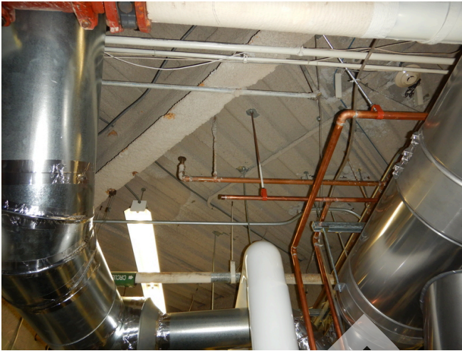
Metal roof deck.
