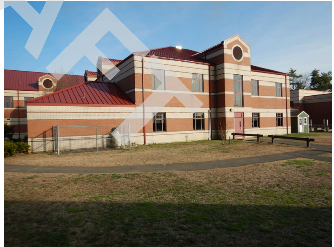
Partial west elevation of the building.
