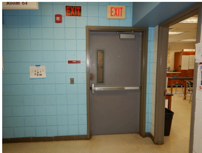
Emergency exit door leading to the egress stairway.
