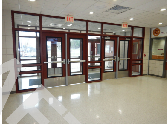
Photo 76: Main entrance lobby.
