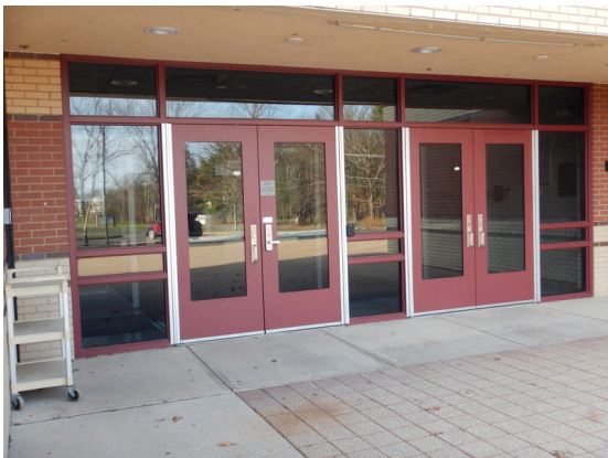
Photo 35: main entrance doors.
