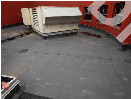
Photo 51: EDPM roof membrane over cafeteria..
