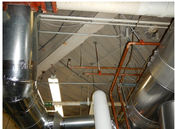
Photo 48: Metal roof deck.
