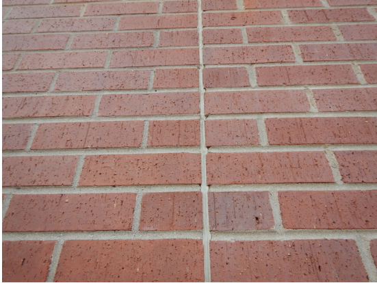
Photo 37: Elastomeric sealant.
