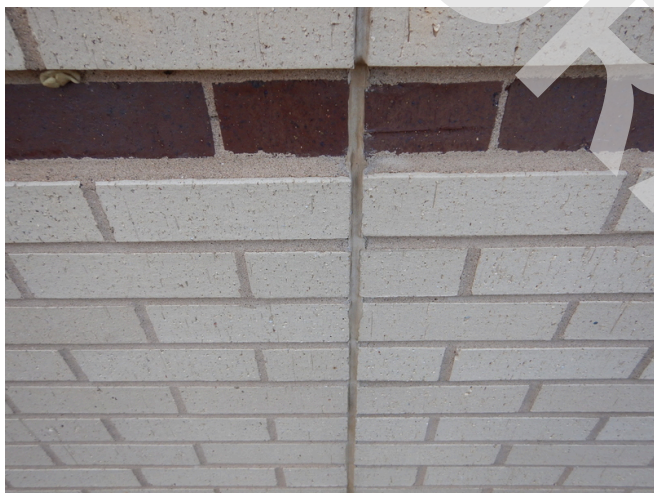
Elastomeric sealant.
