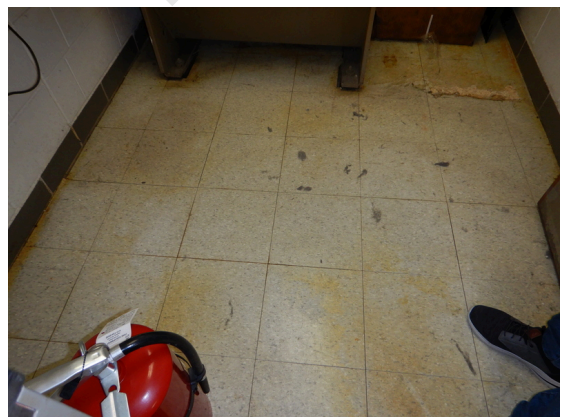
Photo 132: Elevator equipment room flooring.
