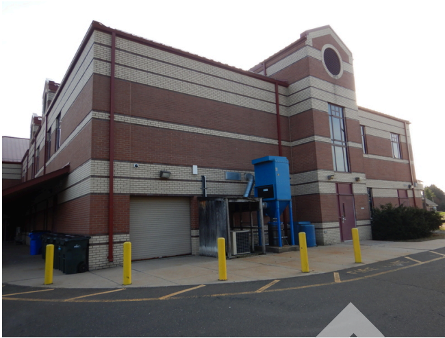
North elevation of the building.
