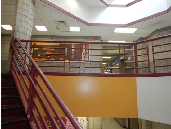
Photo 139: Monumental stairway at the center of the building.
