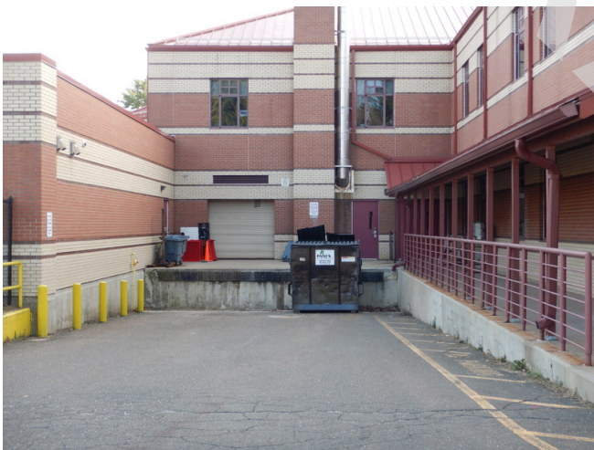
Loading dock area.
