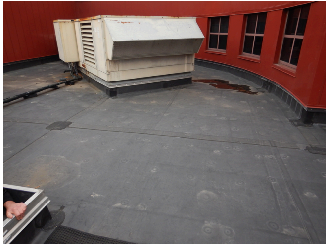
EDPM roof membrane over cafeteria..
