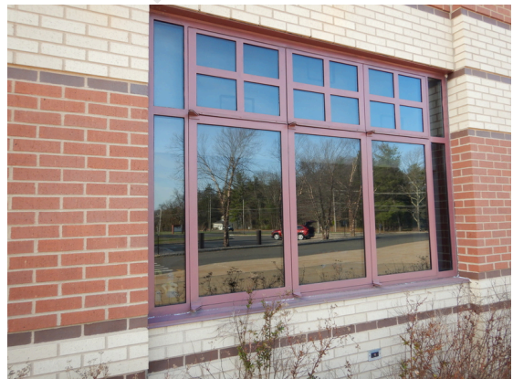
Photo 36: First floor window.
