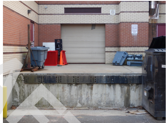
Photo 4: Loading dock steel overhead door.
