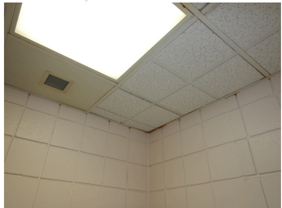
Photo 138: Clinic restroom wall and ceiling finishes.
