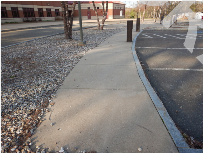
Concrete walkway at the front of the building.
