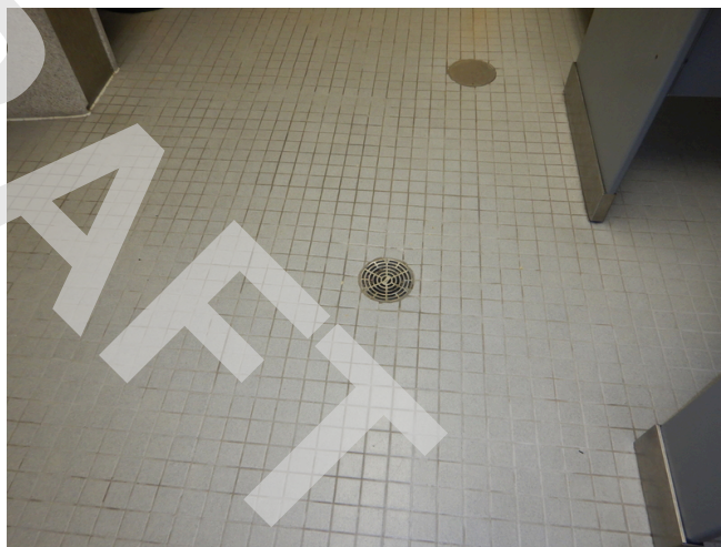
Typical 1st floor restroom flooring.
