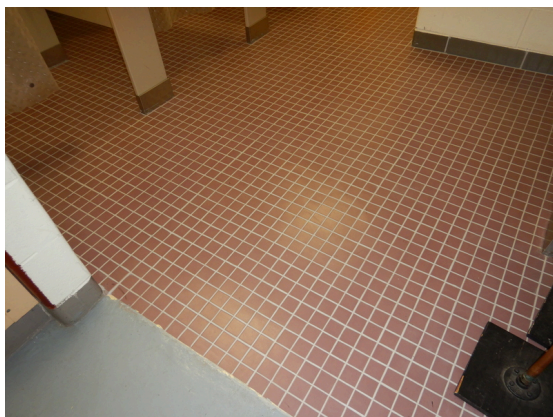
Photo 95: Locker room shower flooring.
