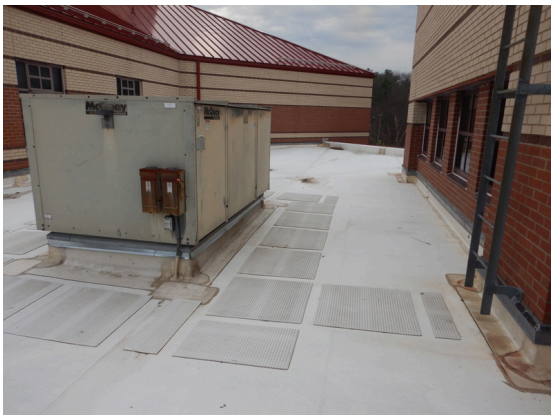
Photo 59: Gym: TPO membrane.
