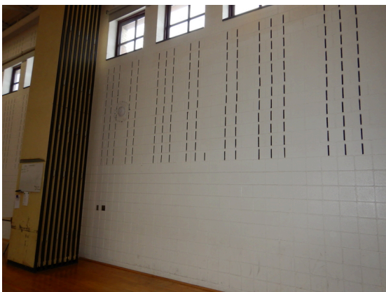
Photo 29: Gymnasium wall finish.
