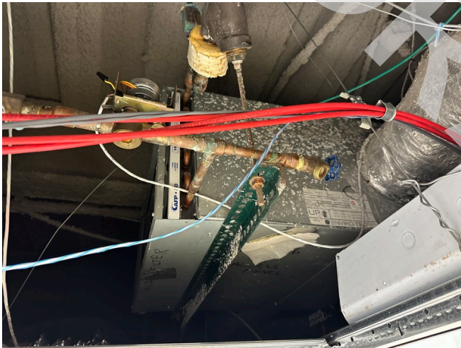
Typical VAV terminal units.
