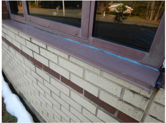
Brick veneer below windows.
