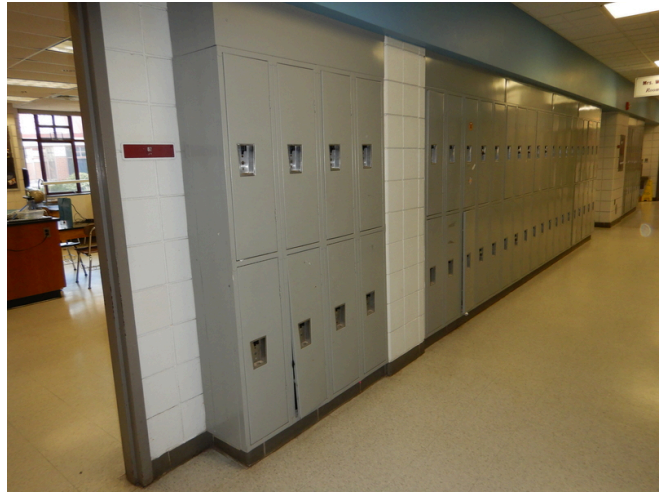
Typical corridor lockers.
