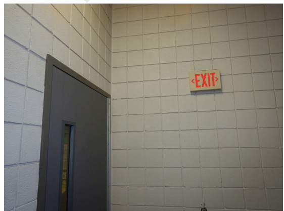
Photo 126: Painted CMU wall finishes.
