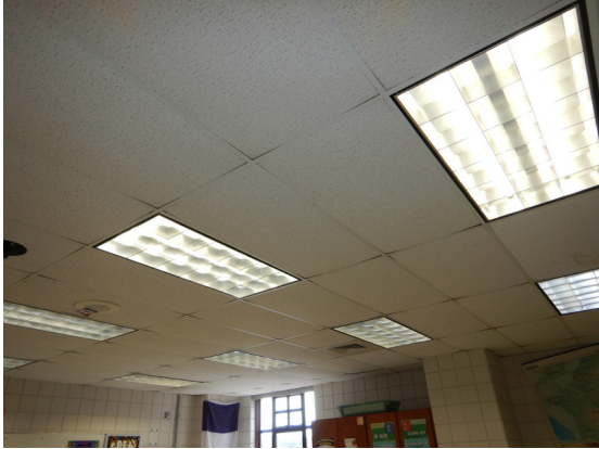
Photo 145: Classroom 81 ceiling finishes.
