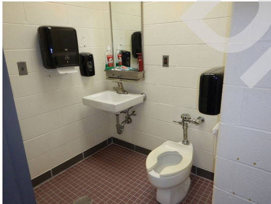
Photo 93: Girls locker room toilet and sink.
