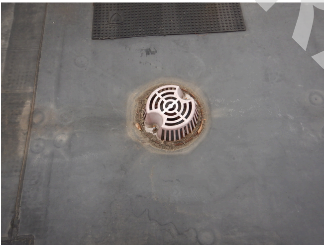
Internal drain.
