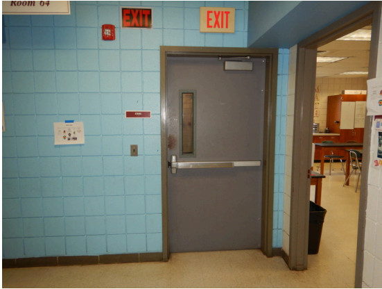
Photo 115: Emergency exit door leading to the egress stairway.
