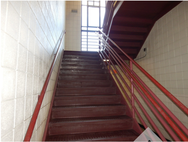
Typical egress stairway steps.
