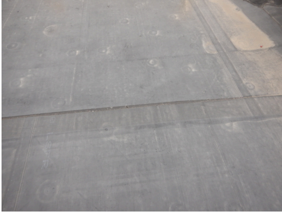
Photo 55: Close up of EPDM roof membrane.
