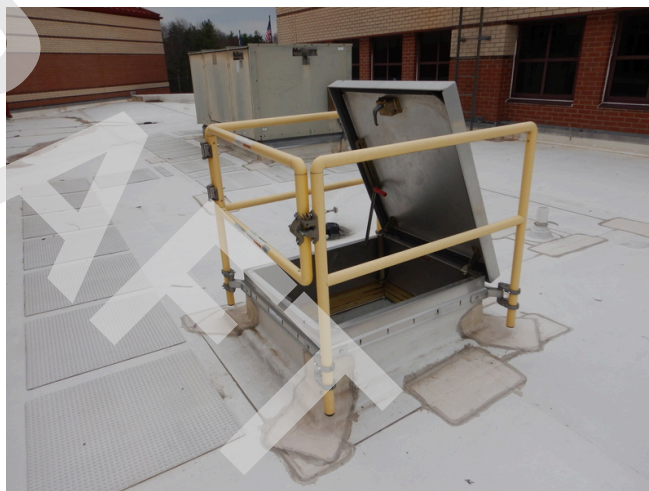
Gym: Roof hatch to the lower roof.
