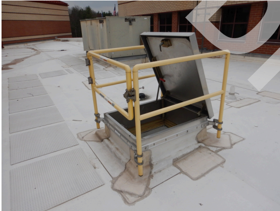
Photo 57: Gym: Roof hatch to the lower roof.
