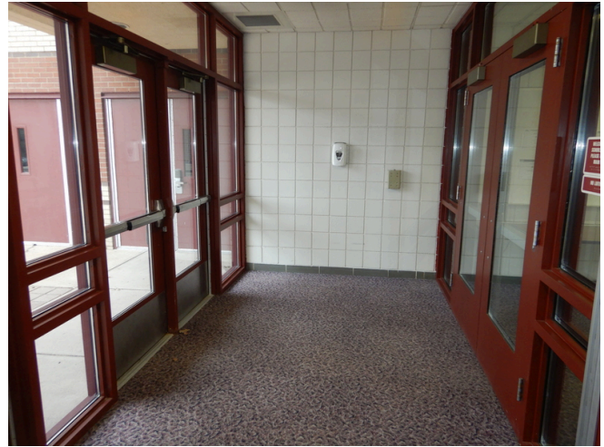
Accessible entrance doors in a series.
