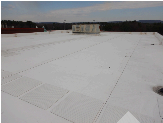
Gym: Roof overview facing northwest.
