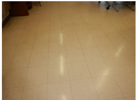
Photo 72: Dining room VCT flooring.
