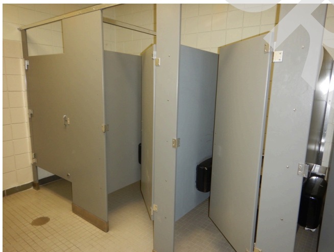
Typical 1st floor restroom toilet partitions.
