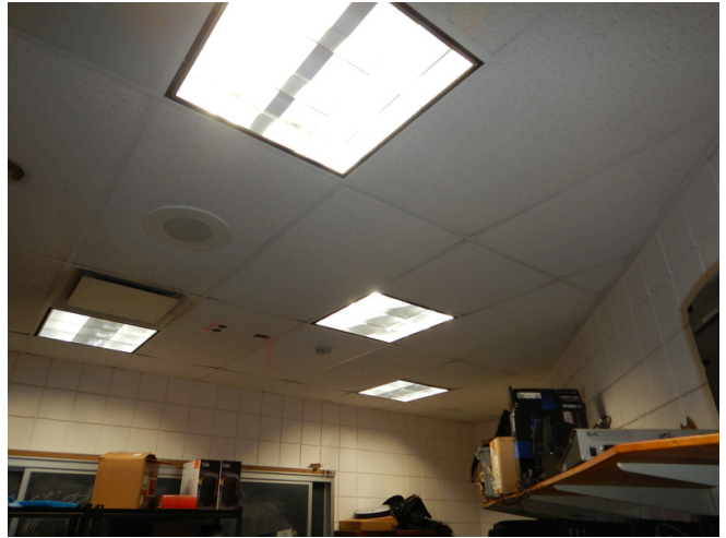
Technology Lab ceiling finish.
