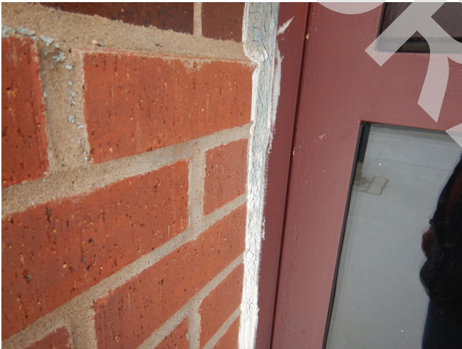
View of elastomeric sealant around the door.
