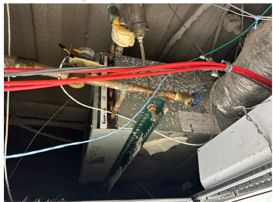
Photo 174: Typical VAV terminal units.
