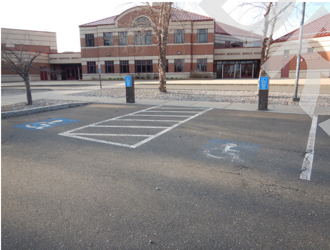
Accessible parking at the front elevation of the building.
