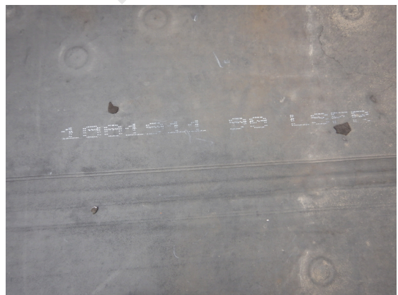
Photo 54: EPDM roof membrane.
