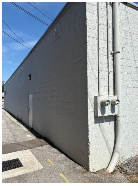
Prep and Repaint Exterior
