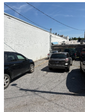
Prep and Repaint Exterior
