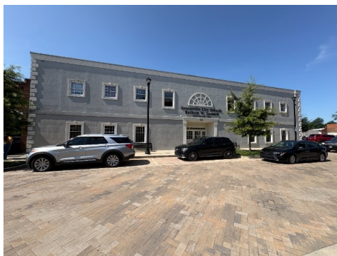
Prep and Repaint Exterior
