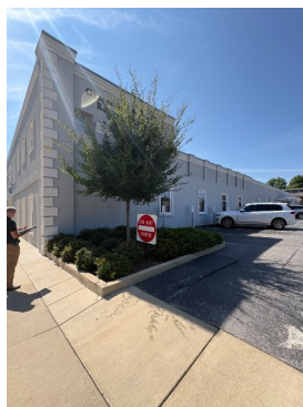
Prep and Repaint Exterior
