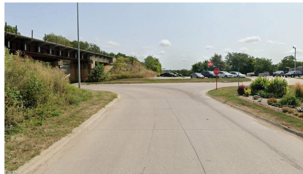
FIGURE 2.08 / NO SIDEWALKS, CROSSWALKS OR CURB RAMPS WHERE 1ST STREET MEETS HIGHWAY 6
