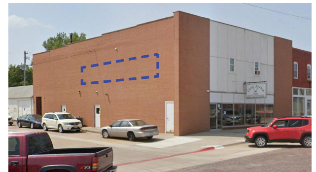
FIGURE 4.32 / POTENTIAL LOCATION FOR SIGNAGE AND LIGHTING ON EAST WALL OF PIZZA KITCHEN BUILDING
