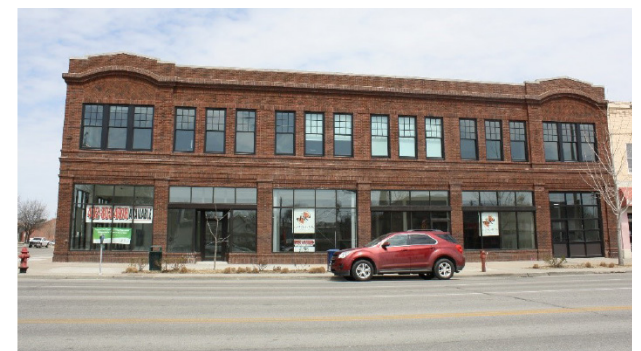
FIGURE 4.26 / AFTER WINDOW RESTORATION
