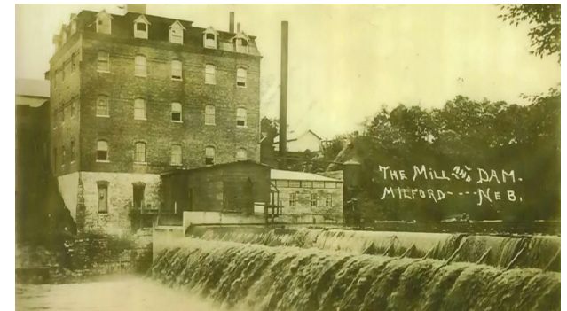
FIGURE 2.13 / HISTORICAL PHOTOGRAPH OF THE OLD MILL
