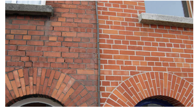
FIGURE 4.24 / BEFORE AND AFTER TUCKPOINTING MASONRY
