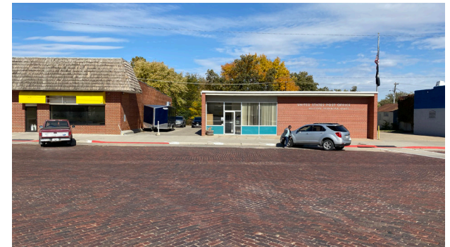
FIGURE 2.20 / POST OFFICE PARKING WITHIN THE INTERSECTION
