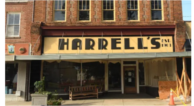
FIGURE 4.30 / BUILDING WITH SIGNAGE ABOVE A CANOPY
