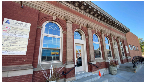
FIGURE 2.22 / OWNER OF ADVANCED ASSOCIATION MANAGEMENT RENOVATED THIS BUILDING WITH NEW WINDOWS
