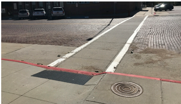
FIGURE 2.06 / PAINTED CONCRETE CROSSWALK WITH CURB RAMPS ON 1ST STREET AT B STREET
