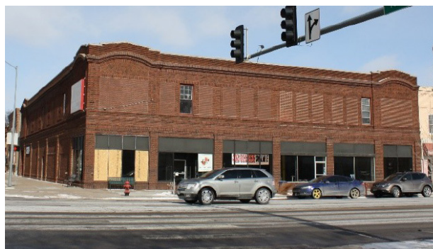
FIGURE 4.23 / BEFORE WINDOW RESTORATION
