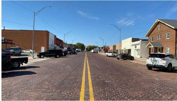
FIGURE 2.27 / BRICK SURFACING ON 1ST STREET DRIVE LANES
