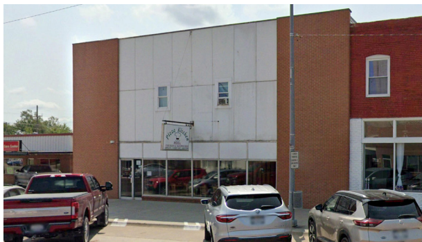
FIGURE 4.29 / EXISTING FACADE (PIZZA KITCHEN BUILDING)
