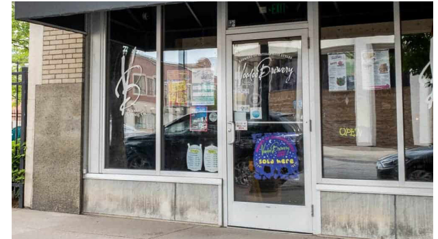
FIGURE 4.20 / COMMERCIAL DOOR ON COMMERCIAL BUILDING
