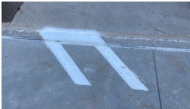
FIGURE 2.29 / PAINTED MARKINGS DESIGNATING EDGE OF ANGLED PARKING STALL ON 1ST STREET
