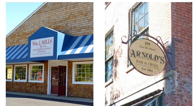
FIGURE 4.36 / AWNING SIGNS (LEFT) AND CAREFULLY DESIGNED PROJECTING SIGNS (RIGHT) ARE APPROPRIATE FOR DOWNTOWN USE
