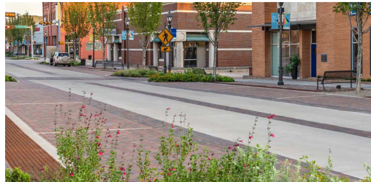
Brick at Intersections
