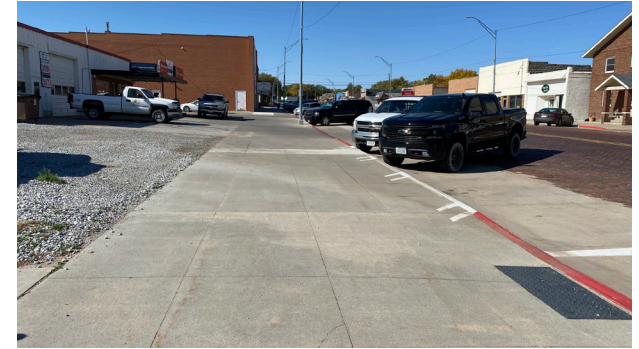
FIGURE 2.30 / CONCRETE SIDEWALK ON 1ST STREET LOOKING WEST
